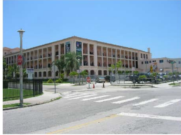
Shenandoah Middle School and Park are important destinations.
