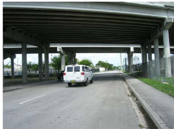
NW 11th Street could accommodate bicycle lanes.
