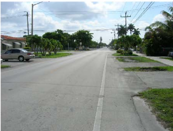
NW 14th Street is wide enough to accommodate a bicycle lane.
