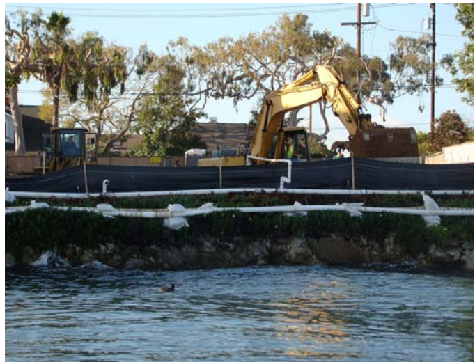
Figure 4.4. Construction in pipe trenches, Coronado. 02.17.11, 8:50am : ~6.7 feet above mean low tide.
