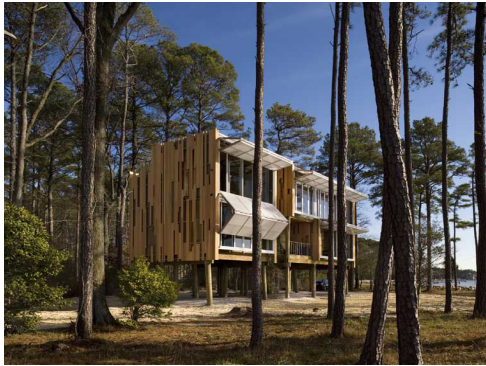
Loblolly House, Kieran Timberlake Architects
