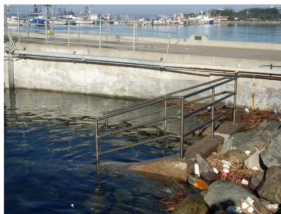
Figure 4.3. Flooded Storm Drain Outfall. 01.20.11, morning : ~7.2 feet above mean low tide.
