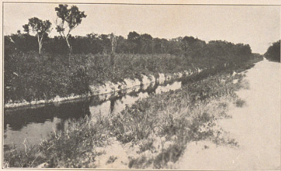
Shows how lands are drained. The white is coral rock, which when removed can make a boulevard in front of each lot.
