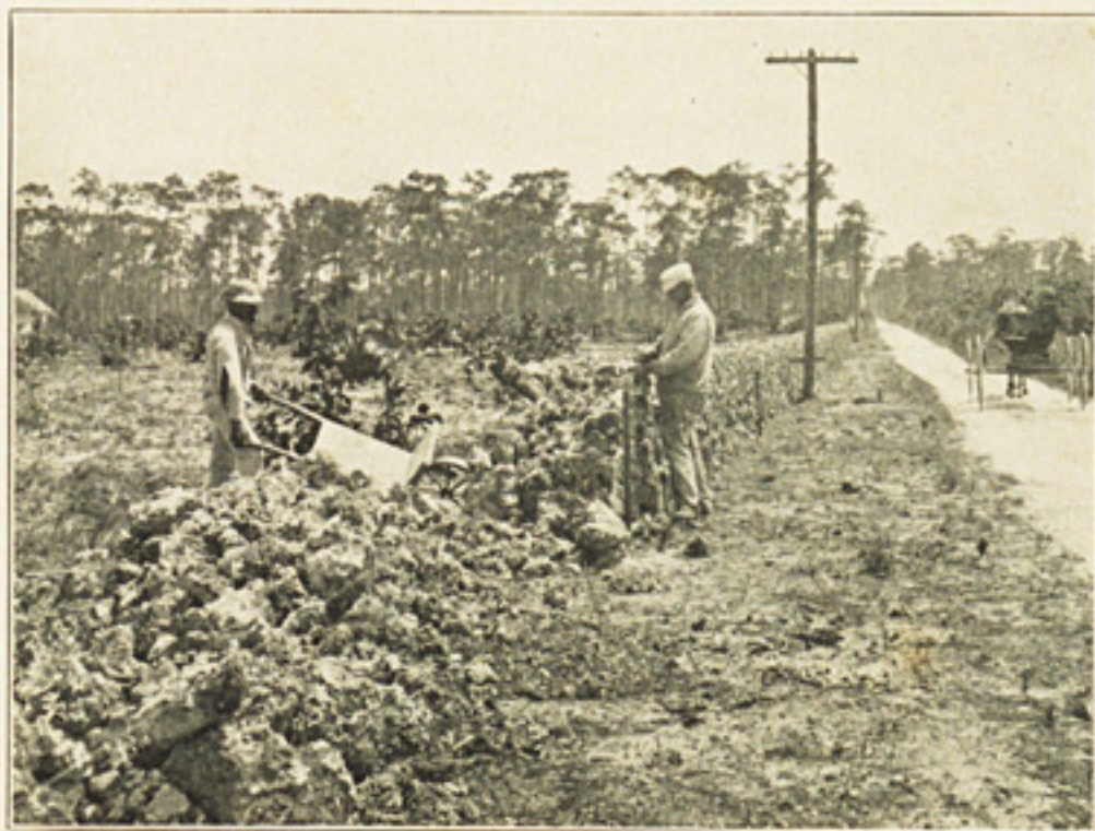
A SCENE IN THE PINE LAND ON THE MAINLAND. THE PINES ( P. CARIBAEA ) IN THE BACKGROUND. THE ROAD IS CONSTRUCTED OF LIME-ROCK, ALSO THE FENCE. THE ROCK WAS TORN FROM THE CLEARING ON THE LEFT BY GRUBBING AND BLASTING. (PHOTO BY PROF. JOHN CRAIG.)
