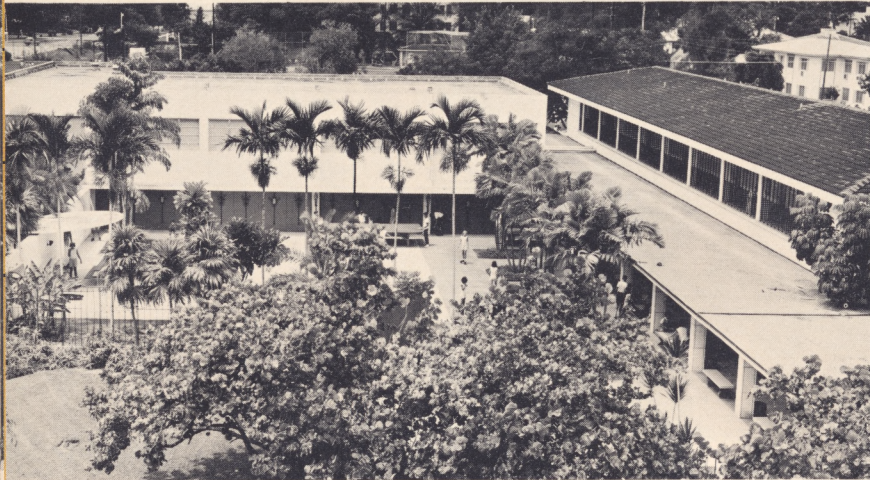
The Coral Gables Youth Center on Riviera Drive is an idealistic concept of a War Memorial
