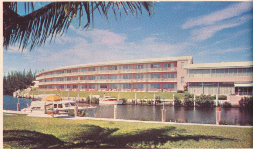
The University Inn on S. Dixie Highway is the gem of Coral Gables' own Motel Row, a composite of land and water landscaping that captures the essence of Coral Gables and extends along both sides of the beautiful waterway
