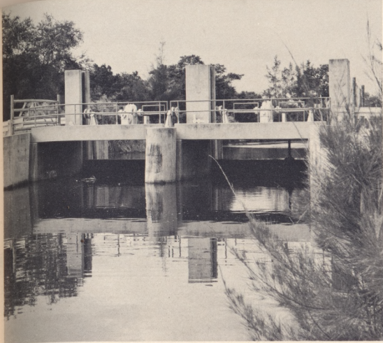
Salt intrusion dams help nature to help itself around the Miami area
