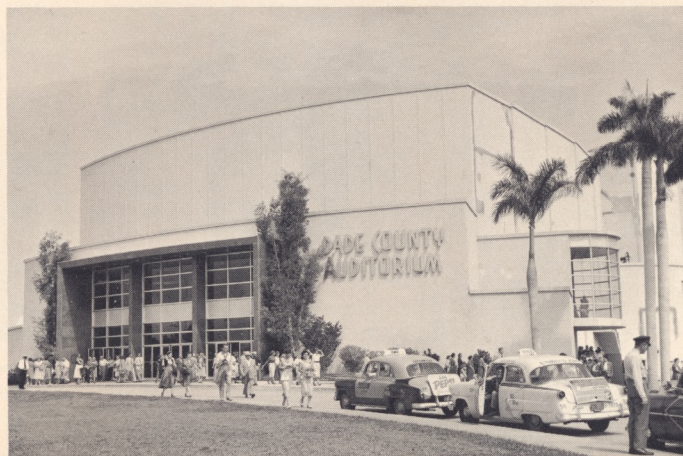
The County Auditorium on West Flagler Street at 28th Avenue accommodates the large conventions, musical productions, lectures and other civic activities
