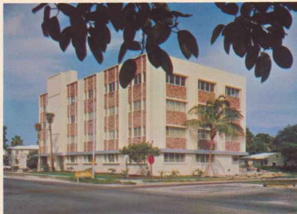
A Keyes-managed office building
