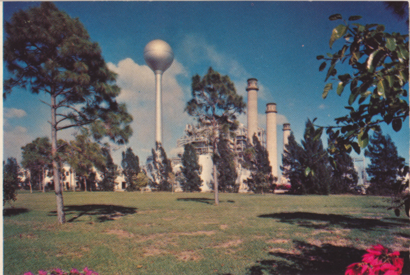
The tremendous expansion of Florida Power & Light plants is pacing the industrial growth of the area. Shown here is the Cutler plant
