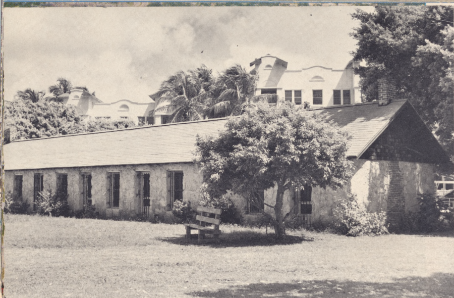
Old Fort Dallas originally stood in Dallas Park but was removed to Lummus Park at N.W. Third Avenue and Fourth Street
