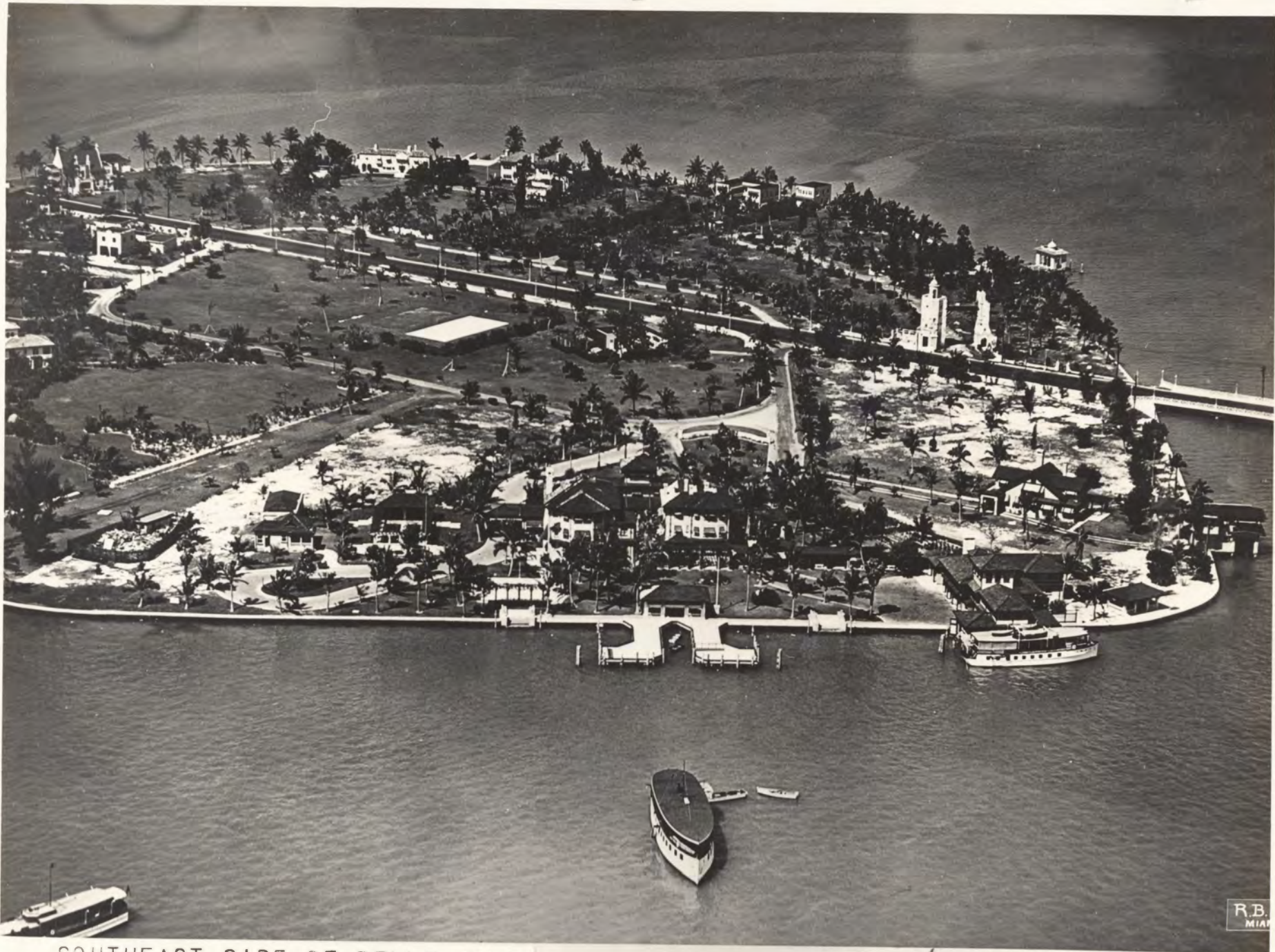
SOUTHEAST SIDE OF BELLE ISLE FEB. 1929
