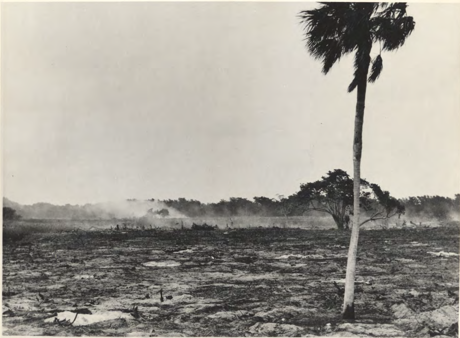
1-13. 1920—Clearing ground at Dade Boulevard and Prairie Avenue.
