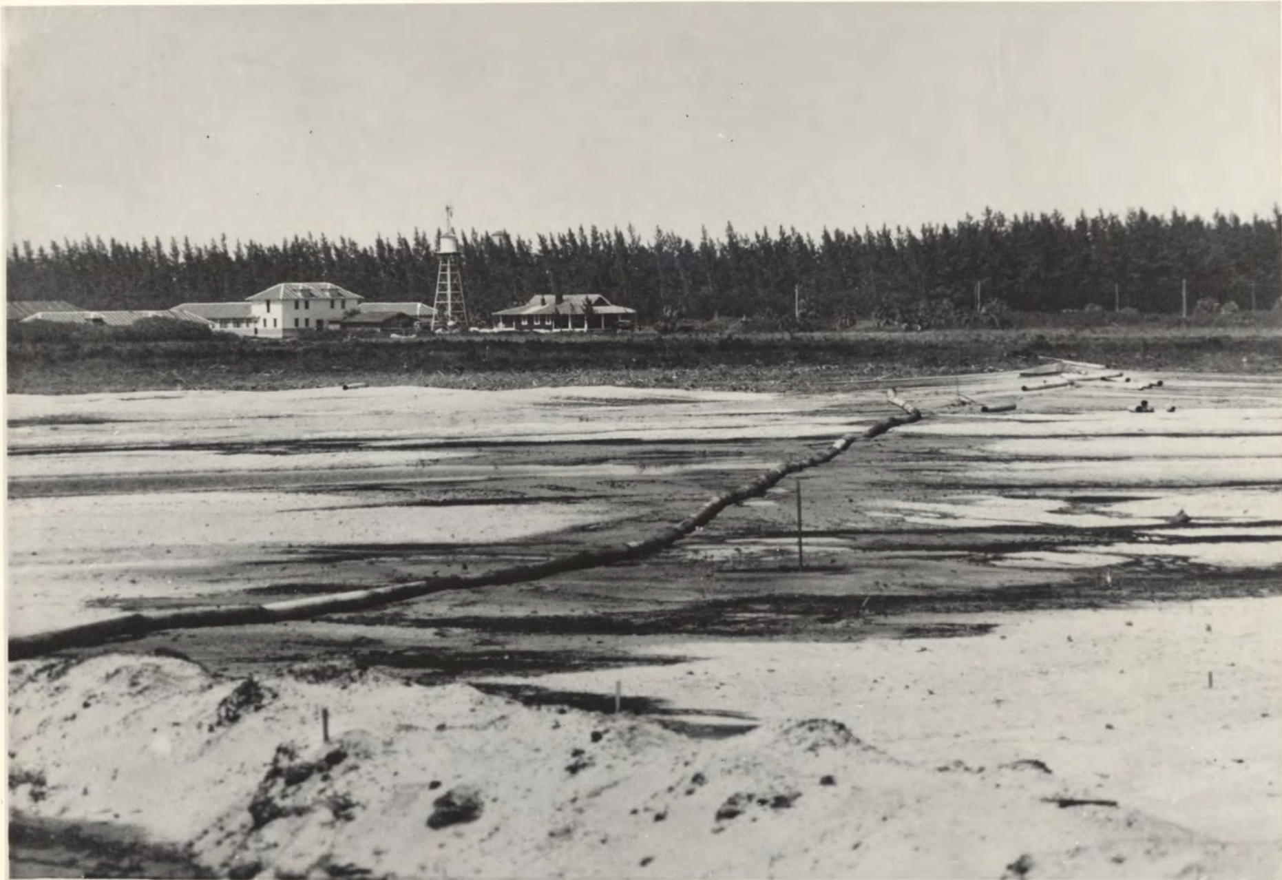
9-13. 1920—Dredge pipes in position for filling the low ground at Forty-first Street. The building shown in the picture is the Miami Beach Dairy, which was located on Forty-first Street near Chase Avenue.
