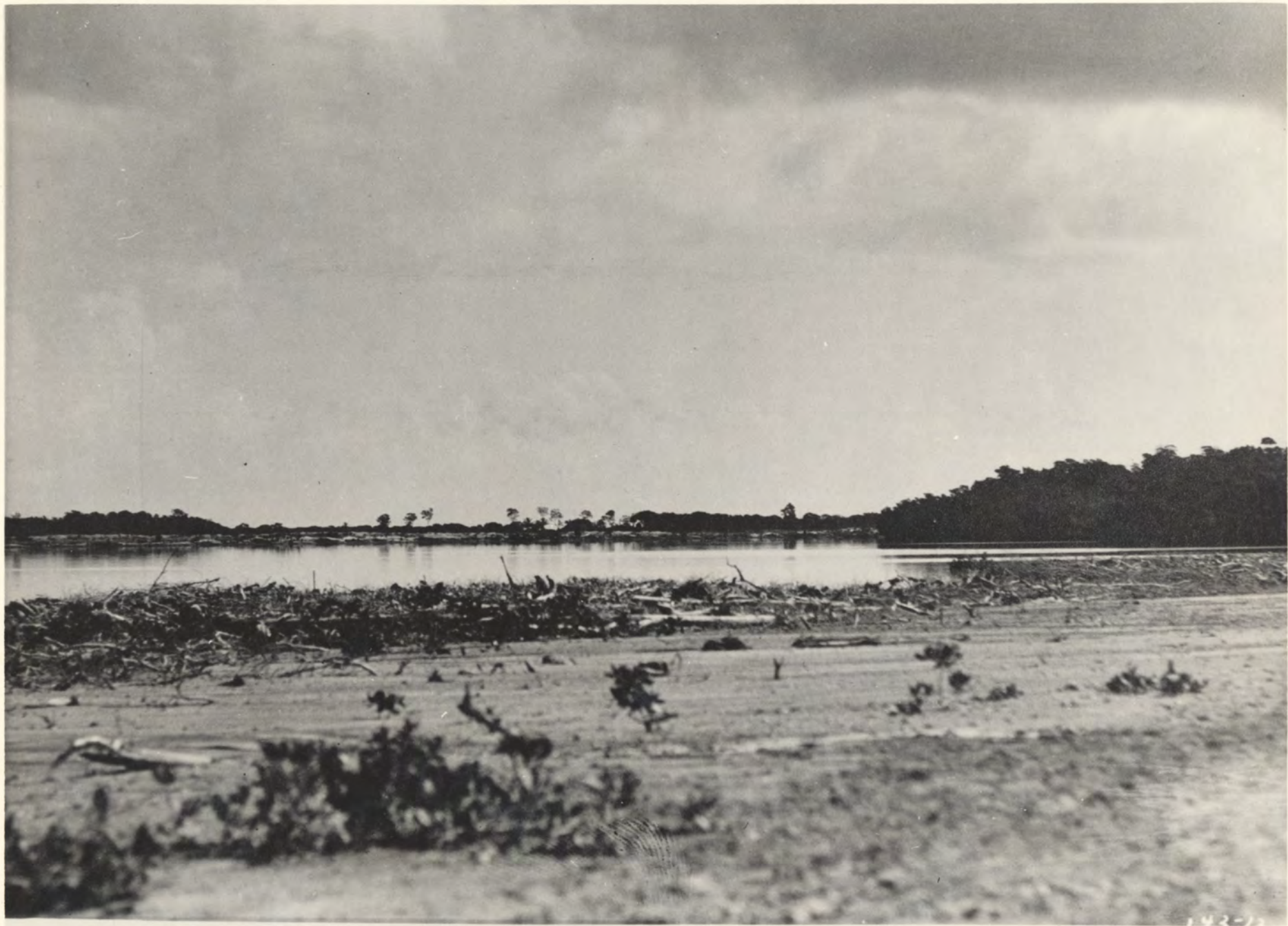
142-13. 1923—Nearly ready to fill, just north of the Nautilus Hotel site.
