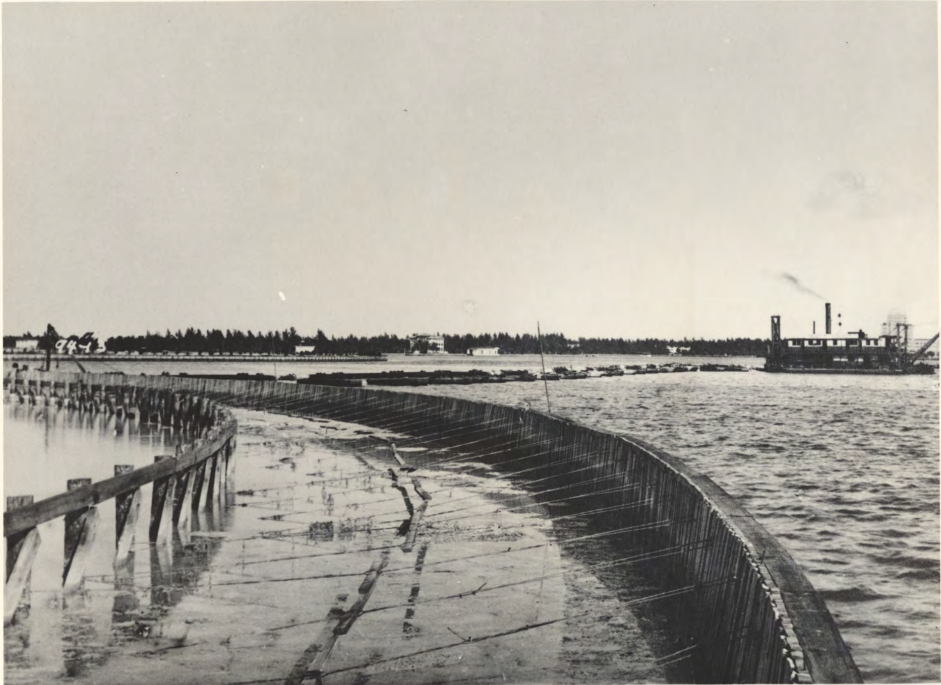
94-13. 1923—Bulkhead of a Venetian Island.
