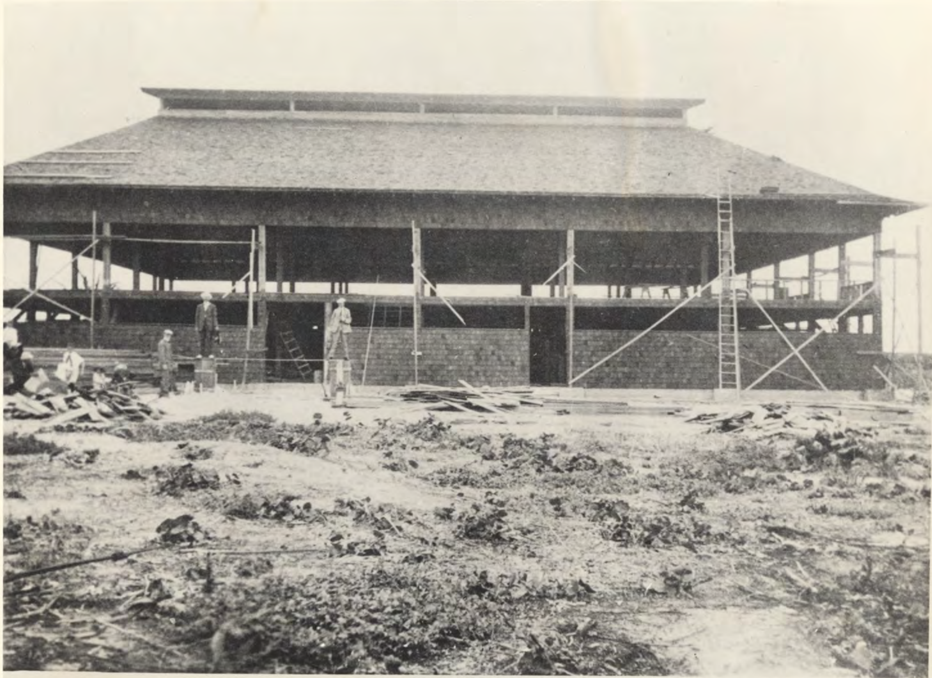
185-12 1913—Miami Beach Bathing Pavilion under construction. 23rd Street and Ocean.
