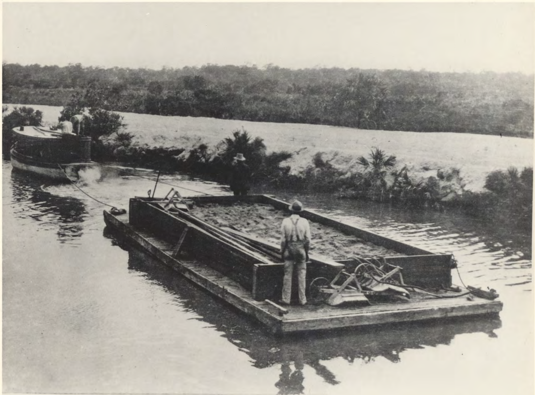
221-12. 1913—Collins Canal at Meridian Avenue.
