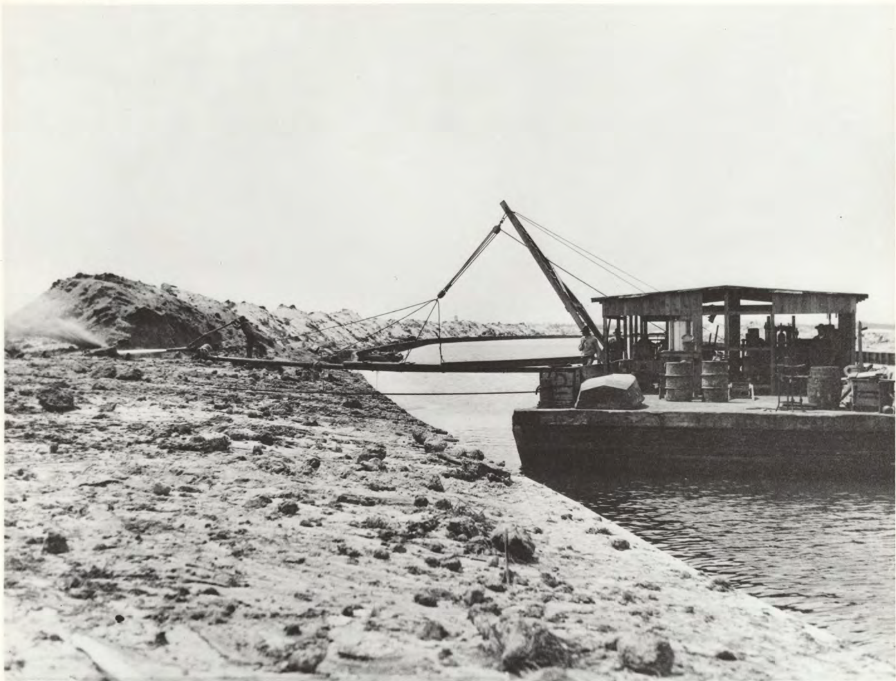
29-13. 1921—Filling and leveling back of sea wall.
