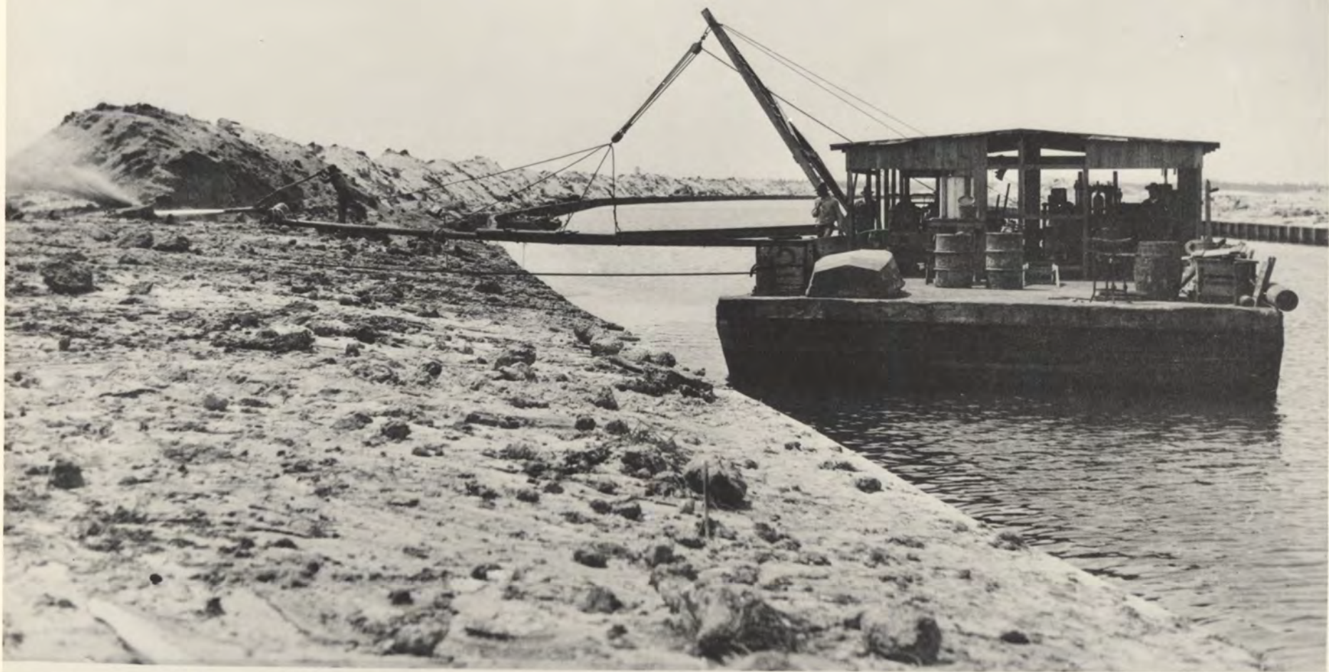
29-13. 1921—Filling and leveling back of sea wall.
