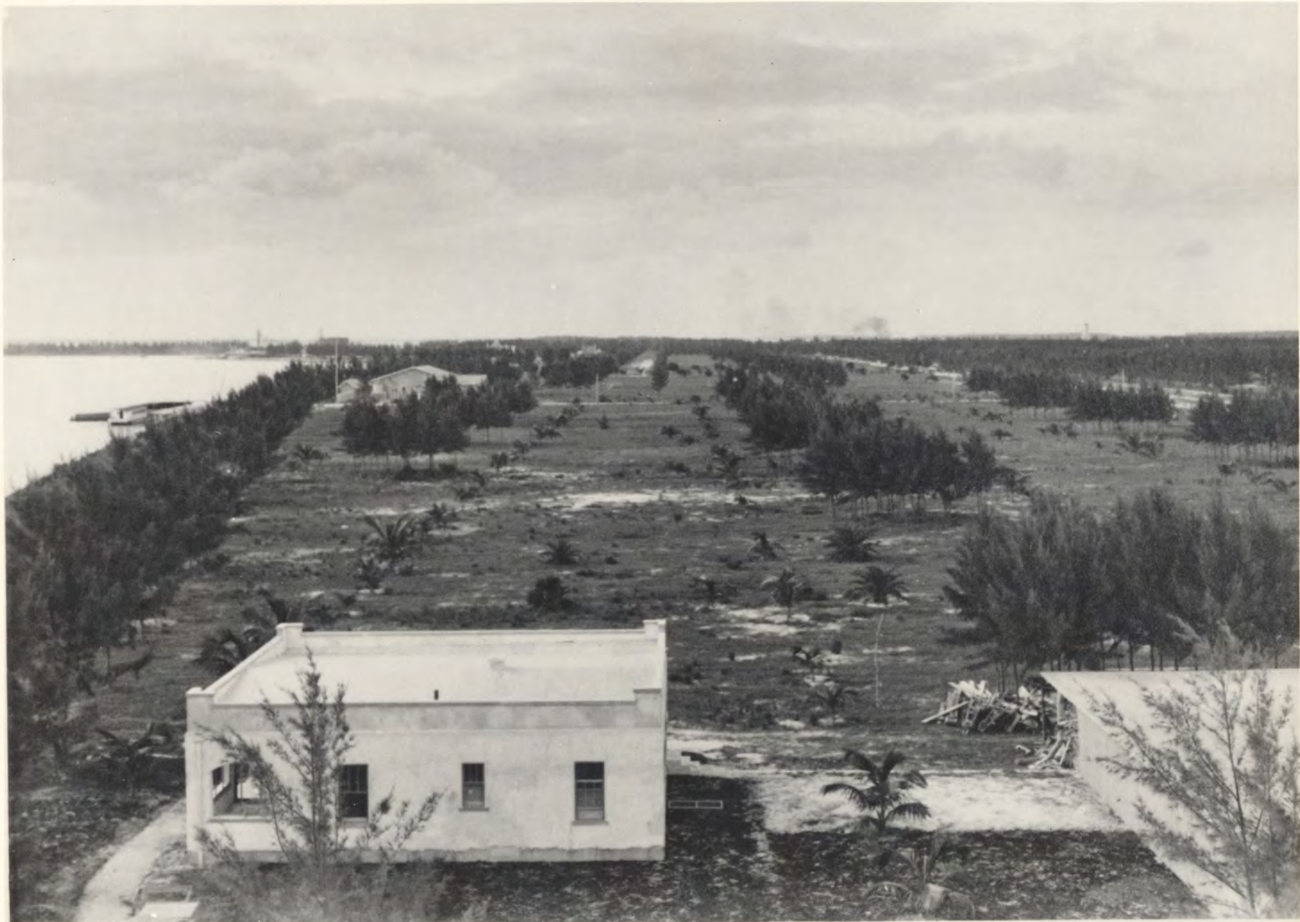
16 12. 1920— Bay side, looking north from the roof of the Allison Aquarium, which was located on Fifth Street at the bay.
