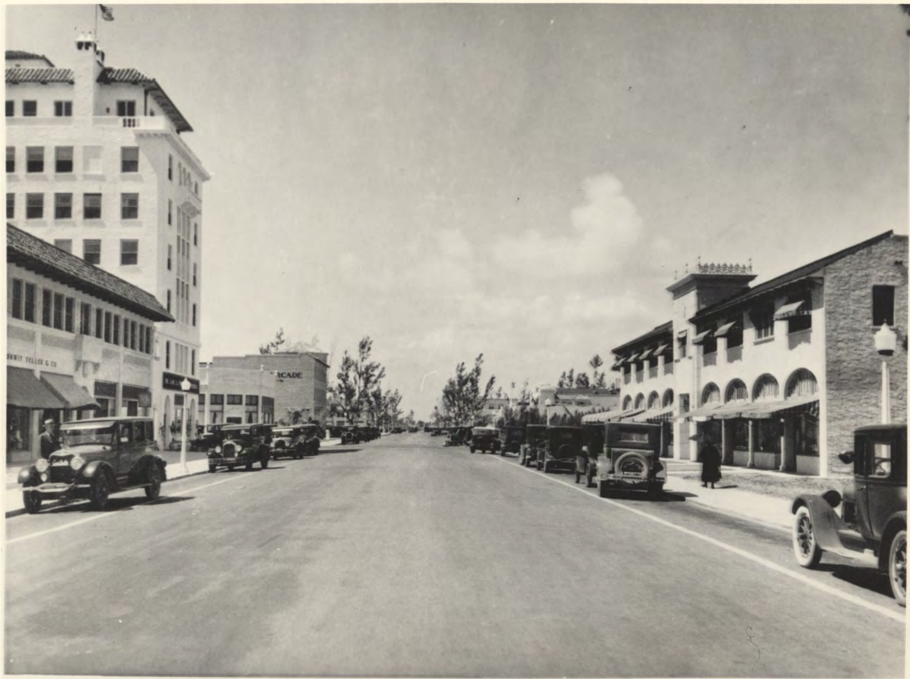
186-14. 1927—Lincoln Road, looking west.
