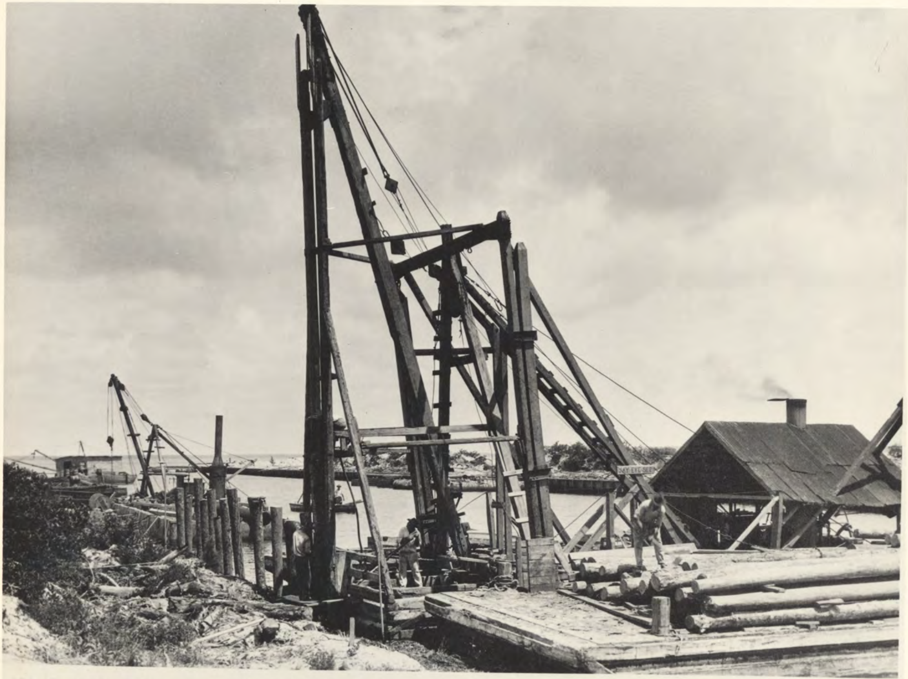
136-13. 1923—Building a sea-wall near the Nautilus Hotel site.
