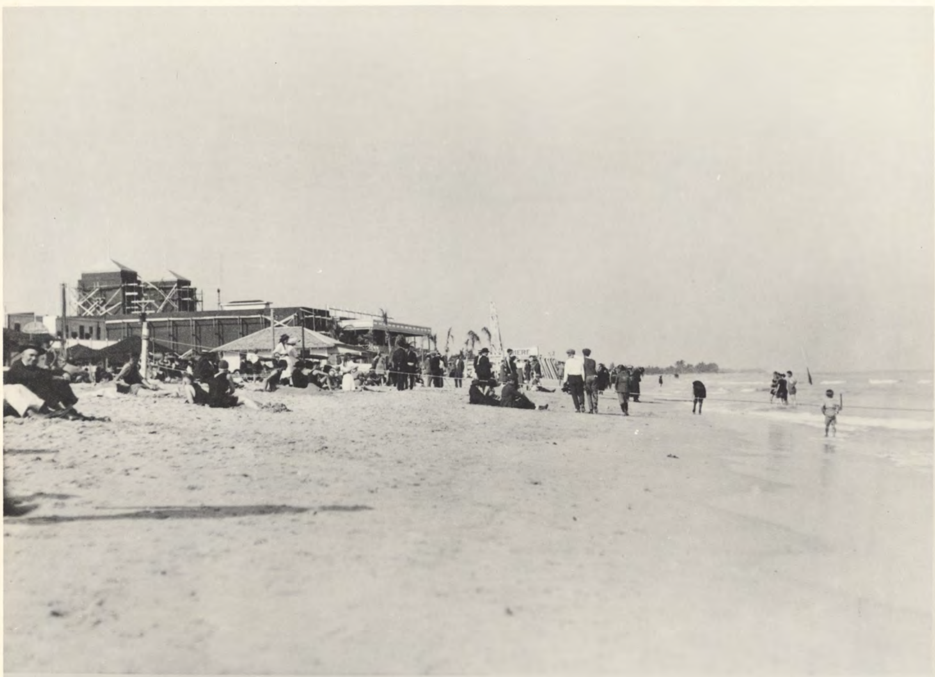
13-12. Christmas Day, 1919. Looking north, showing Hardie's Casino under construction.
