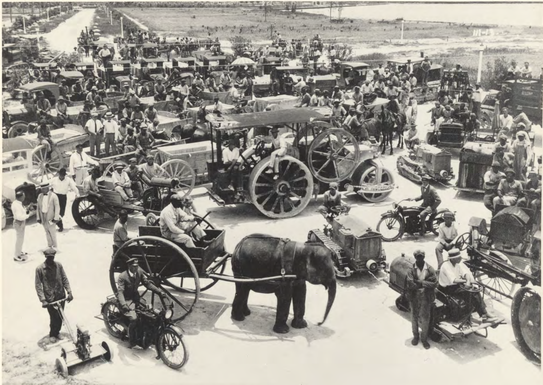
111-13. June 25, 1923—Alton Road at Forty-first Street, looking south. Equipment used in developing the North Bay Shore Section.
