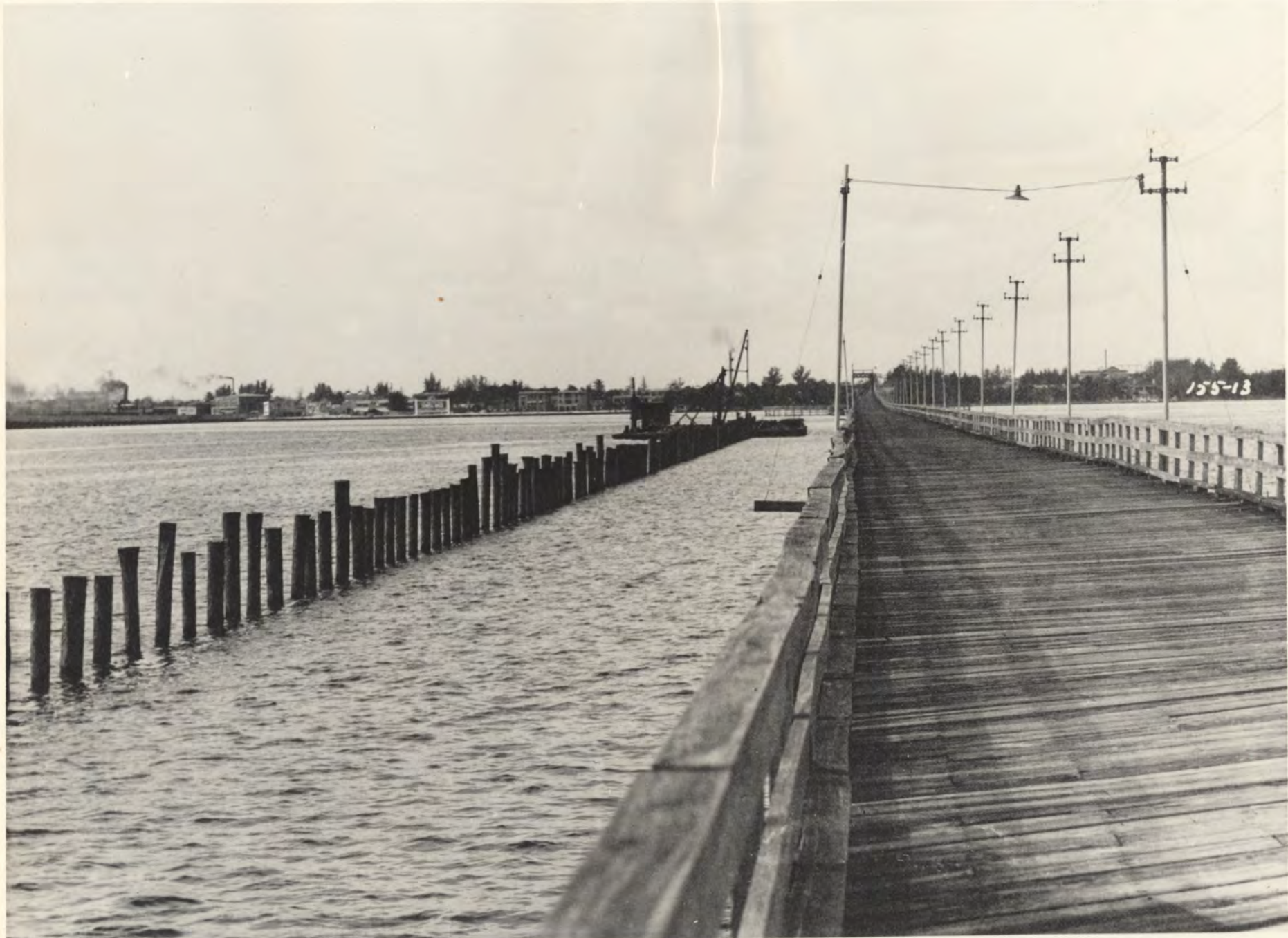
155-13. Dec. 24, 1923—The Collins Bridge, and the Venetian Islands under construction; looking toward Miami.
