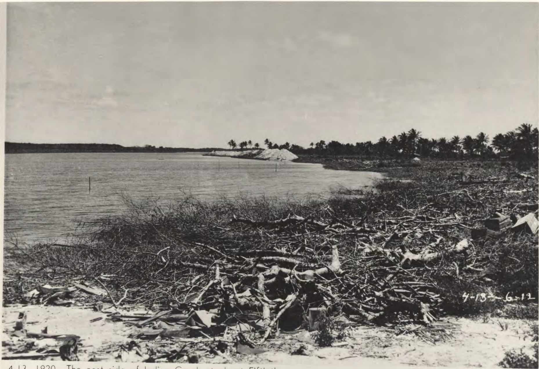
4-13. 1920—The east side of Indian Creek at about Fiftieth Street. In the immediate foreground a ballistic station was located during the World War. The picture shows the mangrove forest cut down, ready for the fill, and in the distance a part of the retaining fill.
