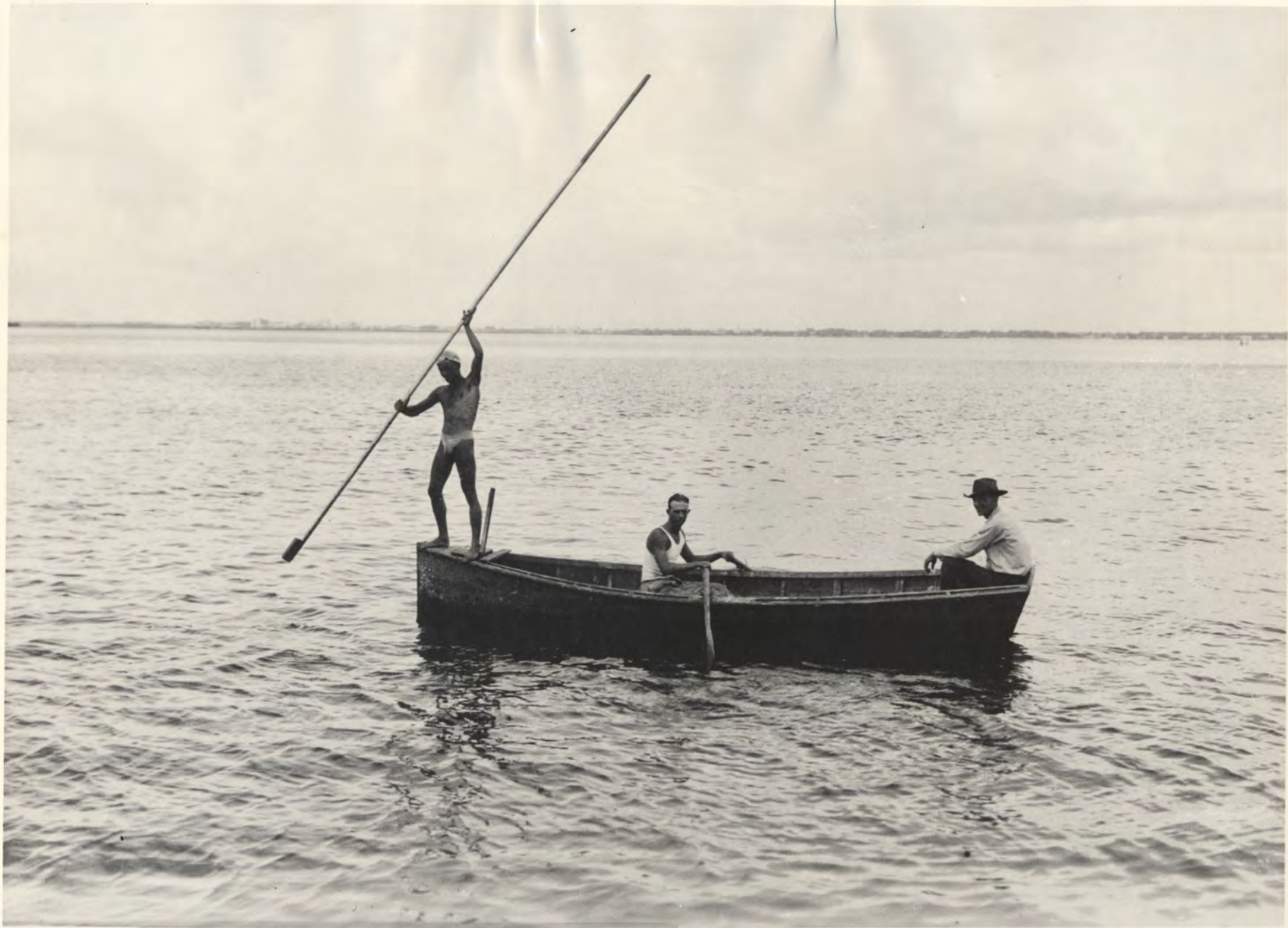
118-13. July 23, 1923—Engineers at work in the development of the North Bay Shore section.
