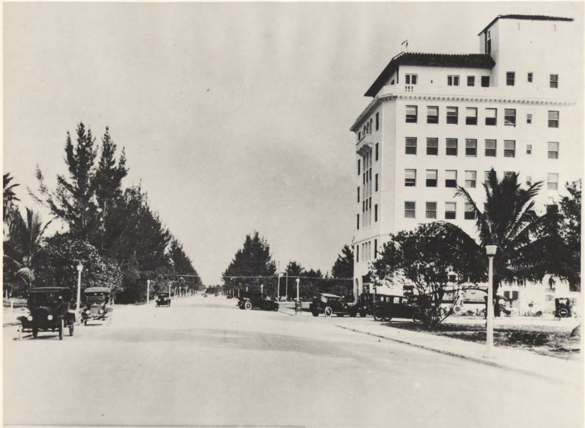
161-14 Nov. 30th, 1924—Fisher Building on Lincoln Road.
