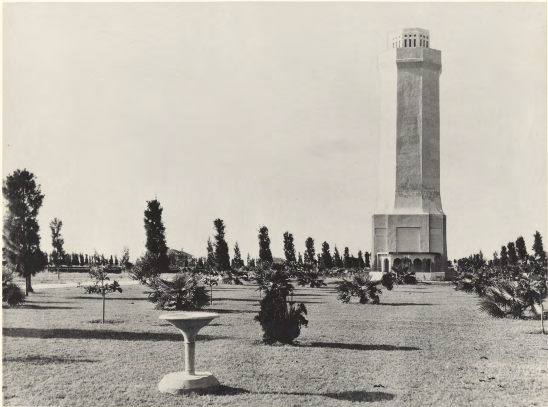
83-12. 1921—The water tower on Star Island.
