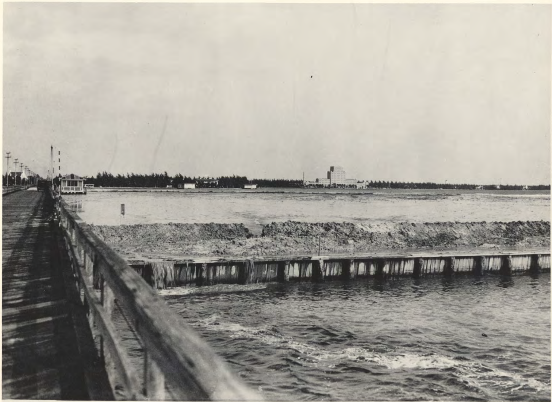
47-13. Nov. 1, 1923—The Venetian Islands under construction. Collins Bridge at the extreme left.
