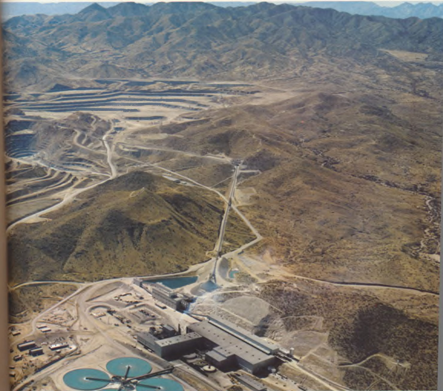
FOREGROUND: The world's largest copper and molybdenum concentrator at Duval Sierrita mine near Tucson, Arizona.
