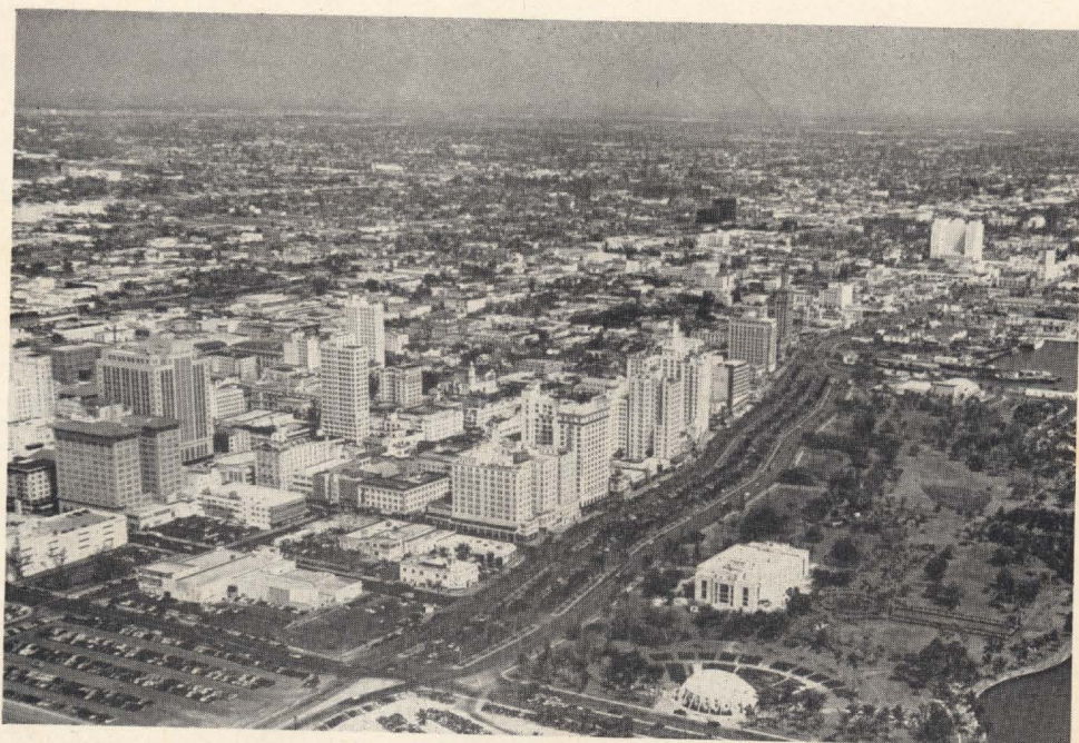
Downtown Miami, Bayfront Park in the foreground, famous Biscayne Boulevard, hotels and office buildings.
