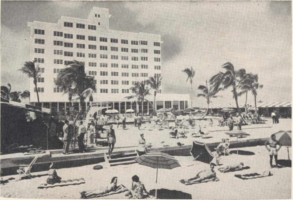
Kenilworth, Collins Avenue at 102nd Street, a Kirkeby Hotel
