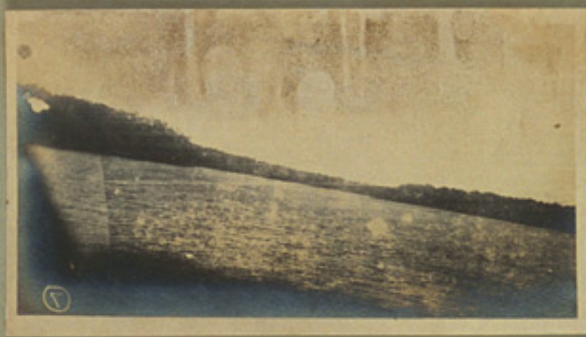
EXHIBIT 7. Photographic view of Chatham Bend River, showing magnitude of same, taken at a point immediately north east of Whitton Place.
