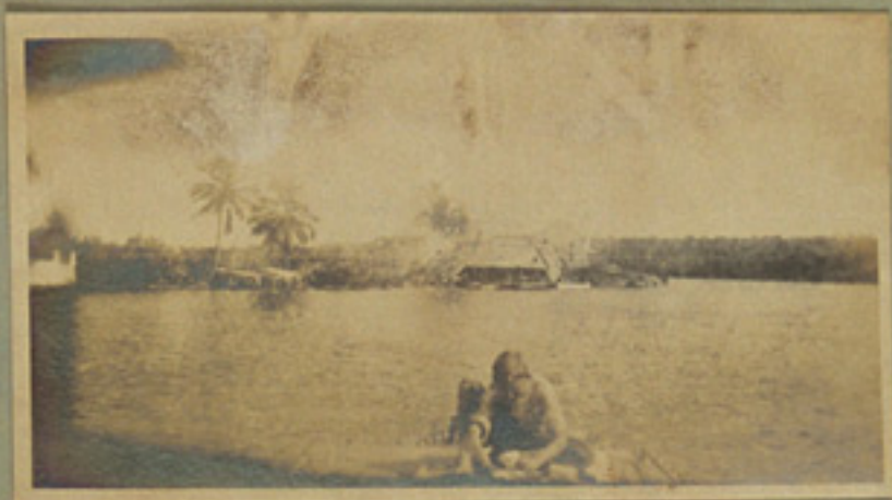
EXHIBIT 5. Photographic view of place occupied by D.H. Whitton, on north west shore of Chatham Bend River, formerly old Watson place, showing house, sugar mill, with sugar cane growing in back ground. Area of
