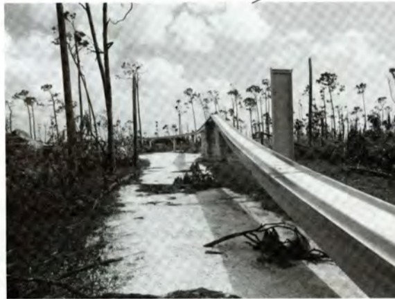
Monorail Track, Cars, Barn $2,450,000
