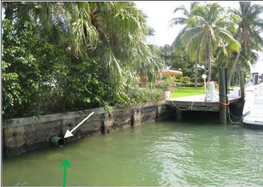
Tide Just Below Outfall
