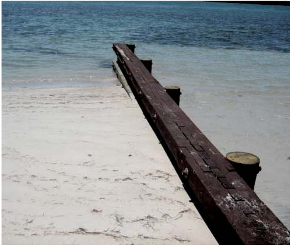
Photo 11: Timber groin, typ.
