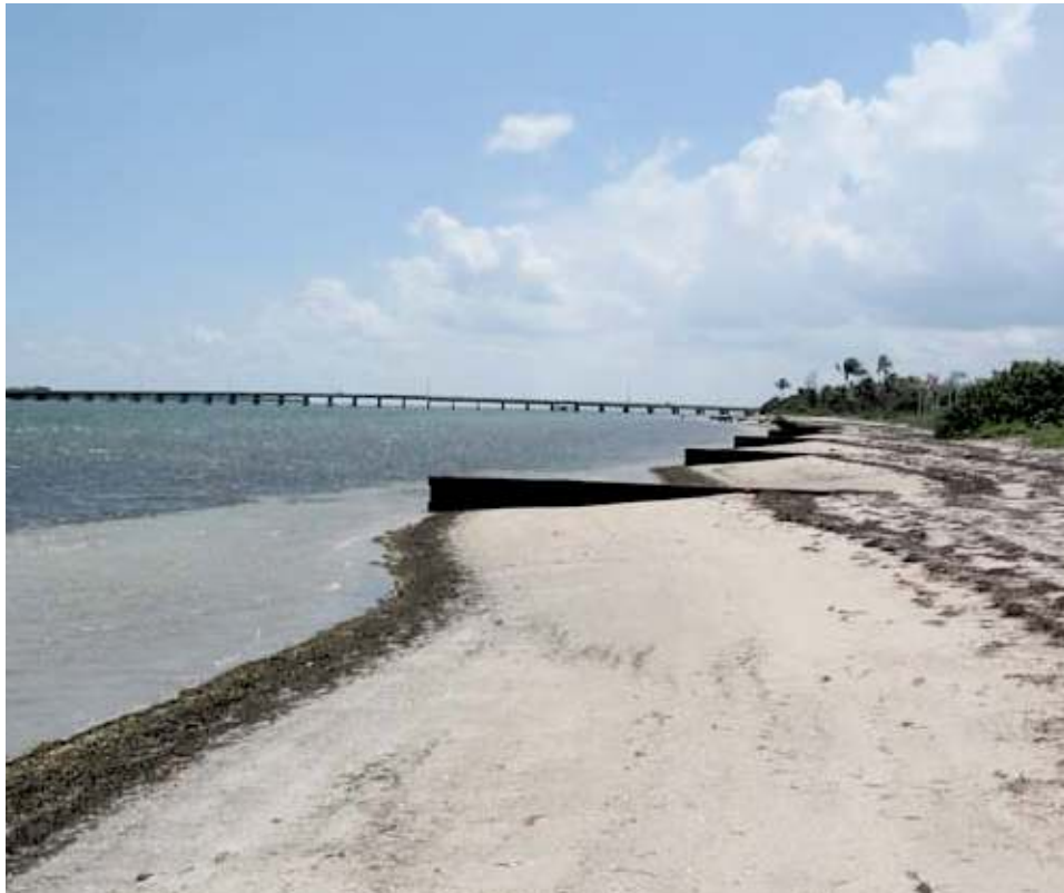
Photo 12: Southwest view along eastern segment of timber groin field.
