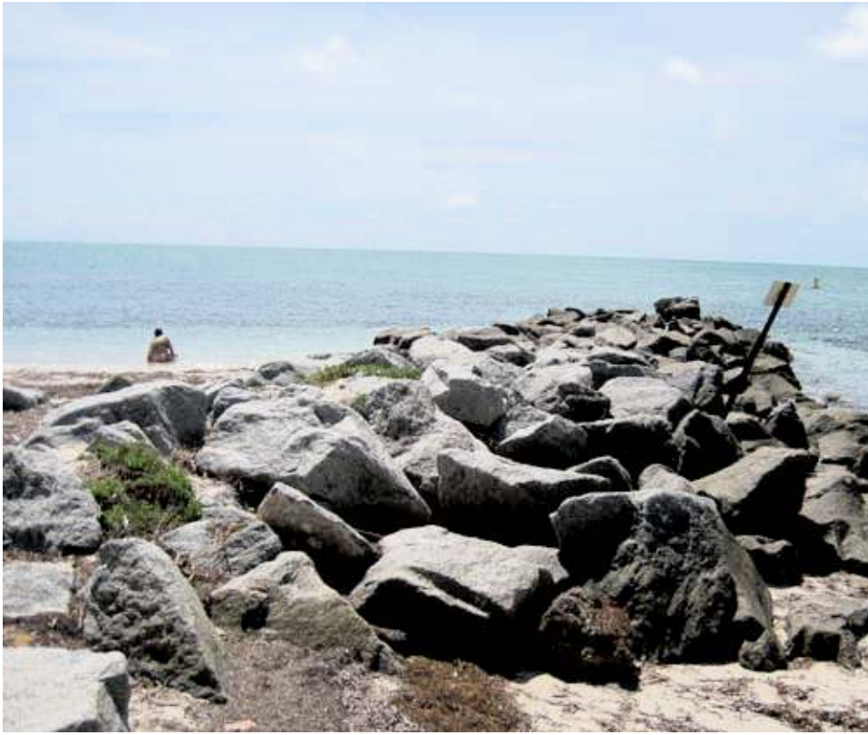
Photo 1: Rock groin, typ.
