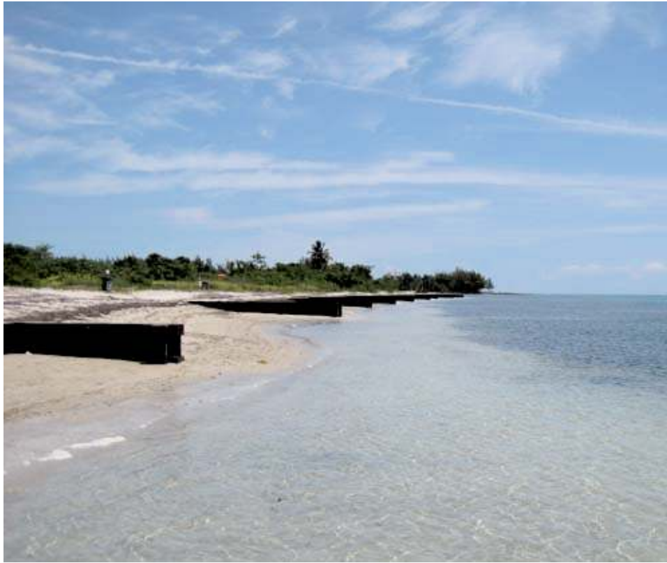
Photo 13: Northeast view along middle segment of timber groin field.
