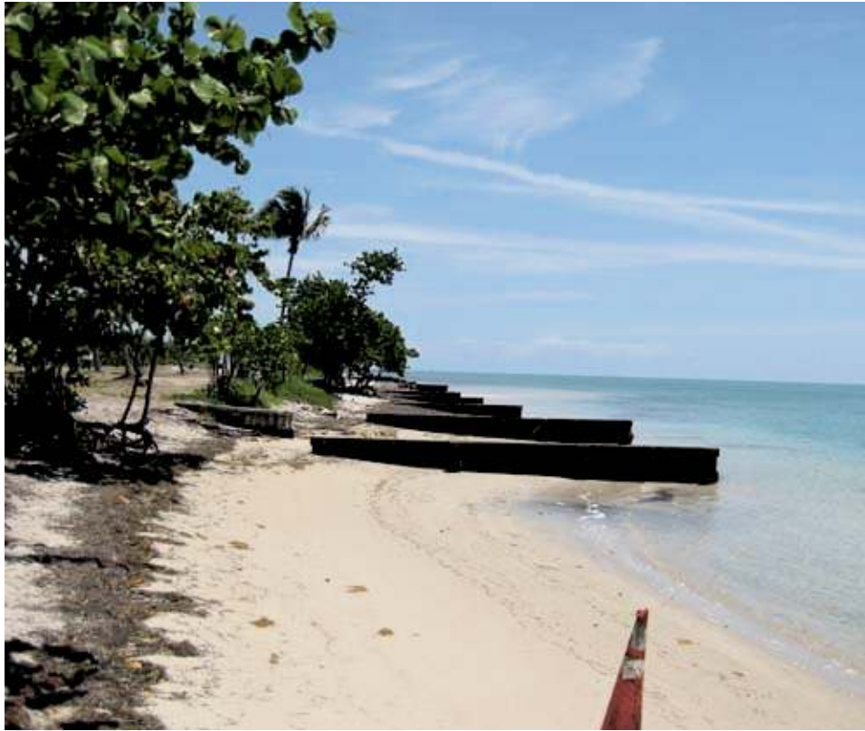
Photo 15: Northeast view along western segment of timber groin field.
