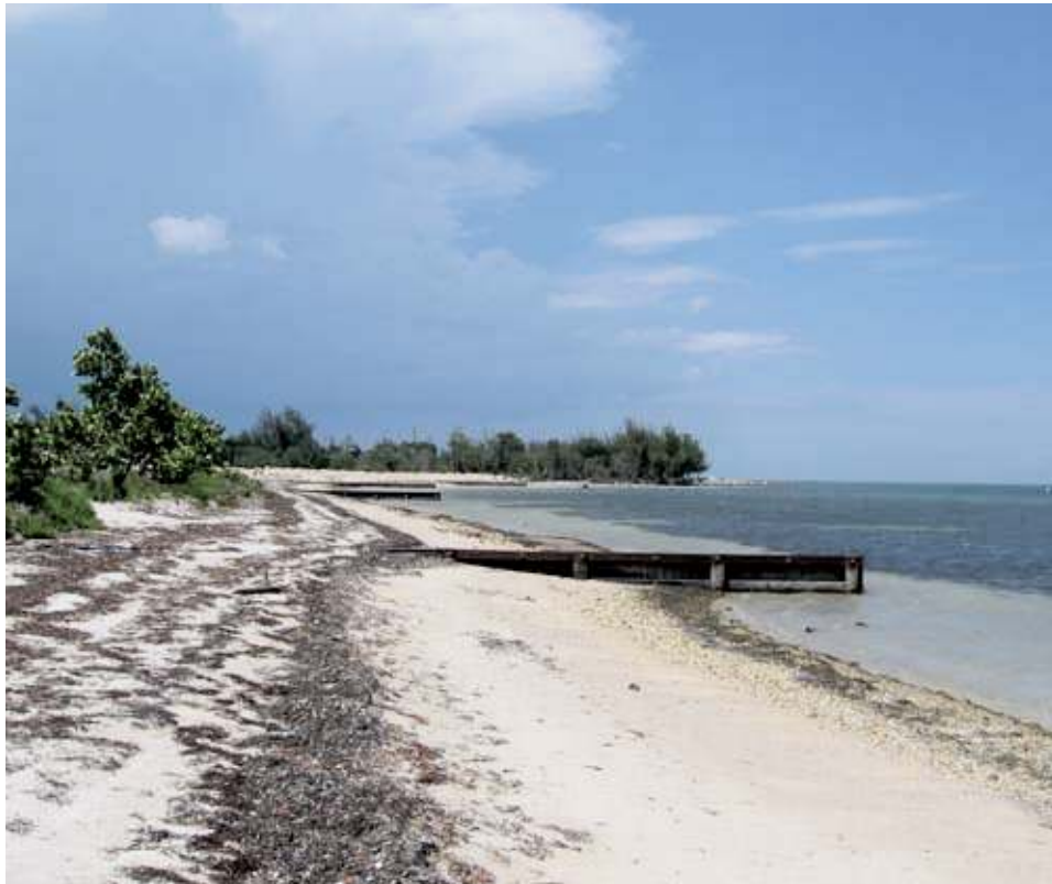
Photo 10: Northeast view along eastern segment of timber groin field.
