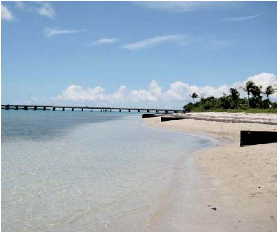
Photo 14: Southwest view along middle segment of timber groin field.
