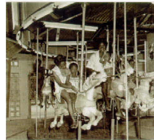
Carousel interior has been lost
