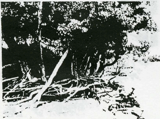
Eroded shoreline will be stabilized and revegetated
