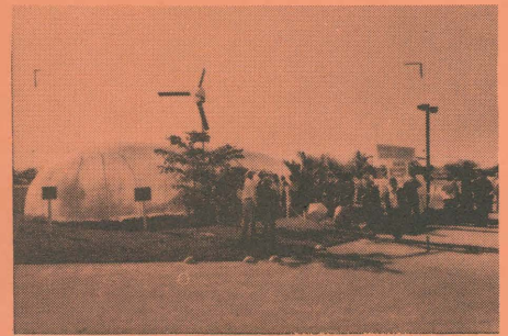
Above, 60-ft. long and 12-foot high, the structure was inflated in twelve minutes.
