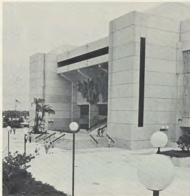
Main entrance of Primera Casa
