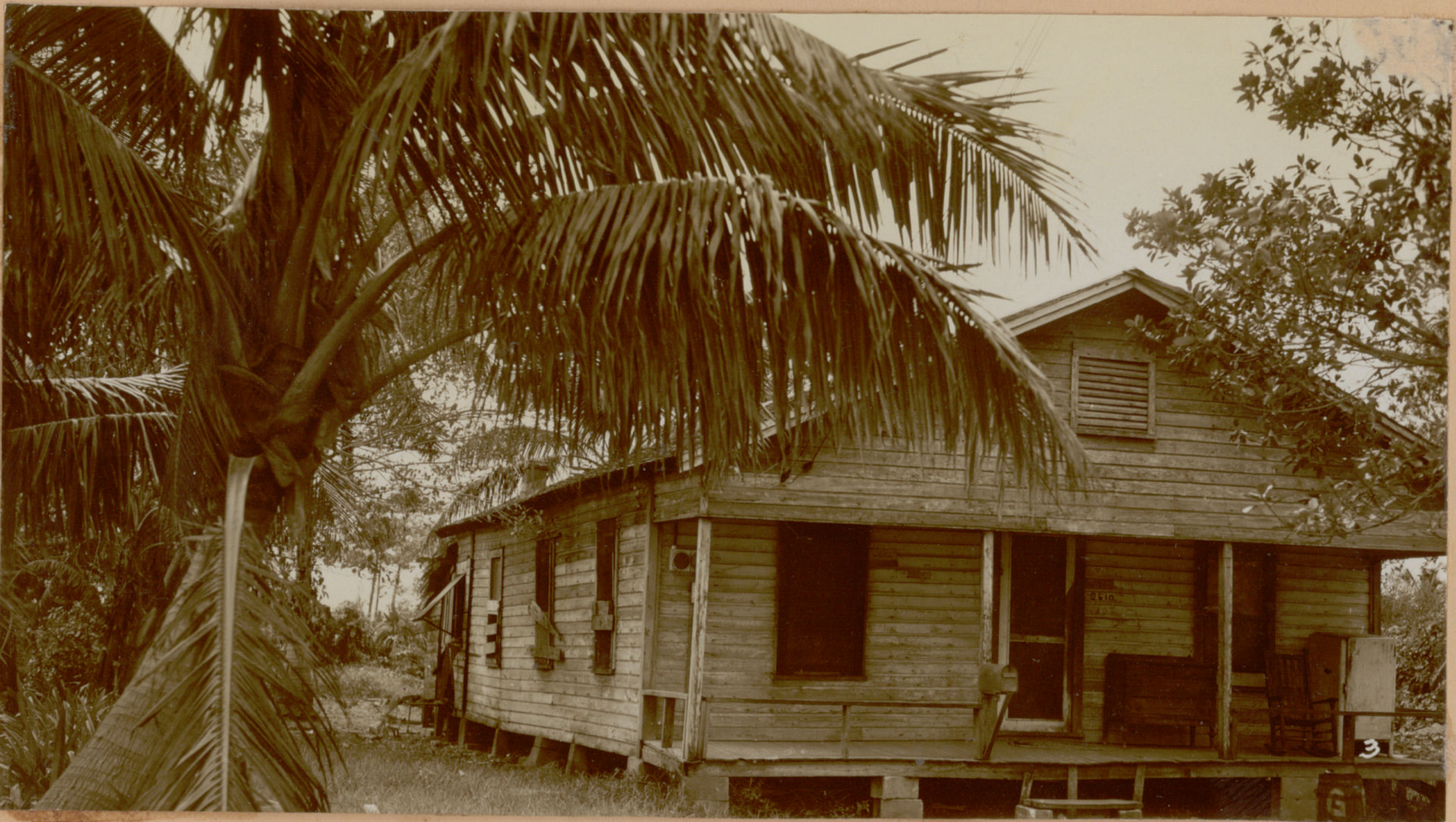
Looking Southwest at Building #2
