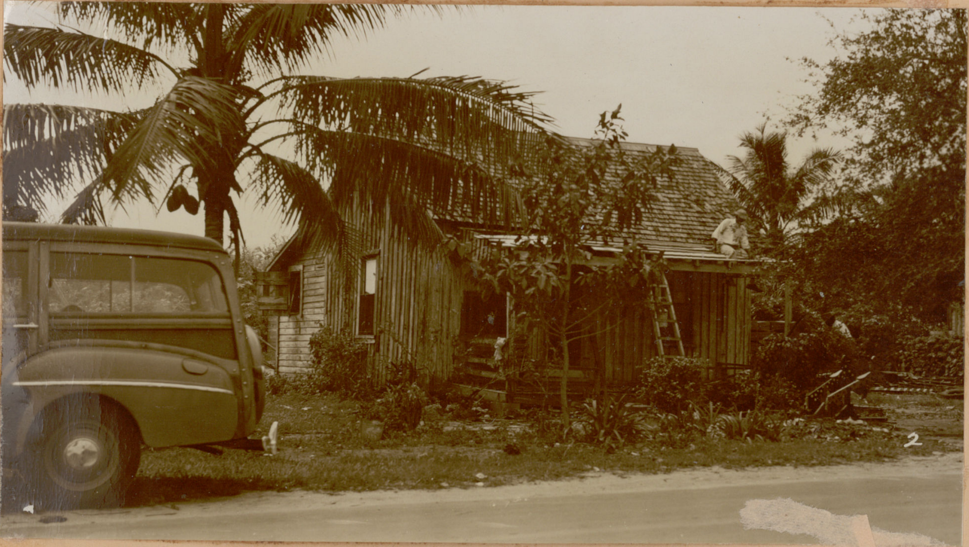
Looking Southwest at Building #1
