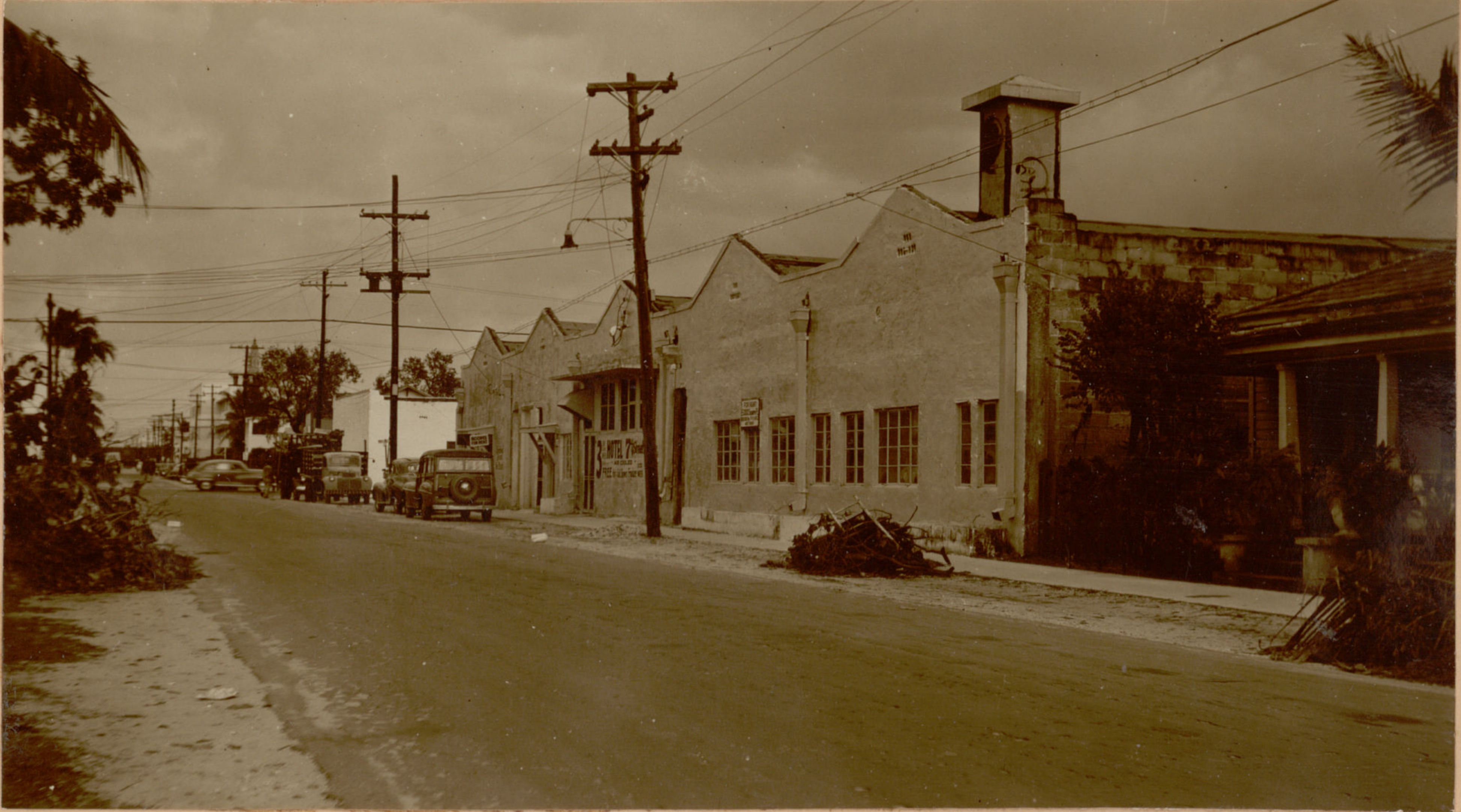
Looking Northeast at South (rear) elevation of converted warehouses
