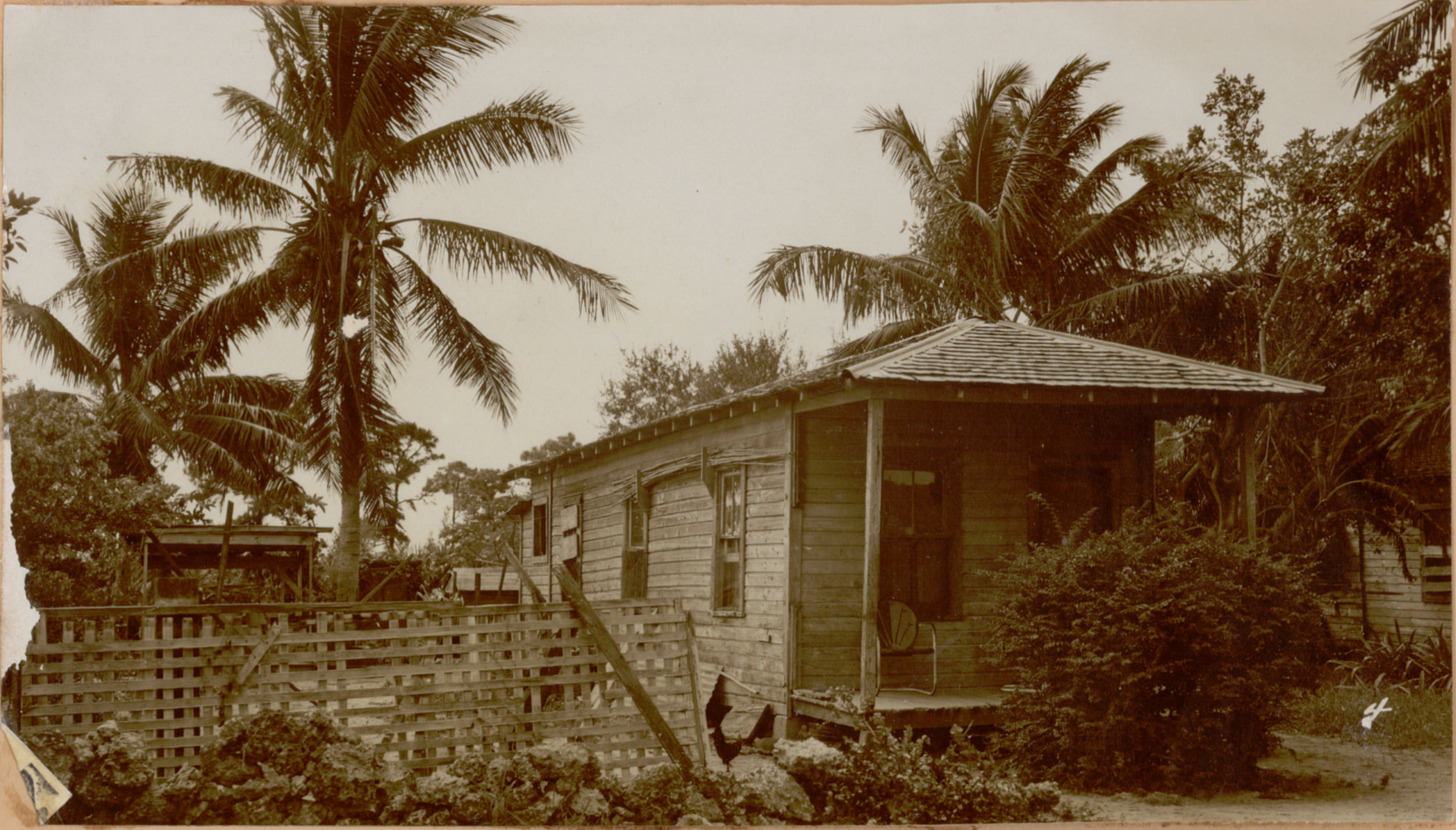
Looking Southwest at Building #3
