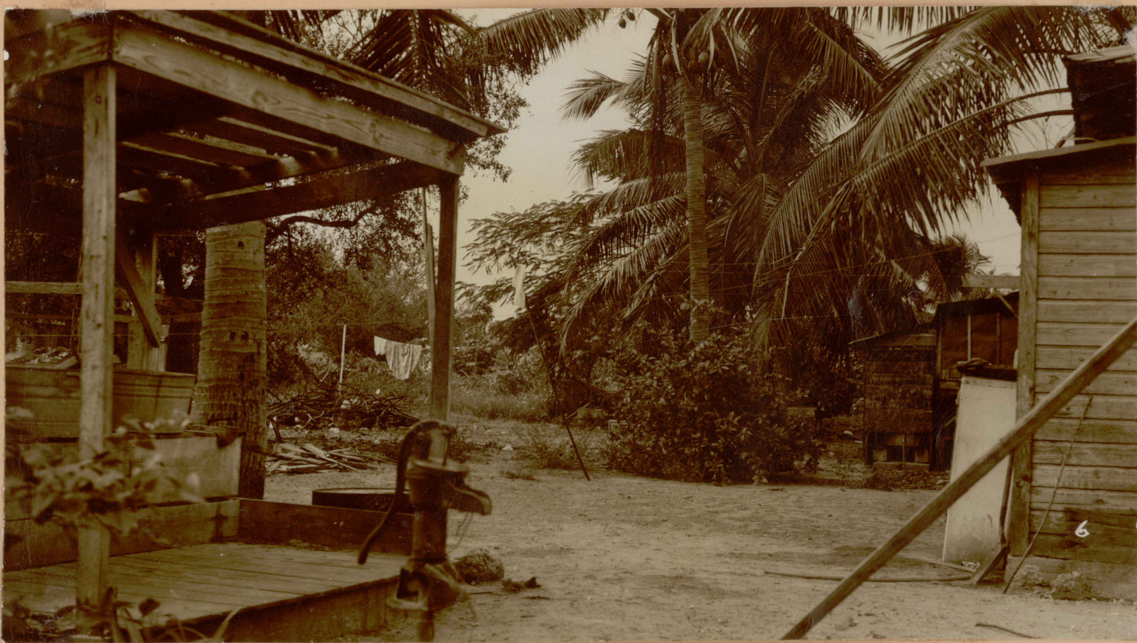
Looking Southwest from backyard of Building #4
