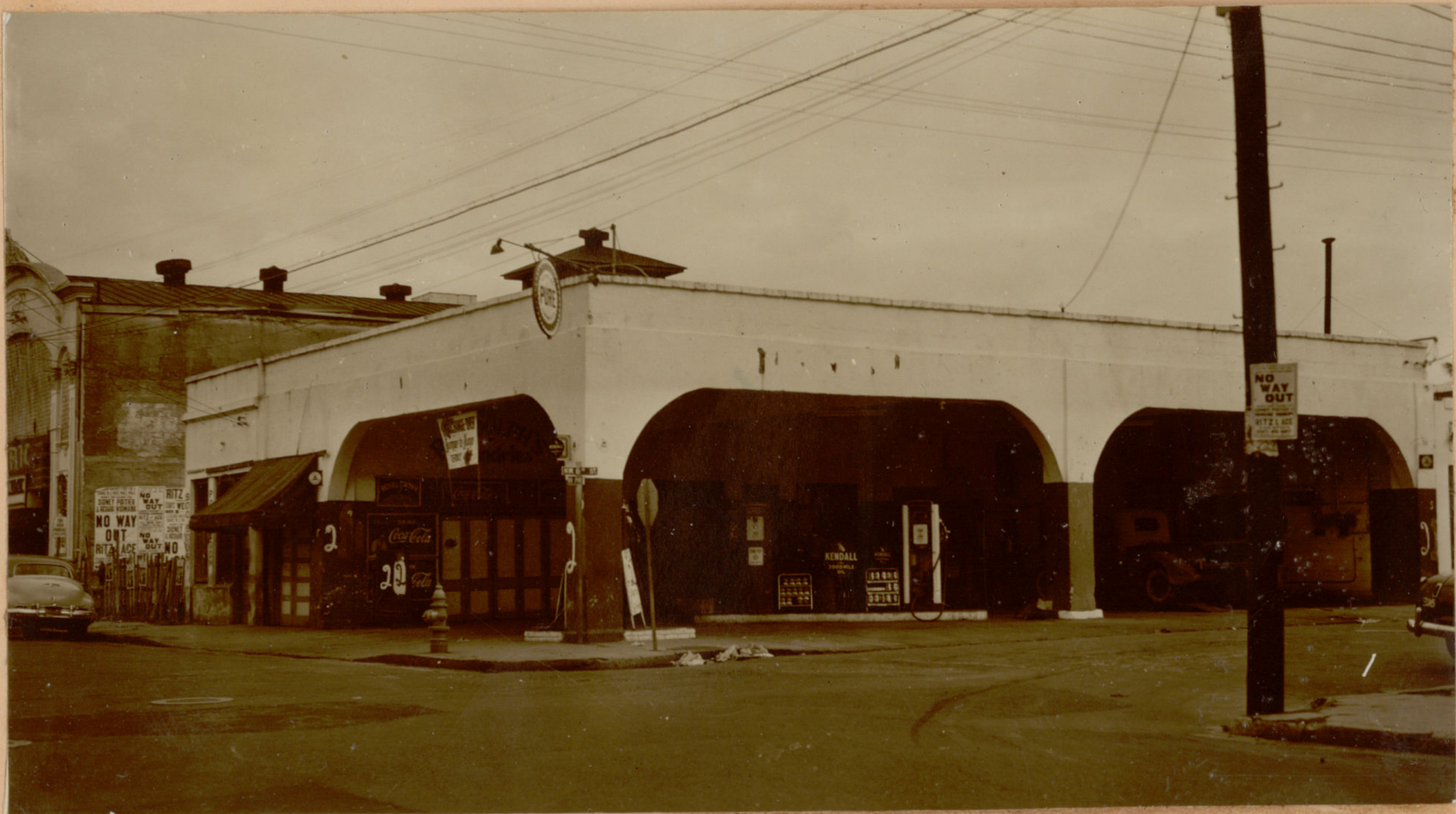
Looking Northeast at West elevation (at left) and part of South elevation (at right)
