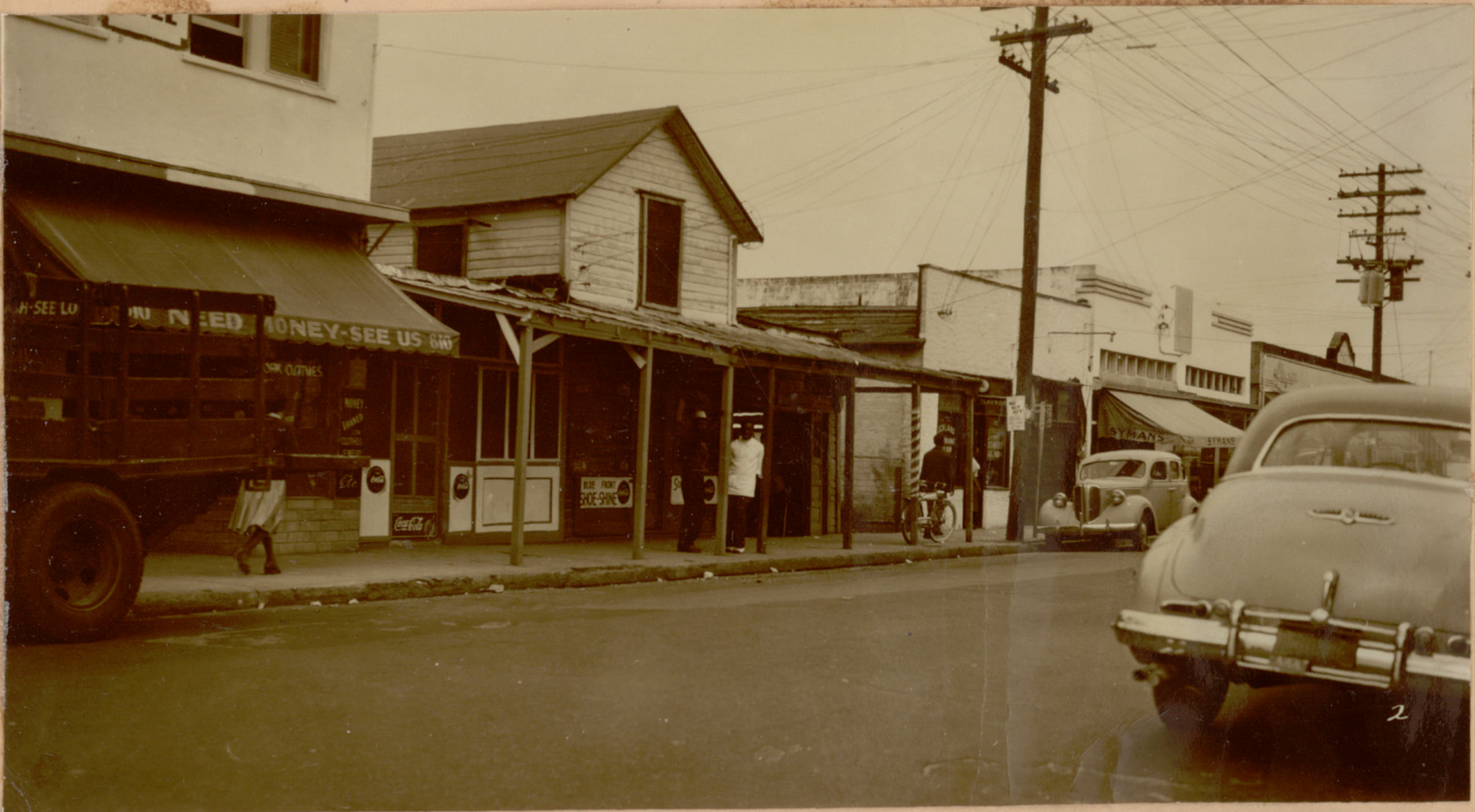
Looking Northwest at front elevation - Buildings at extreme left and at extreme right (white) are not part of subject property
