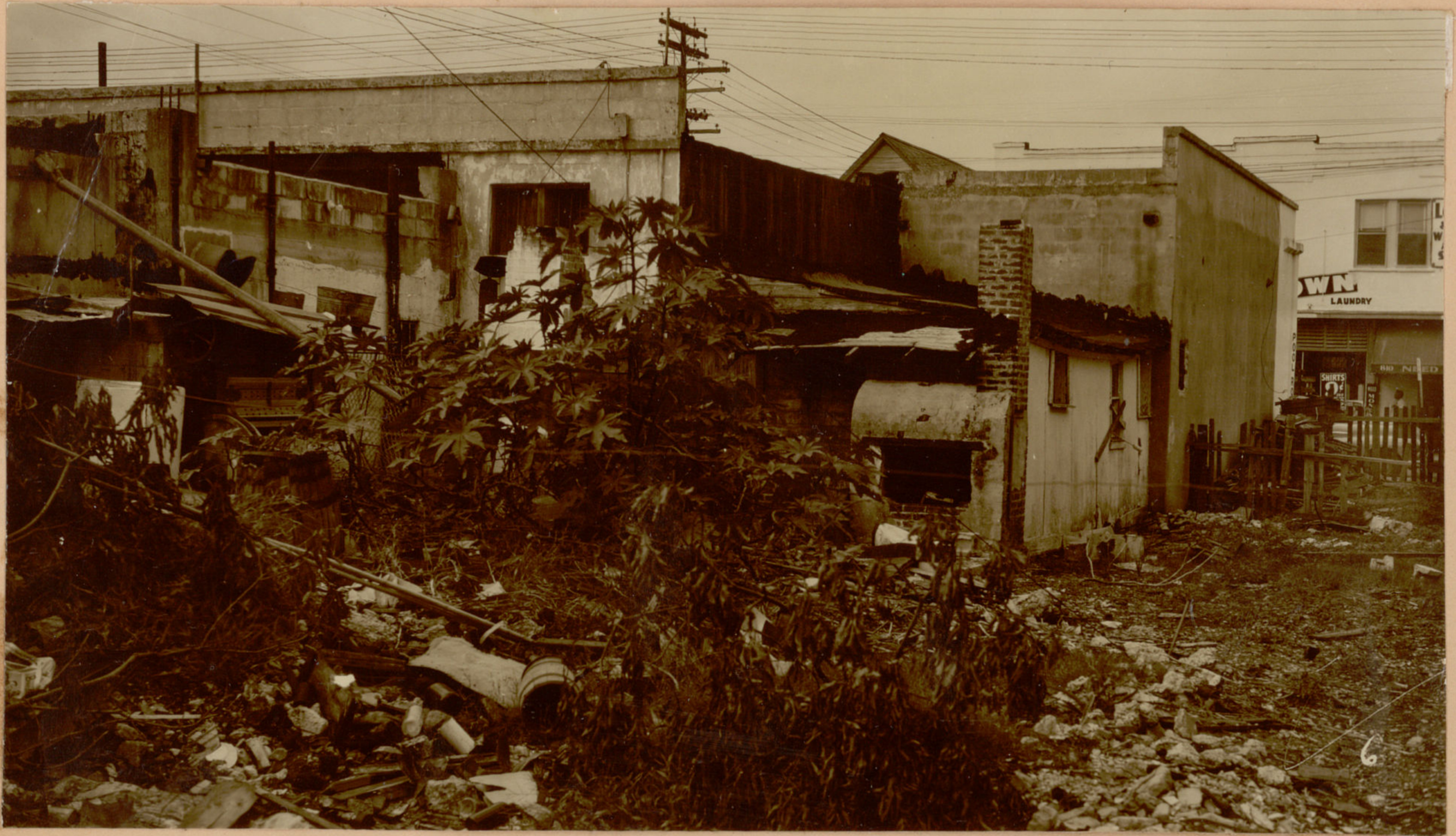
Looking Southwest at rear of buildings facing on N. W. 2nd Avenue and N. W. 8th Street
