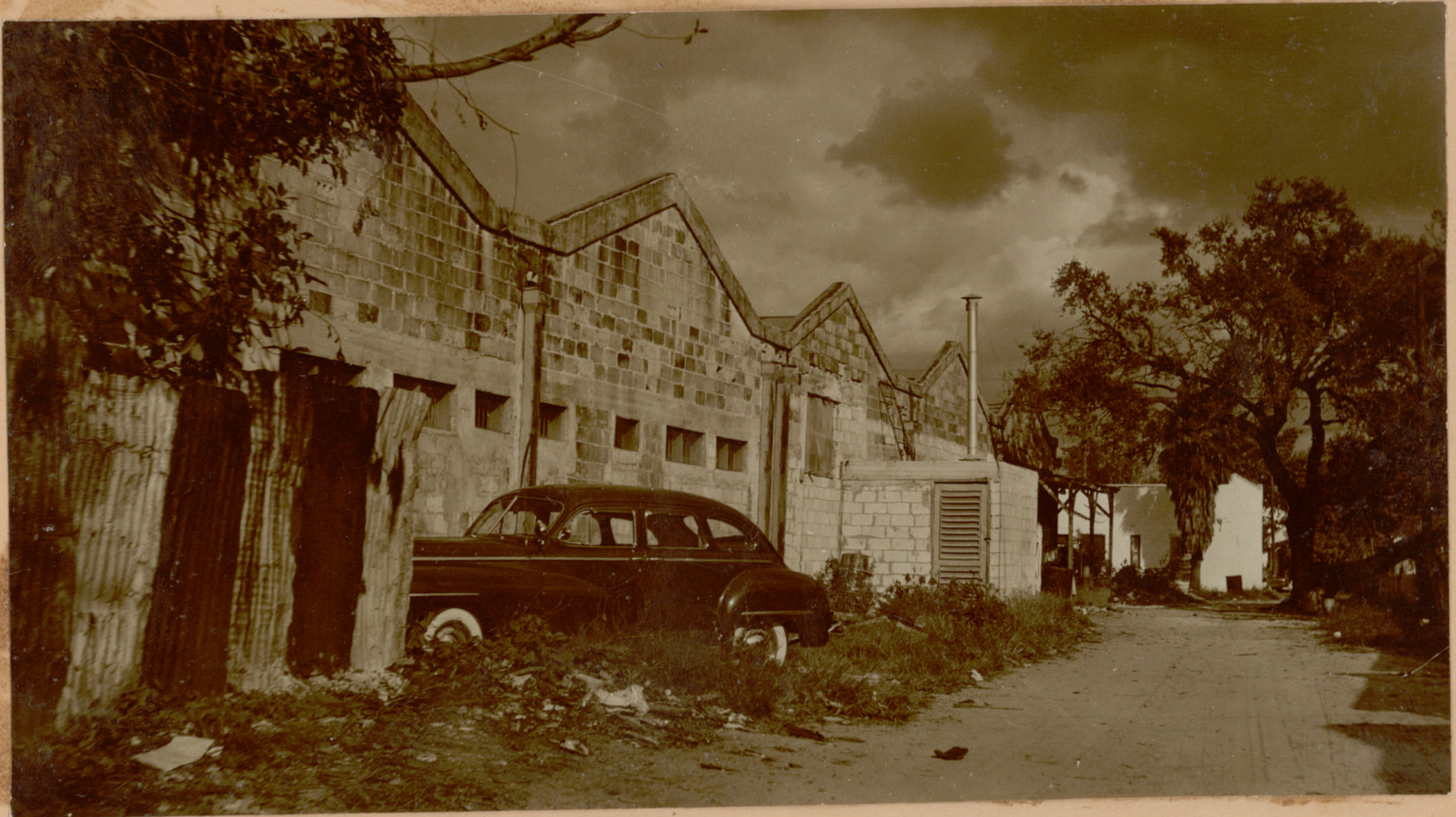
Looking Southeast at converted warehouses
