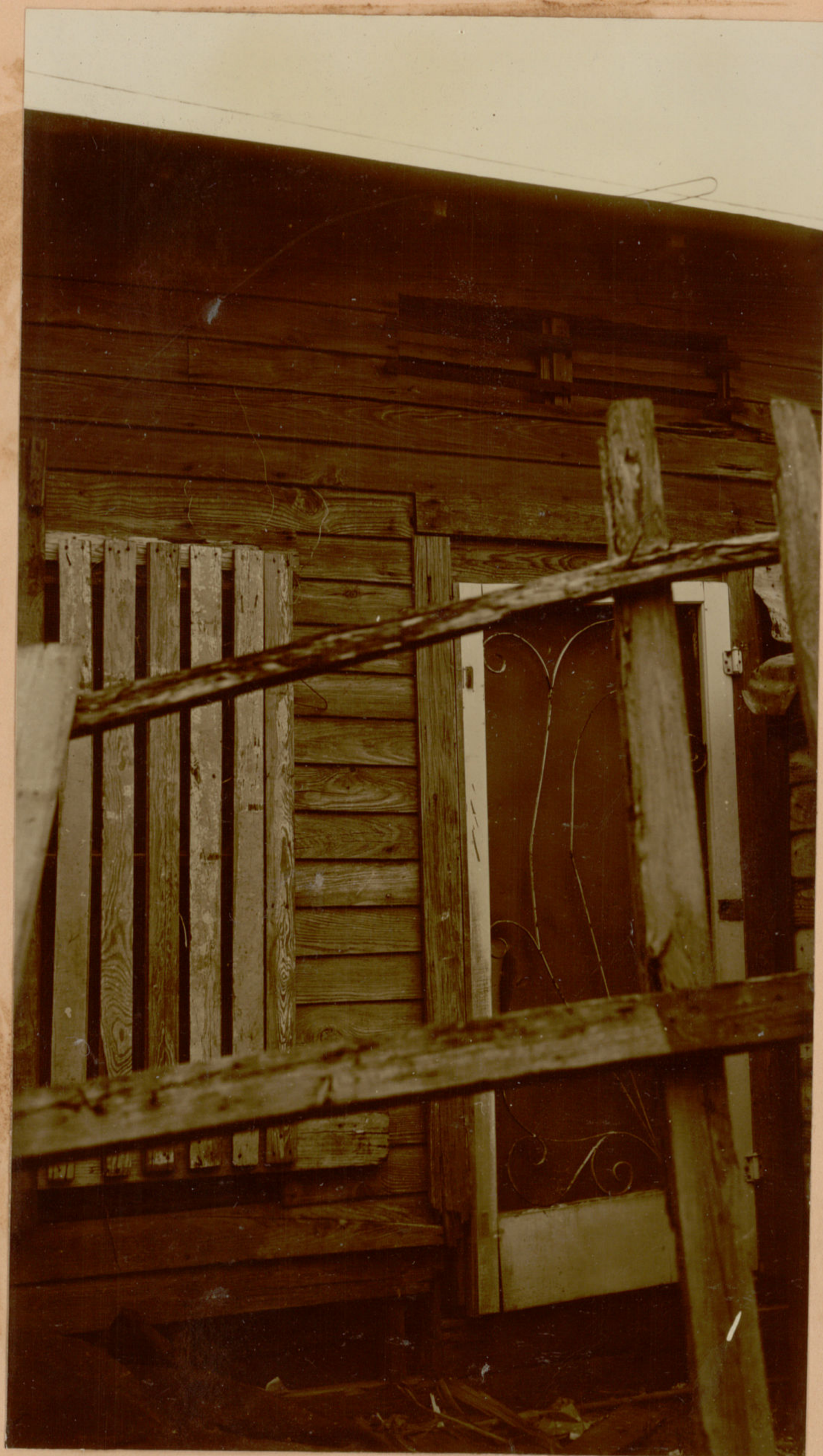
Close-up of Back Door
