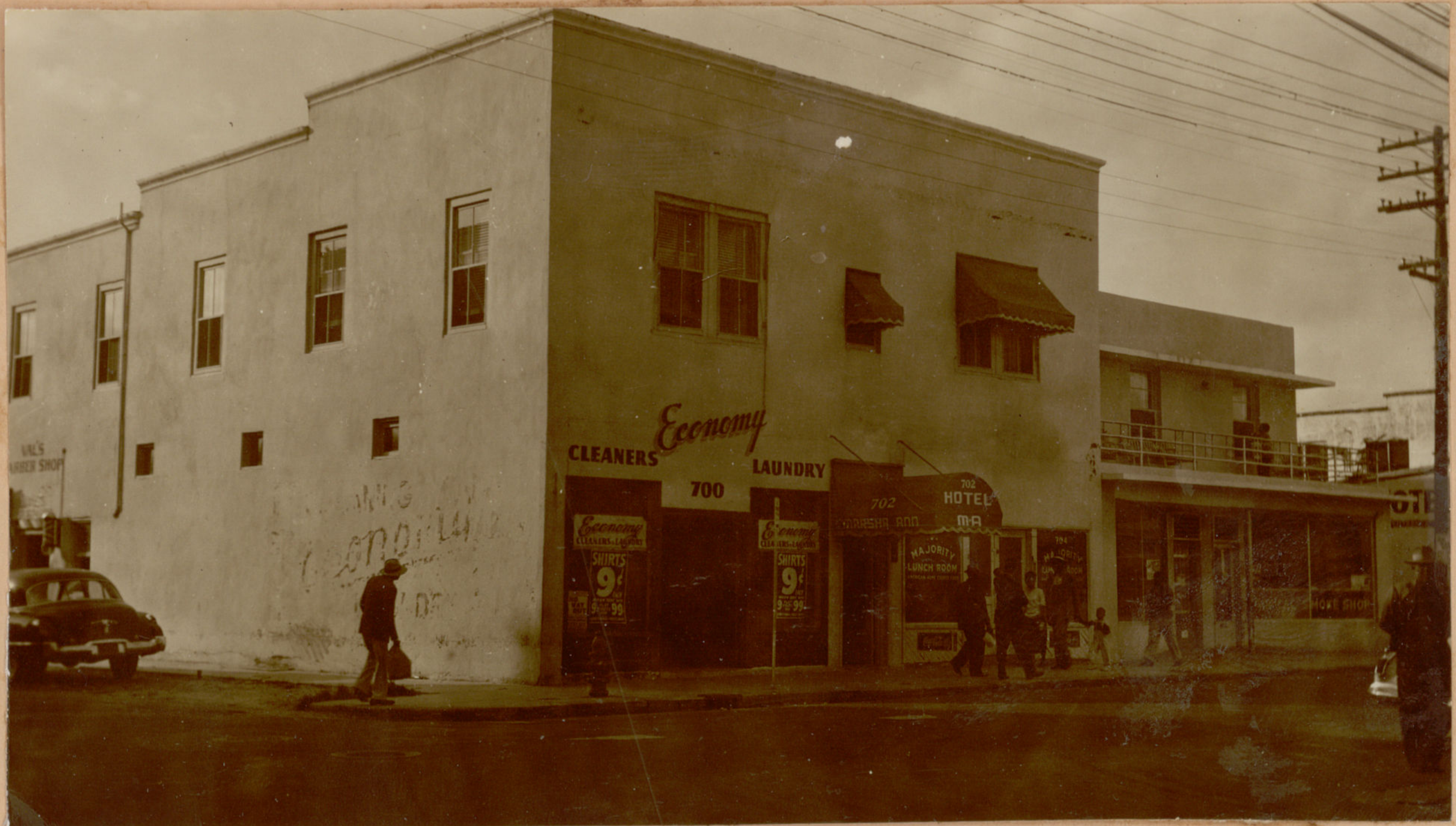
Looking Northwest - South elevation at left and East elevation (front) at right
