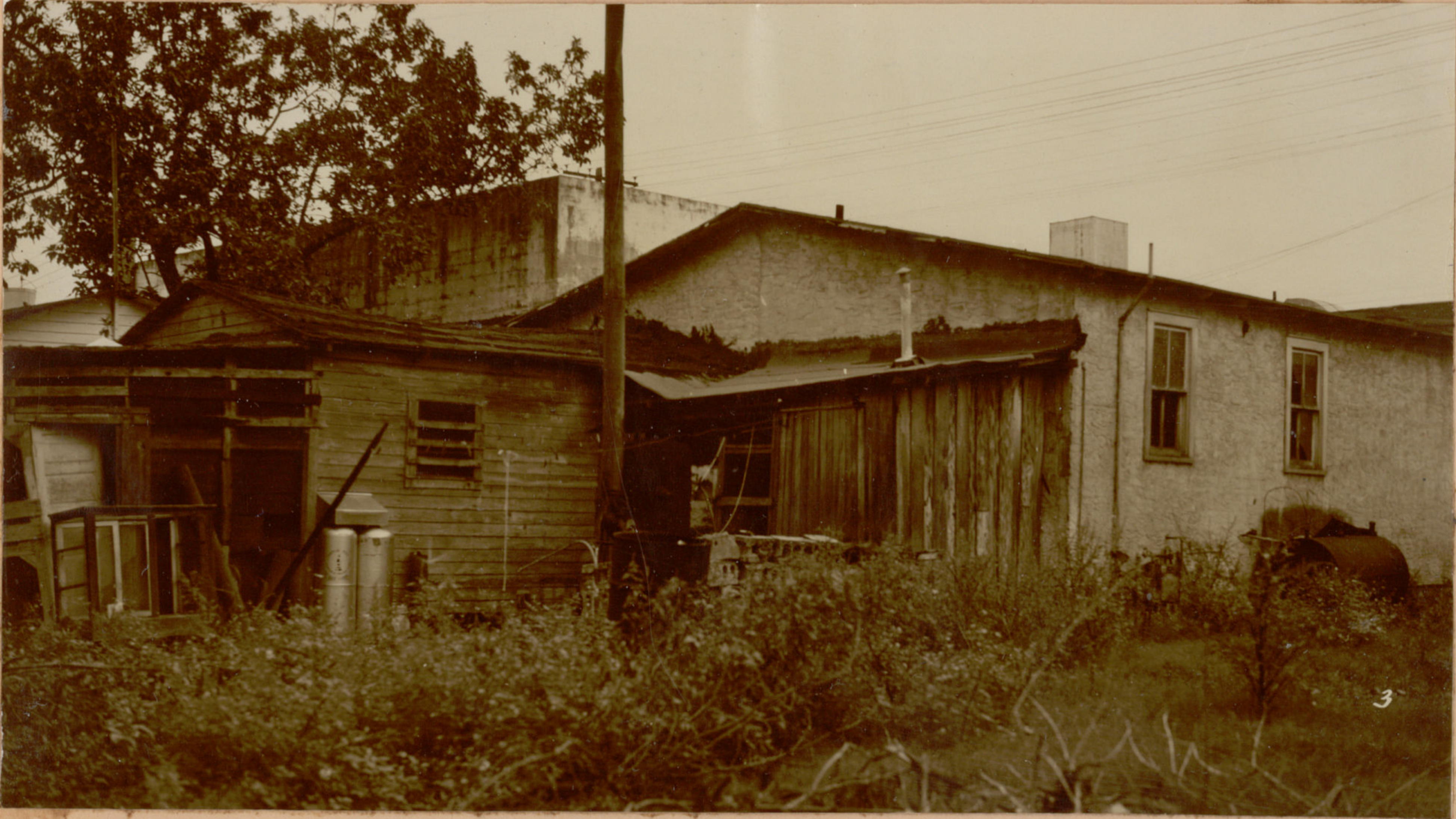
Looking Northeast at rear elevation of building
