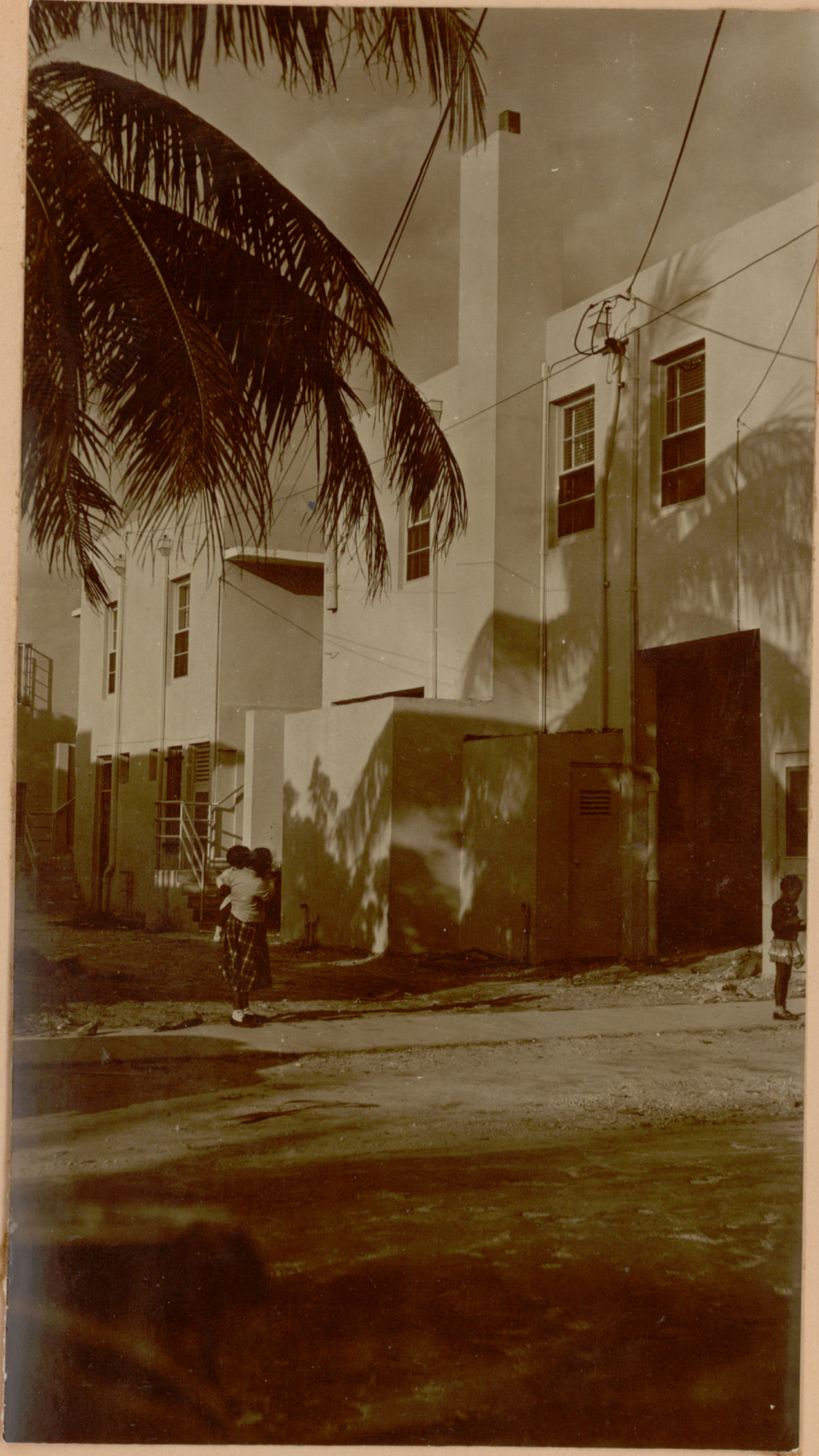
Looking Northeast at West (rear) elevation.
