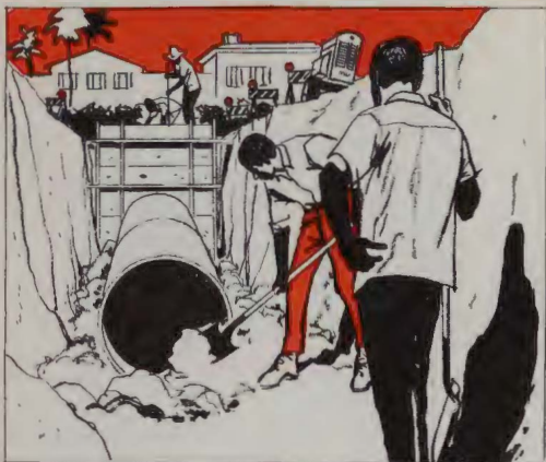
7. Provide for drainage of storm water.
