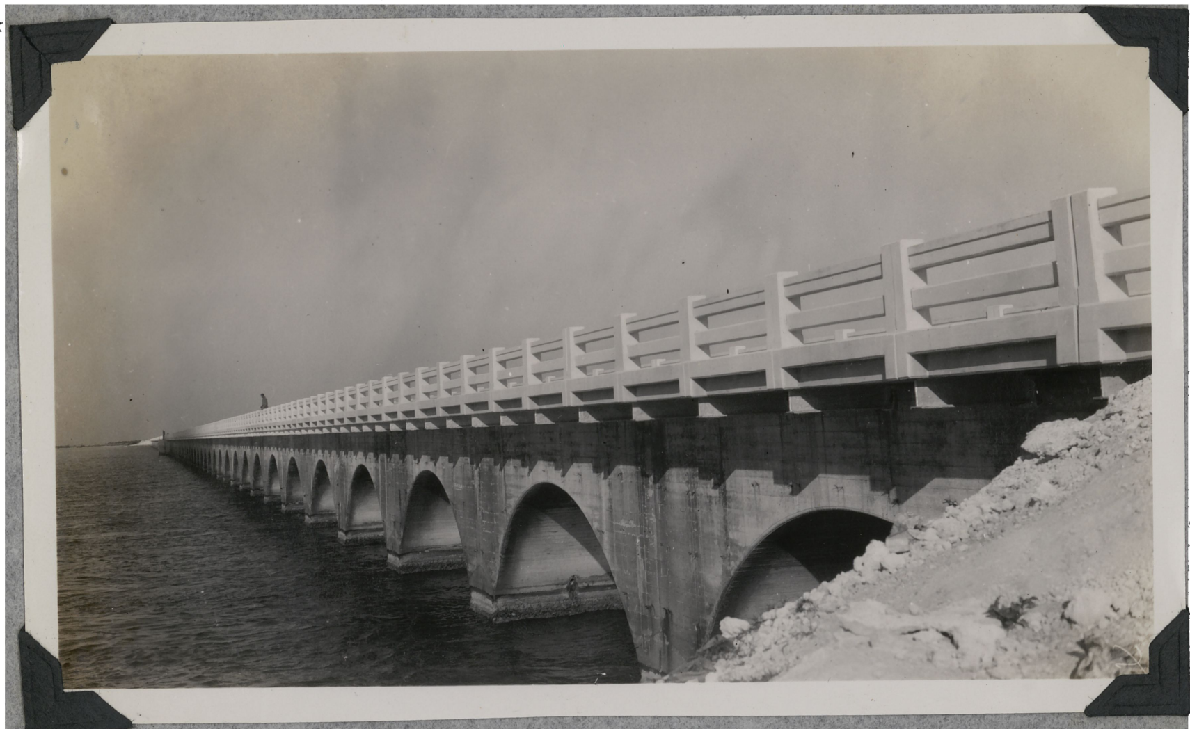
Close up of east end of Long Key Viaduct. The catwalk referred to on page 3 could be suspended from the under side of the bridge deck. The walk could be extended from span to span as the occasion demands.
