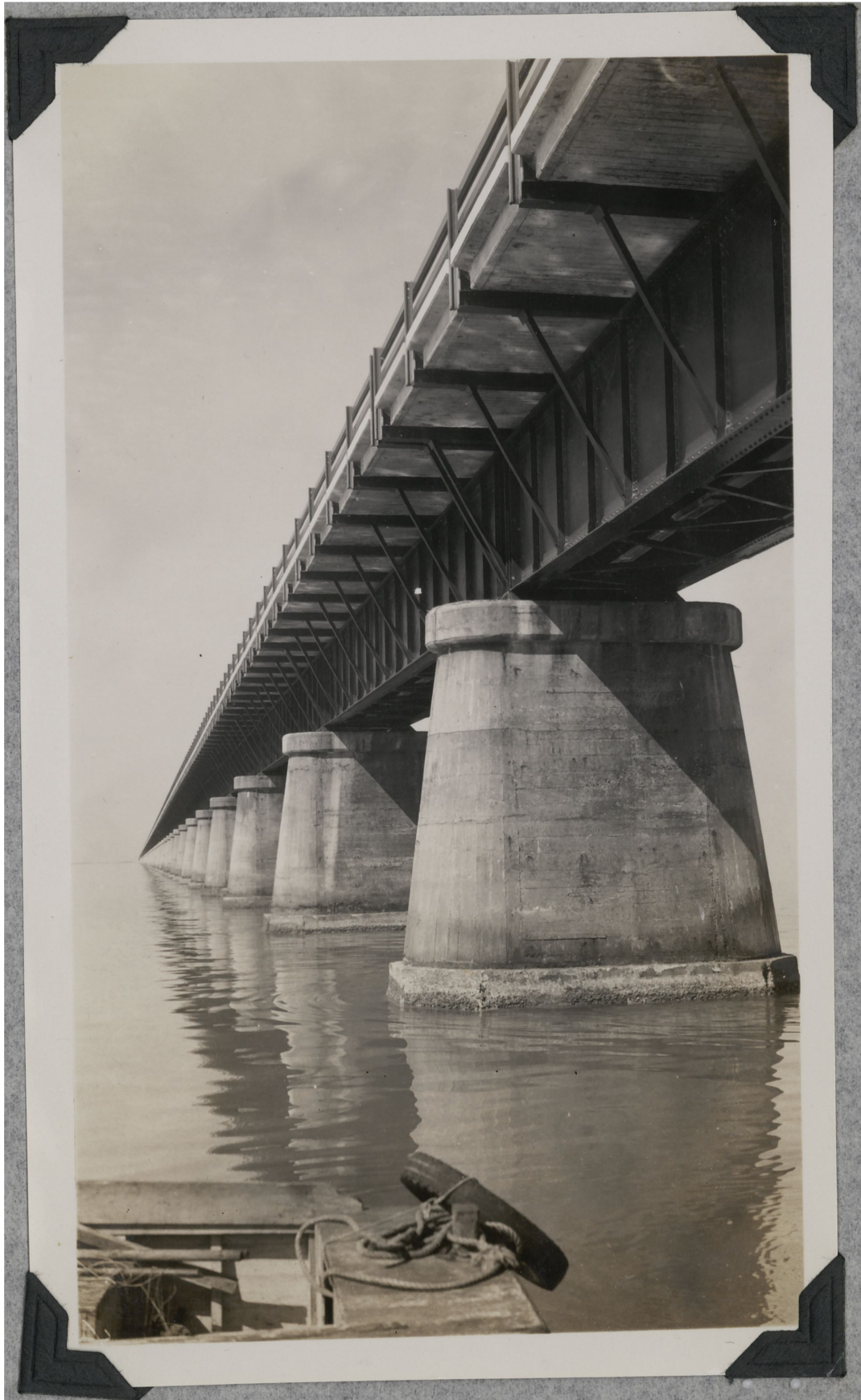
Showing under structure of bridge and possibilities for suspending cat-walk under projecting deck.
