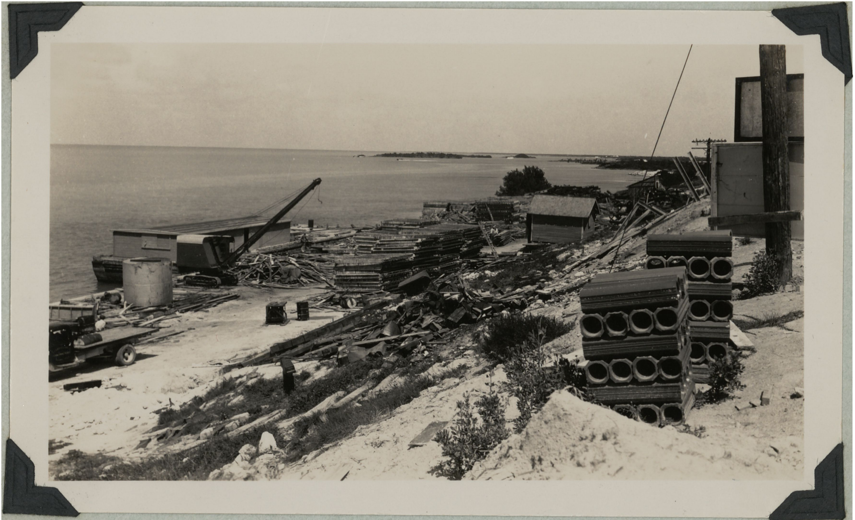
View of docks on Hog Key, north side of highway, looking east. The water is deep enough here to provide docking space for pleasure boats. Parking space on the lower level could be reached by means of a ramp from the highway.
