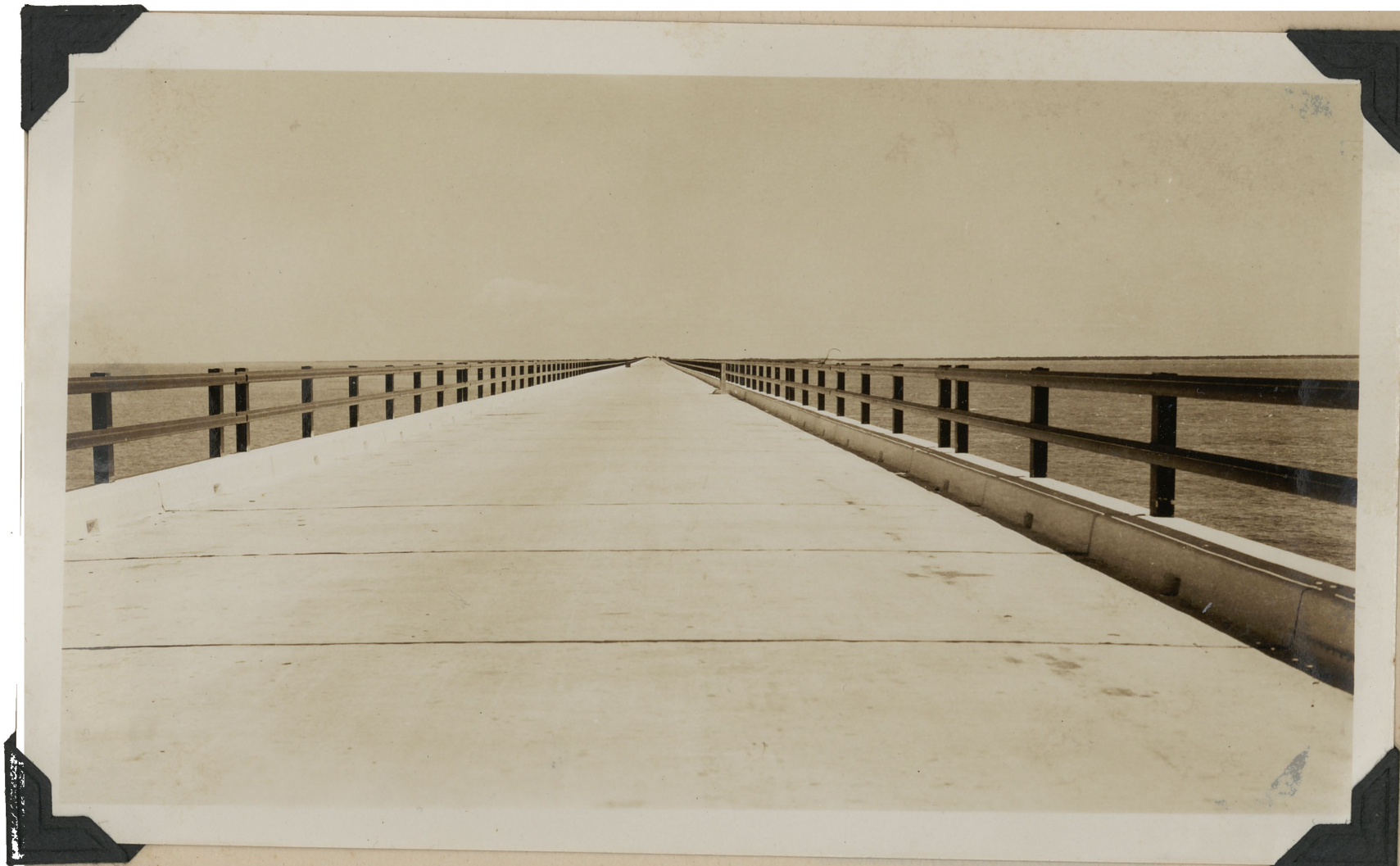
View from deck of finished bridge, directly over Pigeon Key and looking east. Note the railroad rails, formerly the Florida East Coast Railway tracks now being used as railing. The finished color of the rails is aluminum. This picture was taken March 28, the day before the bridge was opened to traffic.
