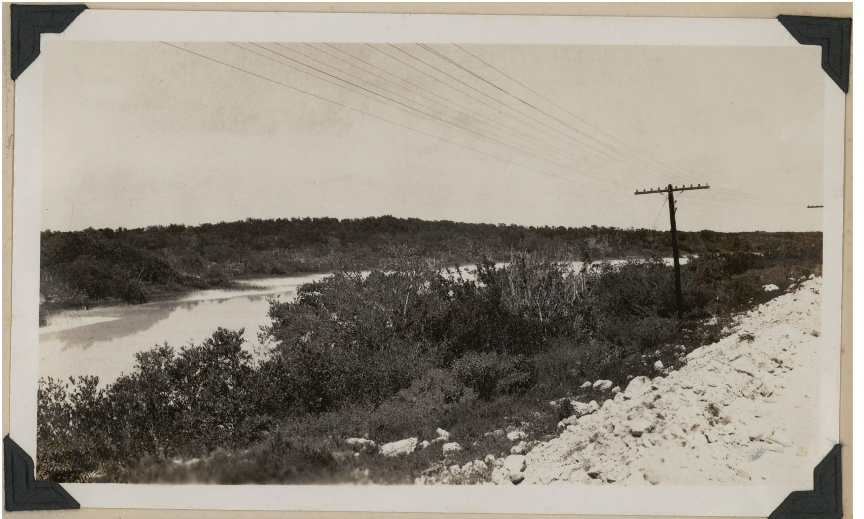
On Bahia Honda Key looking west along north side of highway. Note the marl fill slope at right. A ramp constructed on the side of this fill slope would be required to reach a parkway area below.
