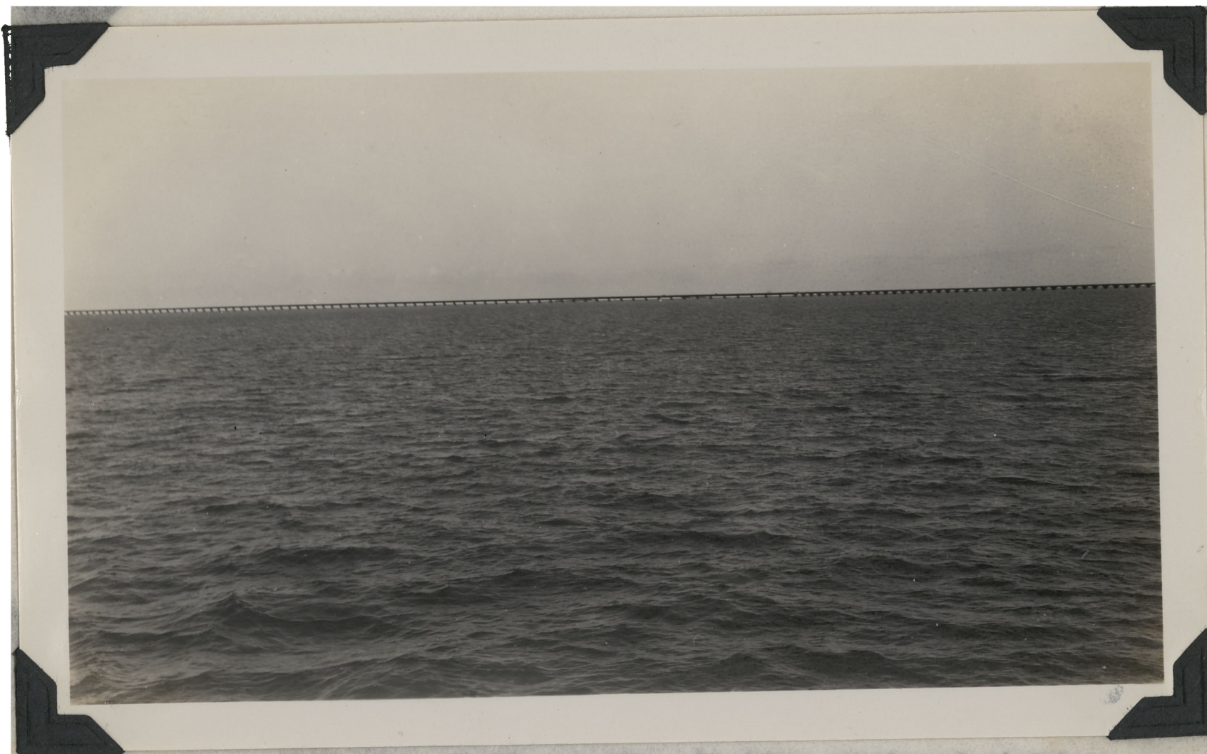
View of north elevation of bridge between Little Buck and Lagoon Key, taken from ferry boat.
