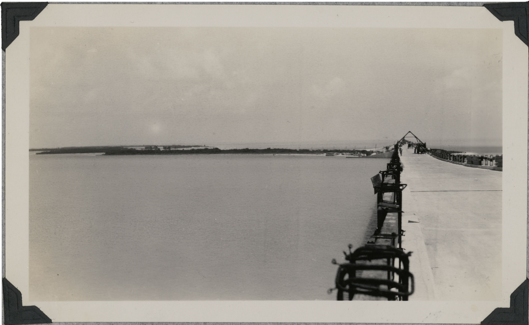
Looking east toward Bahia Honda Key from highest point on high bridge.
