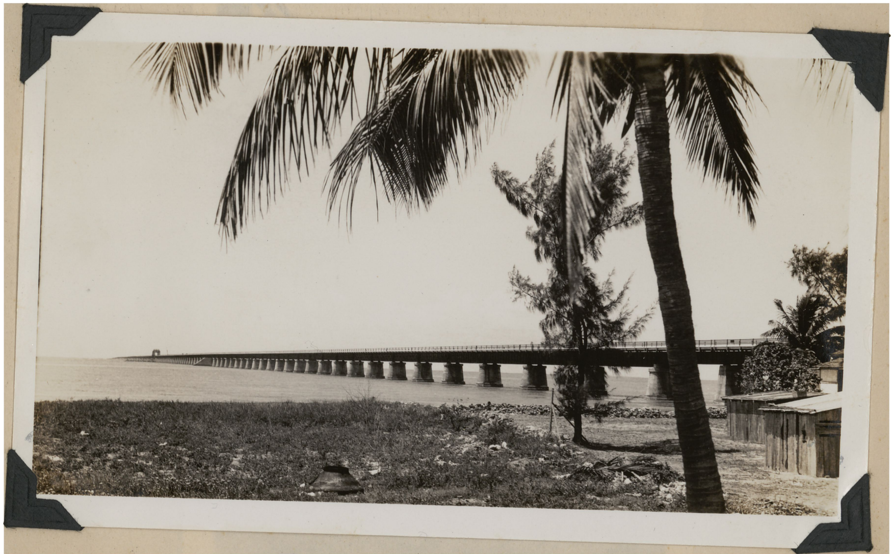
View of bridge from Pigeon Key, looking south west toward Little Duck Key.
