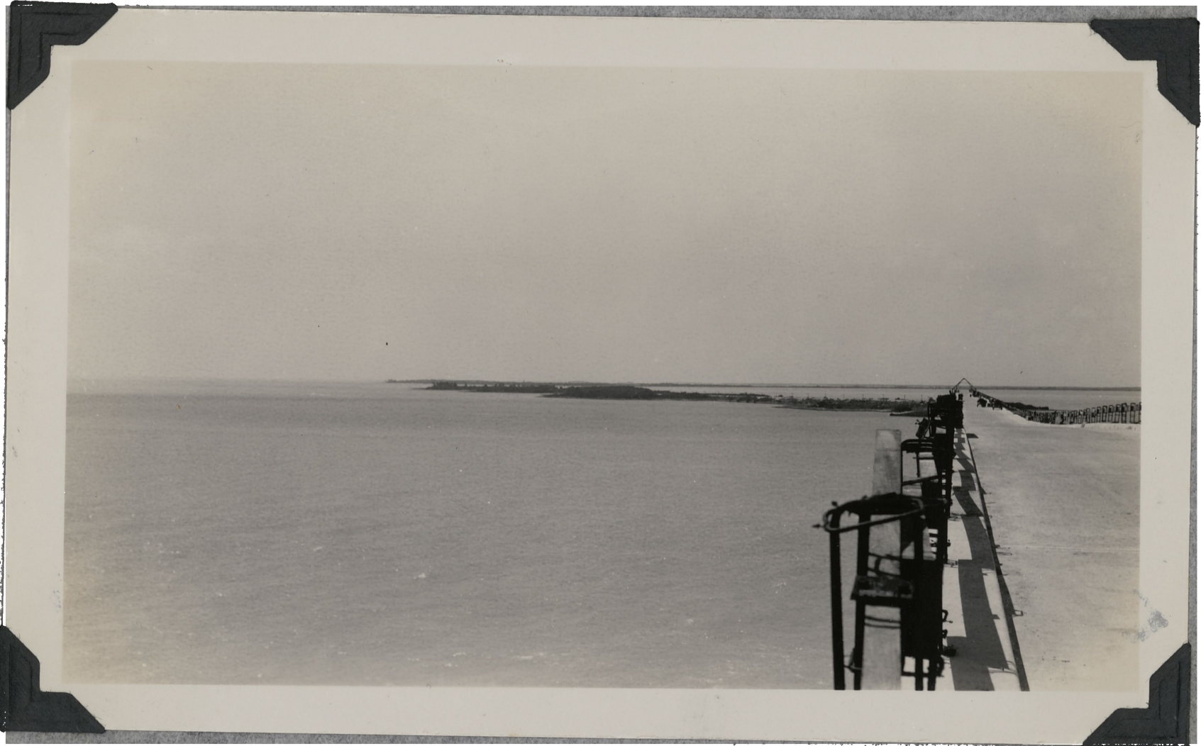
Looking south to Summerland Key from high bridge to Bahia Honda Key. Photo. 0.
