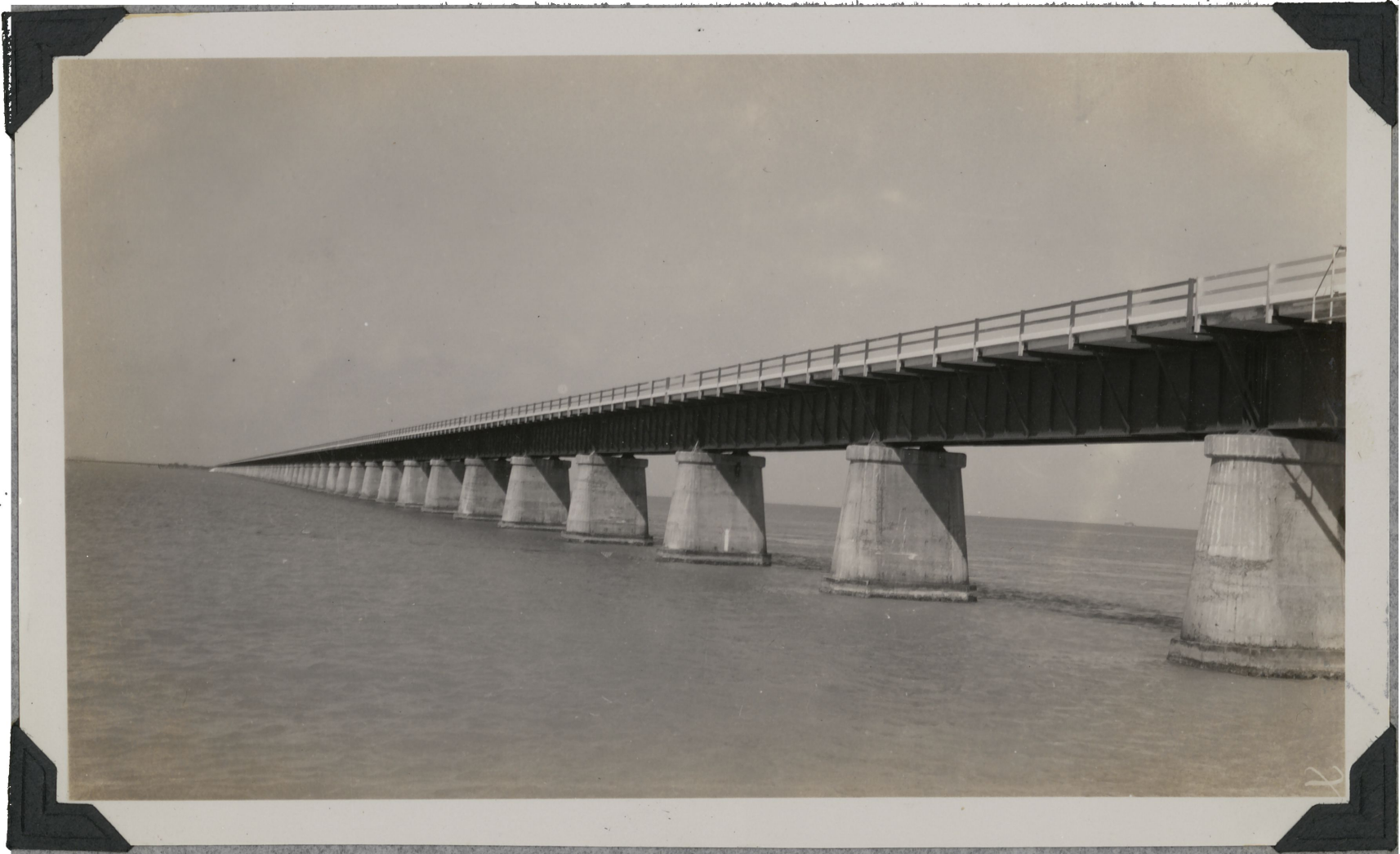
Another good view of the steel span type of bridge completed.
