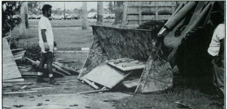
The athletics facilities suffered heavy damage as a result of Hurricane Andrew.
