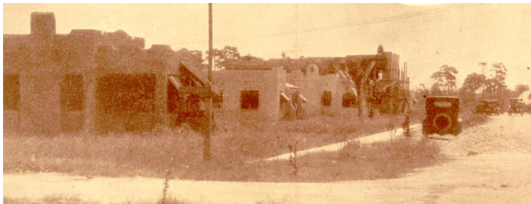
At NE 11th Avenue at NE 127th street looking north are single-family dwellings and an apartment house all under construction in 1924. A photo blow-up showed workman on the apartment roof and the roofing trash chute hanging on the front of the Corner house. Other photos show awnings up during construction?
