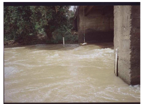
Figure 4. 3. The Sampler is suspended by a bridge crane during flooding at the Kapkimolwa (Amala) Bridge.
