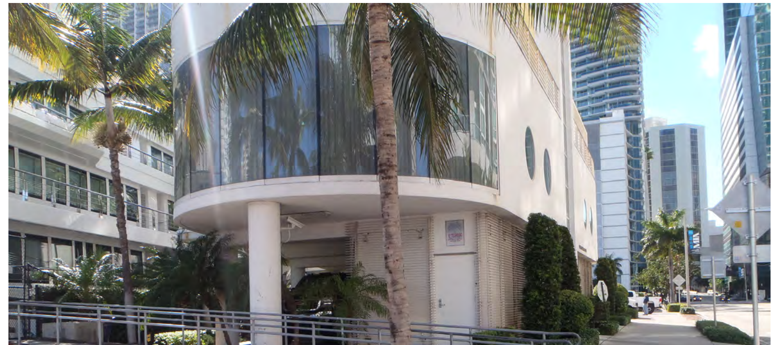
Existing Condition (looking east)
