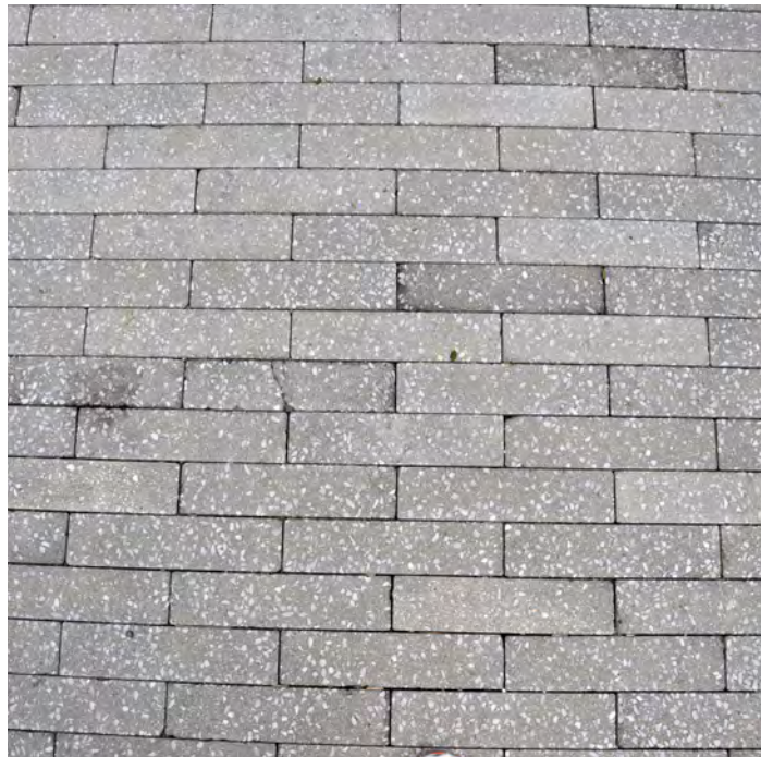
PAVING - NORTH SIDE
