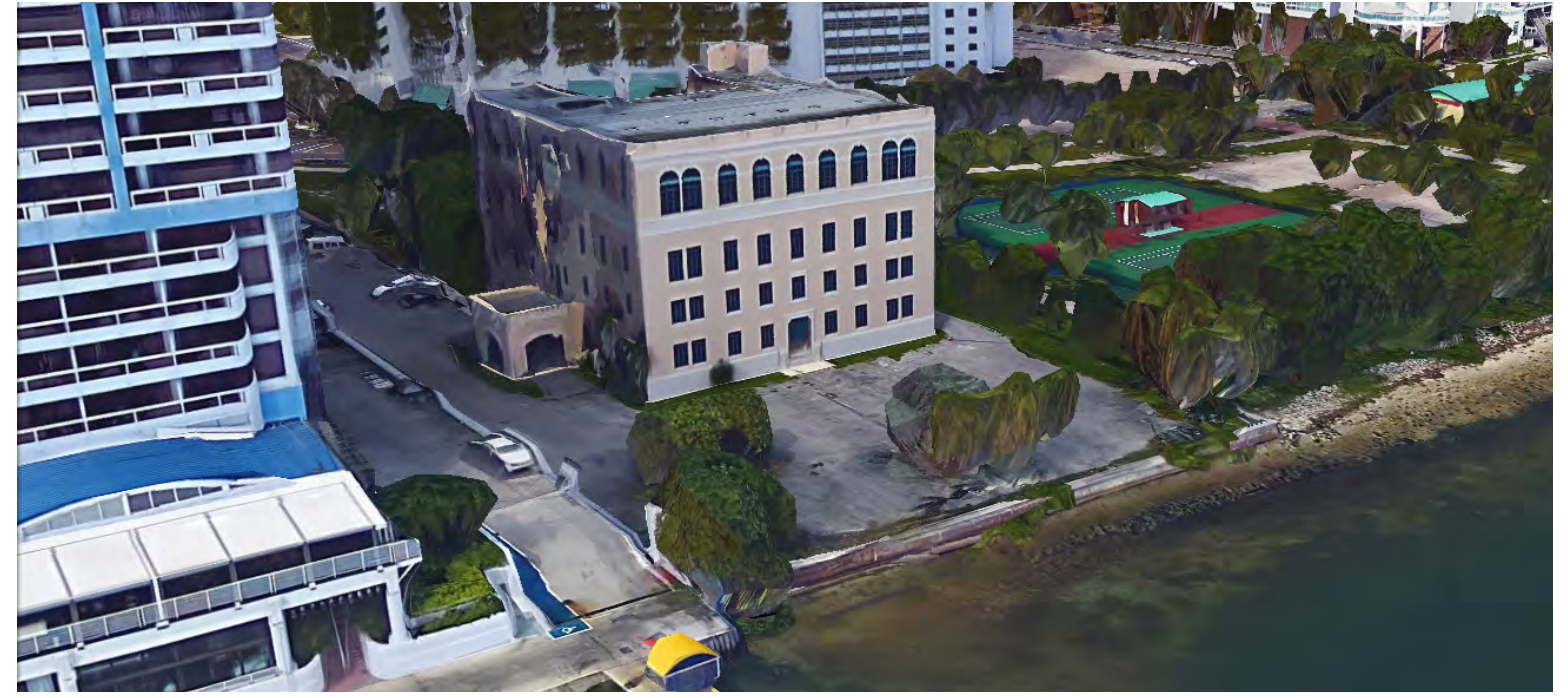
Existing Condition (looking north from Double Tree Marina)
