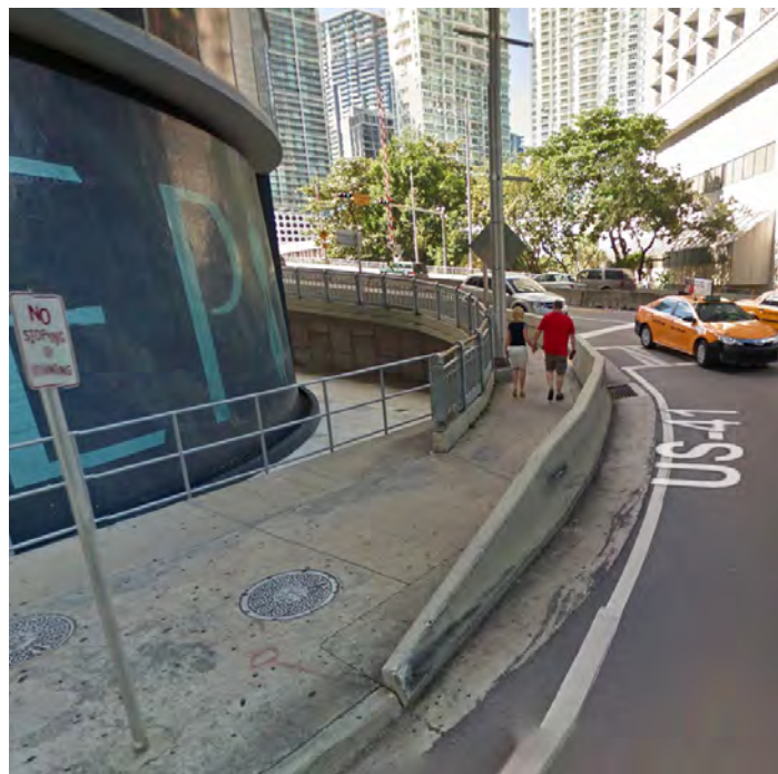
BRICKELL BRIDGE LOOKING SOUTHWEST
