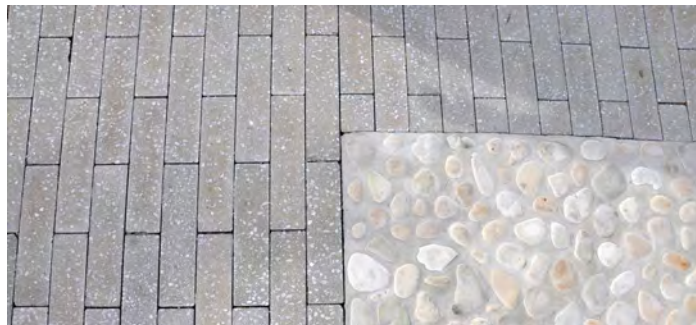
PAVING - NORTH SIDE
