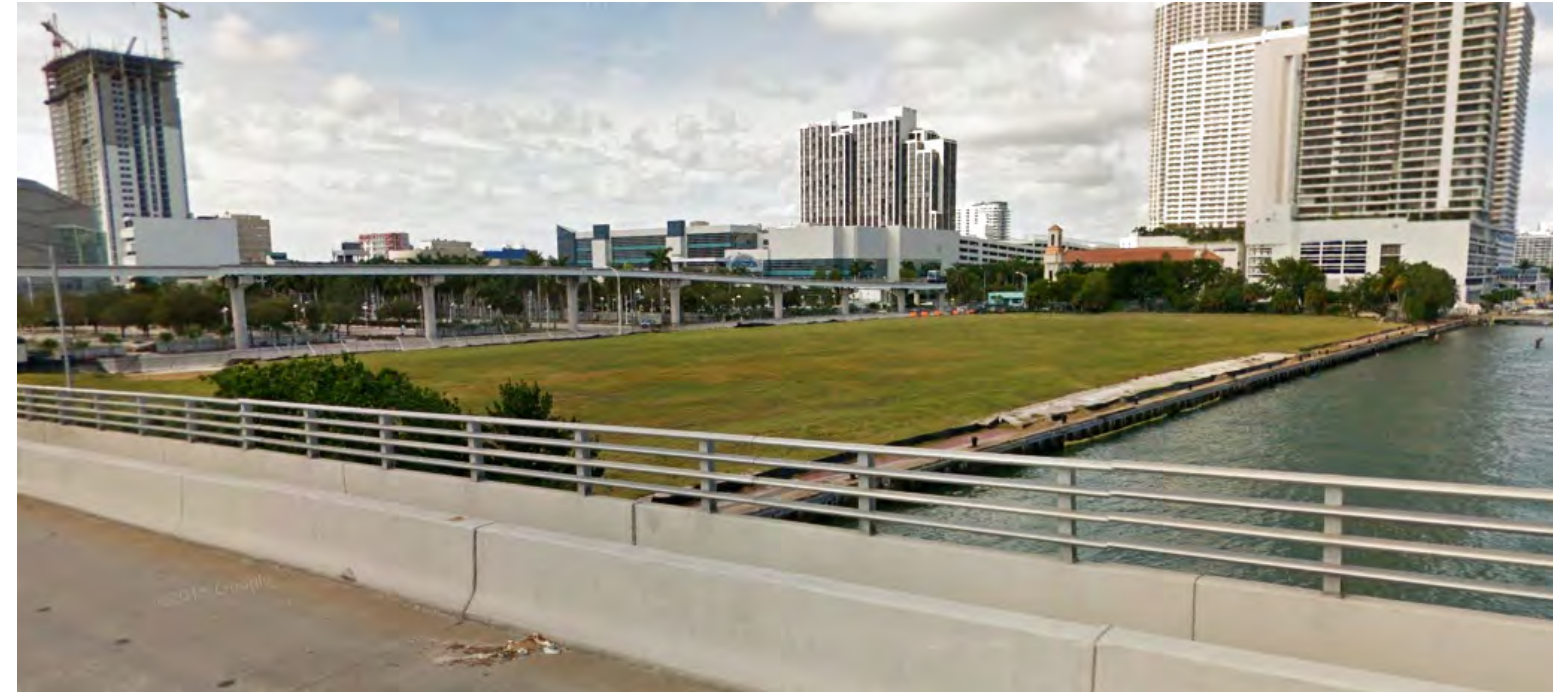
Existing Condition (looking north from MacArthur Causeway)
