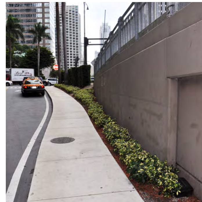
APPROACHING BRIDGE FROM MIAMI CIRCLE
