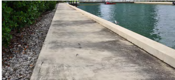
PAVING - SOUTH SIDE
