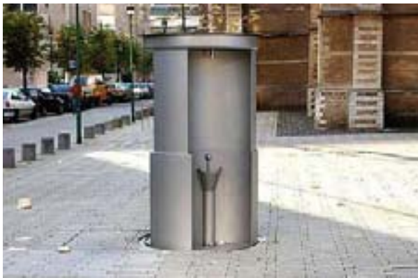
UriLift Reading, UK Pop-up urinal, which rises out of the street in the evening, and goes back down around 6 in the morning. Underground, it is connected to water pipes and electricity, and includes an automatic flushing and cleaning system.
