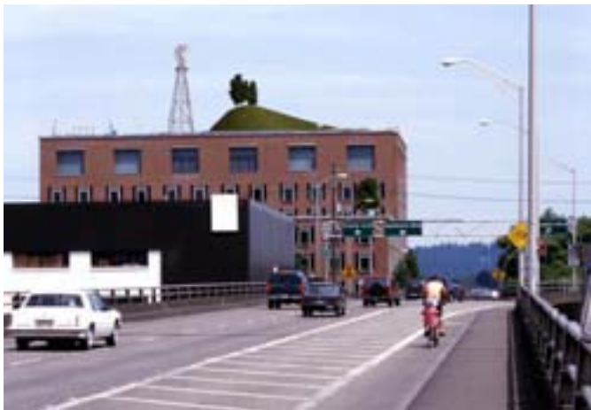
Noel Harding Green Roof Sculpture , 2001 Multnomah County Building, Portland Oregon
