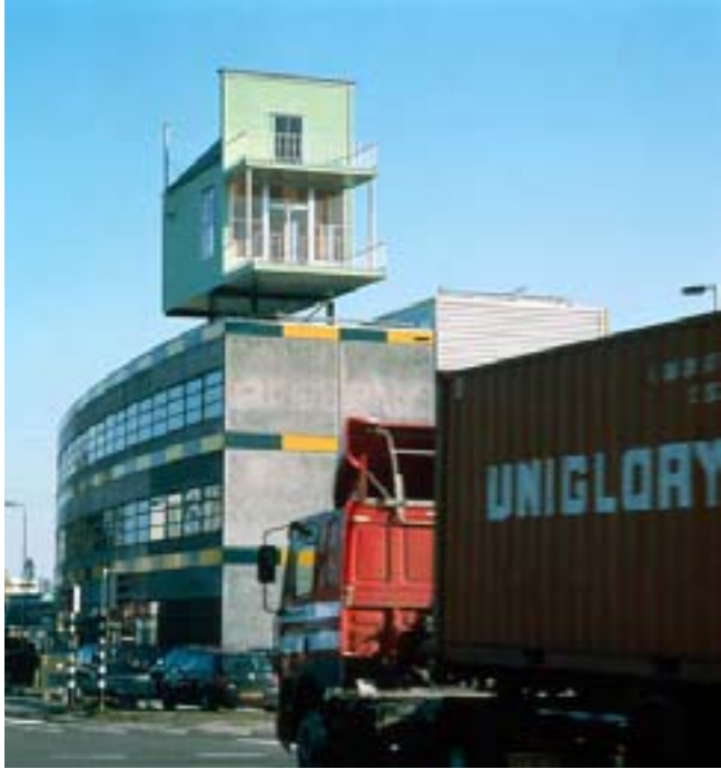
John Kormeling Pioneer House Rotterdam, Netherlands Customs building at the harbour
