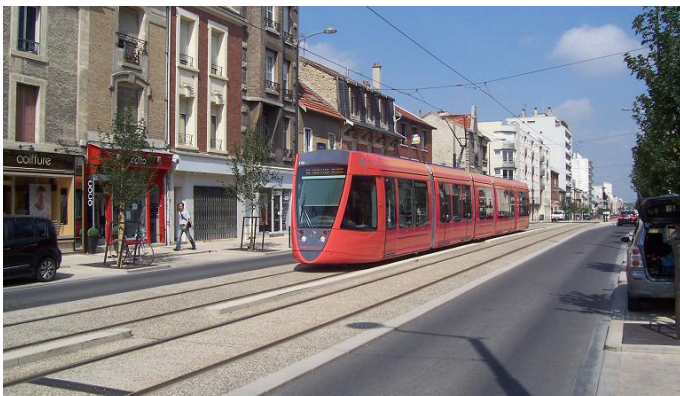
FIGURE 4.25: OVERHEAD CONTACT SYSTEM (OCS) IN REIMS, FRANCE
