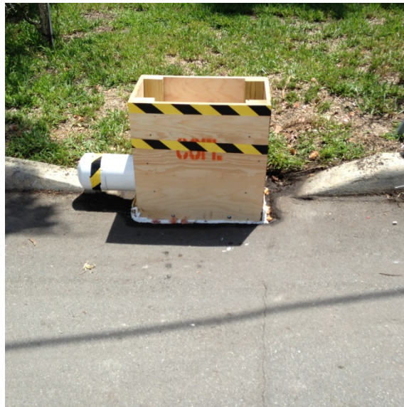
Figure 2 - Catch Basin on Mola Drive with a Temporary Tidal Box Deployed.
