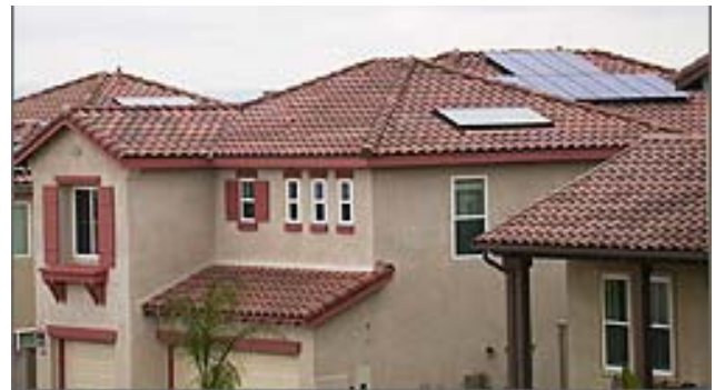
New technology is allowing roof top solar collectors to become smaller.
