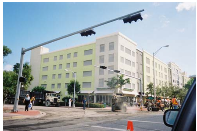
An upper-story parking garage wrapped by ground-level retail uses.
