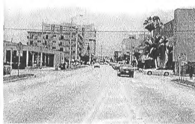
71st Street - View Looking East
