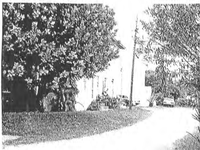
Existing House at Altos Del Mar
