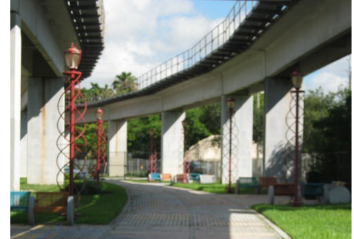
VIEW SOUTH AT PROJECT START AT 7 TH AVE.
