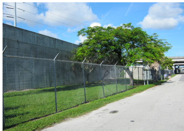
VIEW WEST TO SMALL FPL BUILDING AND METRORAIL
