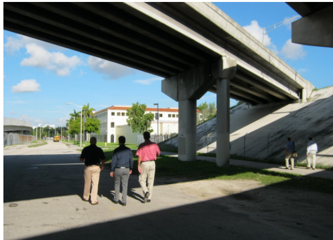
VIEW TO THE WEST BELOW I-95
