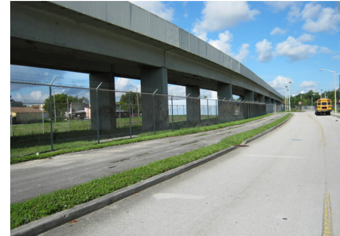
METRORAIL ELEVATED RAILS
