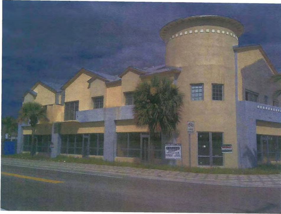
Commercial Façade Program – Antilla Plaza Before
