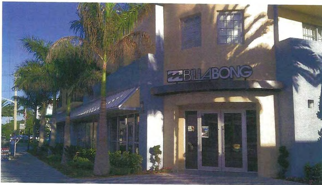
Commercial Façade Program – Antilla Plaza After Anchored by Billabong Surf Shop
