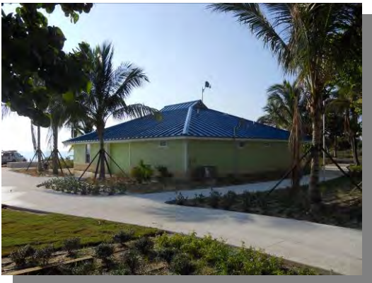
Ocean Rescue Bldg
