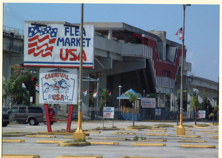
Community Stations serve areas larger than their immediate surroundings. These station areas may provide moderate to high levels of new development or redevelopment potential. Community Stations will be accessed by kiss-and-ride and park-and-ride users and local buses. Walk-up use may also be significant.
