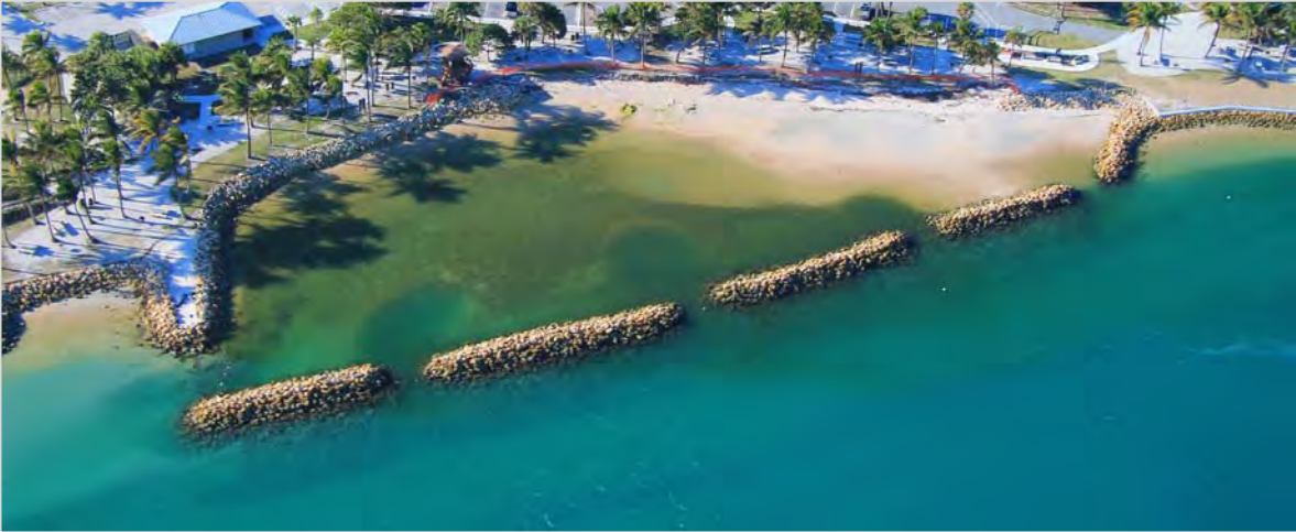
Limestone boulder breakwaters at Dubois Park (Jupiter Inlet) help to protect the Park's shoreline and provide hardbottom habitat for a diverse array of marine life.
