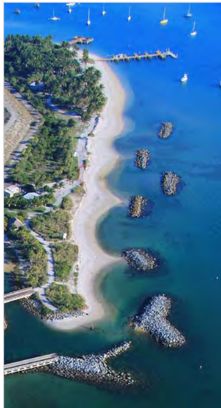
Limestone boulder breakwaters at Peanut Island Park (Lake Worth Inlet) protect the Park's sandy shoreline and form salients (portion of shoreline connecting to the breakwater) behind the structures.
