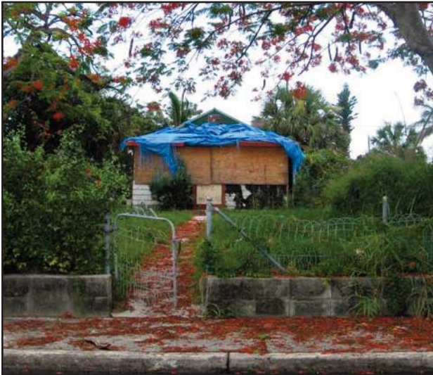
Some parts of neighborhoods have fallen into disrepair
