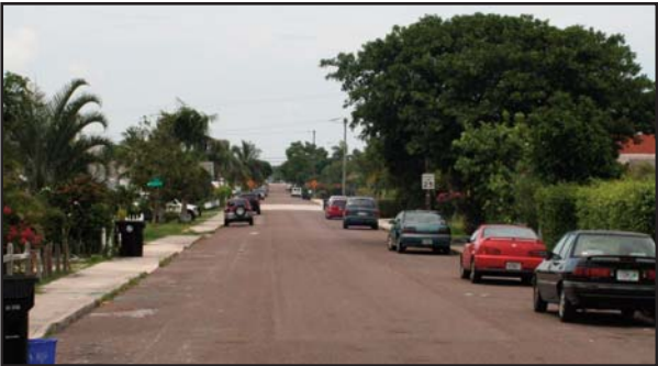
Most of the city’s streets are appropriately scaled, with on-street parking that acts as a natural traffic calming device.
