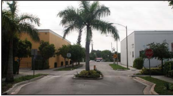
This median in downtown West Palm Beach makes drivers slow at a “T” intersection.
