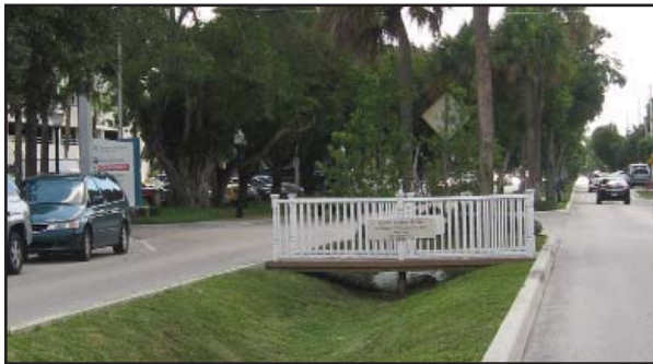
This median in downtown Stuart provides drainage. A bridge has been donated by a local business. Trees continue to define the street space and calm traffic.
