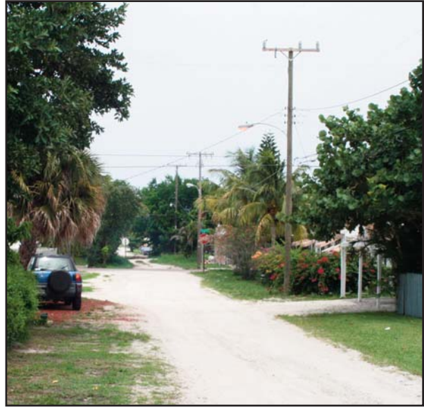
Some of the roads within the study area are not paved, resulting in an uninviting environment for pedestrians and bicyclists.
