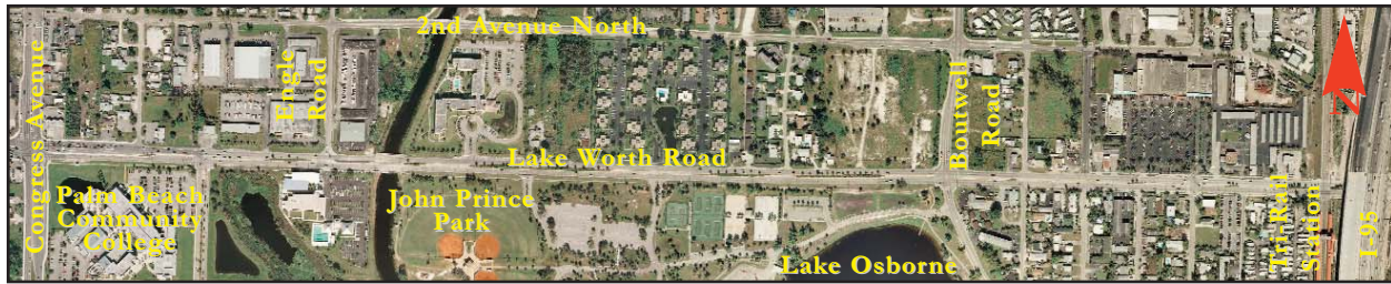
This section of Lake Worth Road holds major destinations such as Palm Beach Community College, John Prince Park, the southern edge of the Park of Commerce, the Tri-Rail station, and Lake Worth High School.
