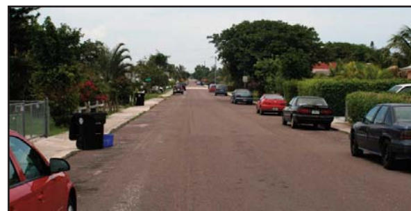
This photo is a typical one-way neighborhood street in the City of Lake Worth that measures 30 feet from curb face to curb face, which is sufficient asphalt to carry two-way traffic with on-street parking.
