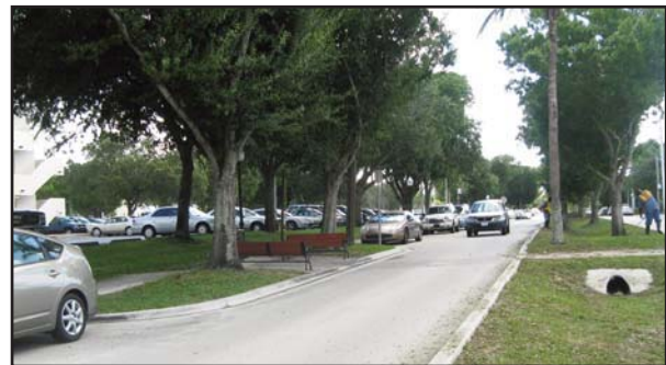
Chokers narrow the lane. This choker in downtown Stuart provides two benches under shade trees.
