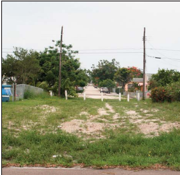
Road closures interrupt the street network.
