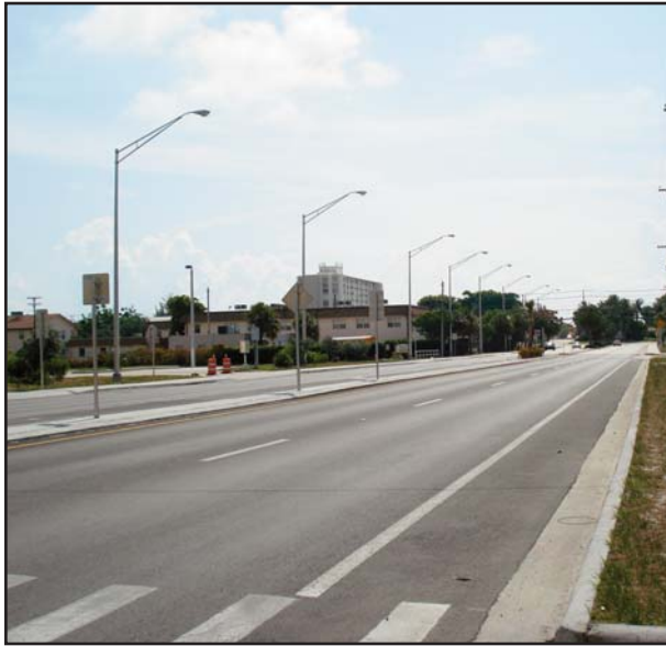
As development extends west, the street becomes more suburban and dangerous for pedestrians
