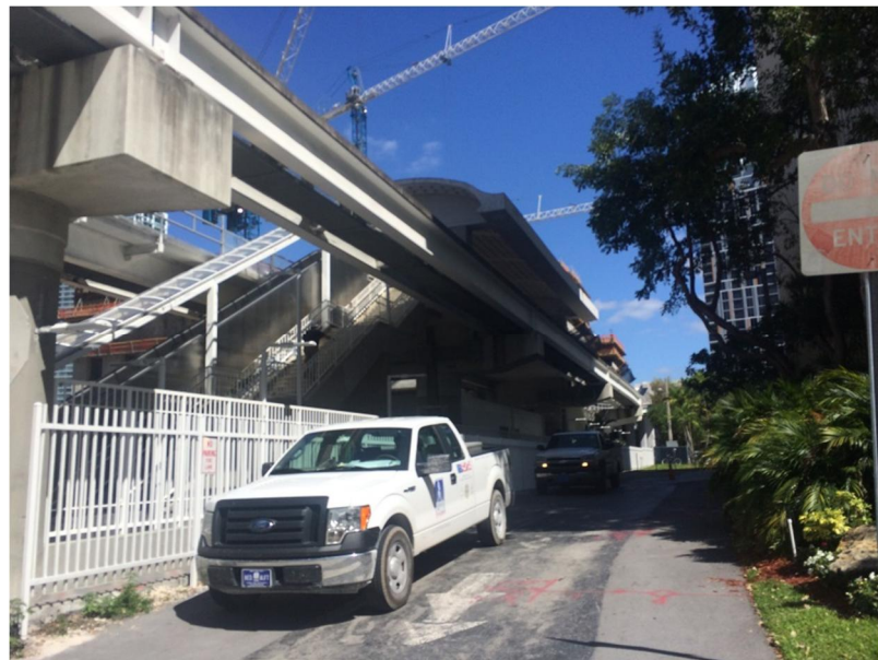
Photo 50: 8th Street Metromover Station
