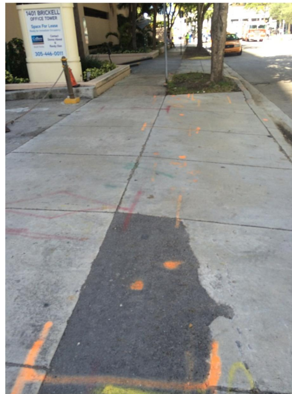
Photo 16: SE 14th Street
