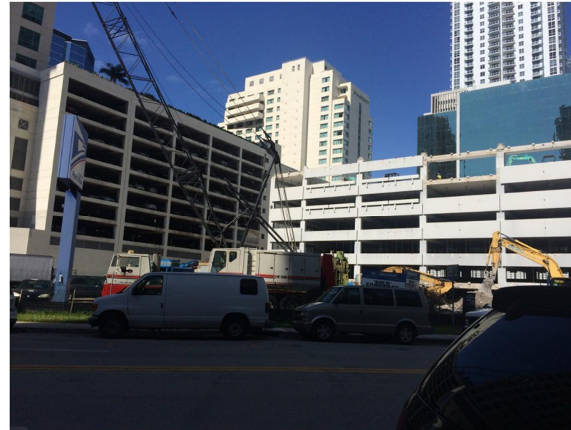
Photo 28: Brickell Bay Drive
