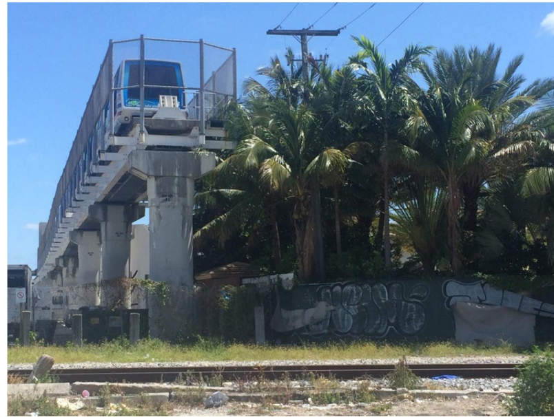
Photo 57: End of Line, School Board Metromover Station
