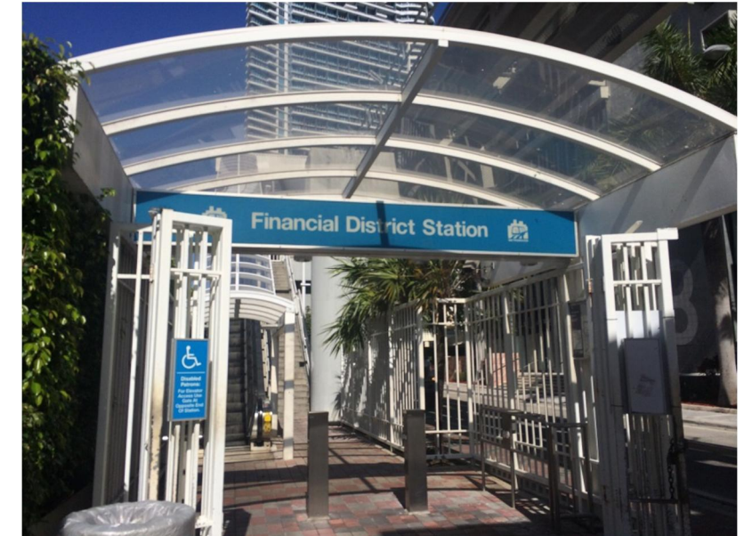
Photo 5: Financial District Metromover Station
