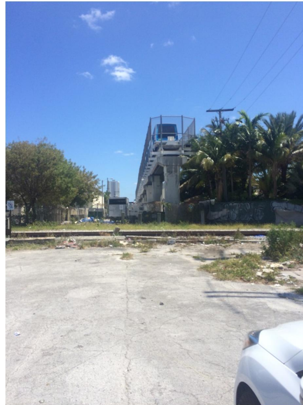
Photo 58: End of Line, School Board Metromover Station
