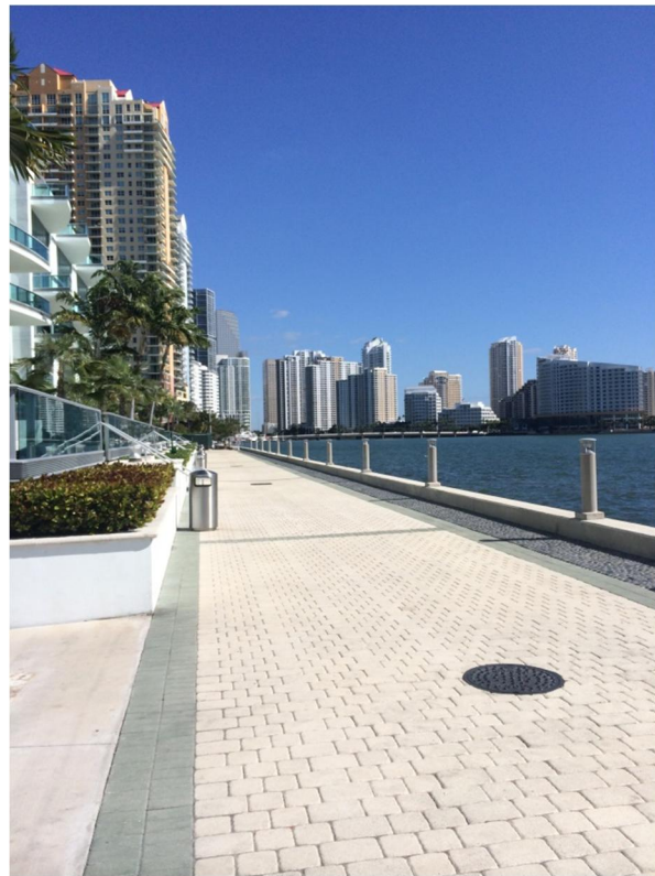
Photo 20: Jade at Brickell Bay Seawall
