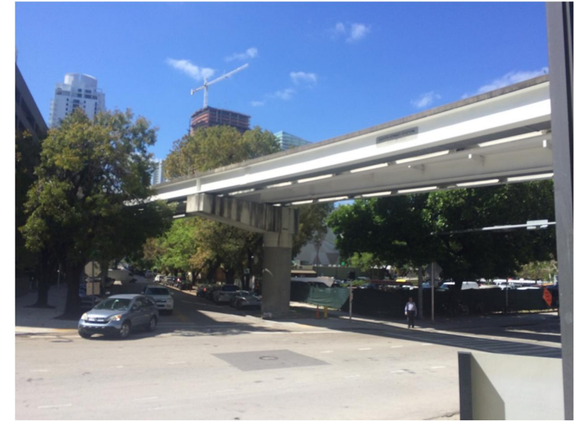
Photo 53: 8th Street Metromover Station
