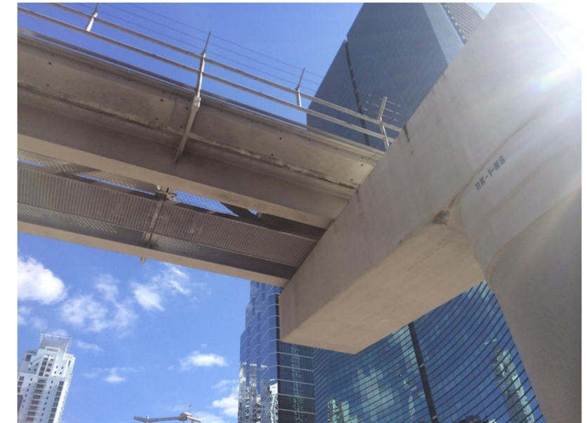
Photo 6: Financial District Metromover Station
