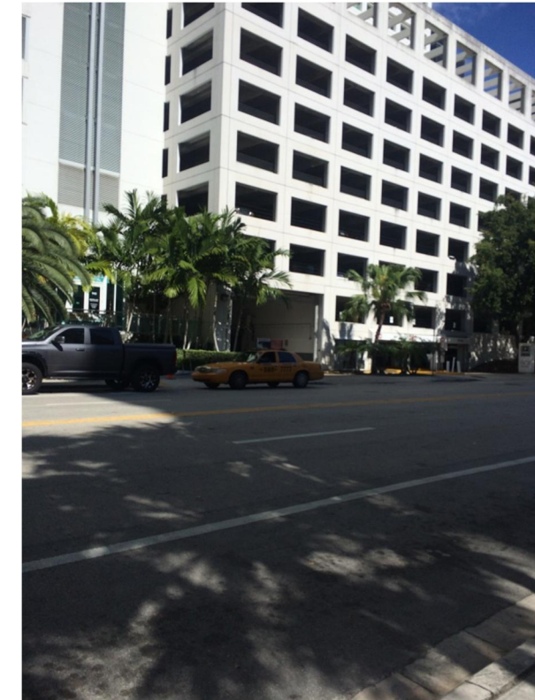
Photo 30: Brickell Bay Drive
