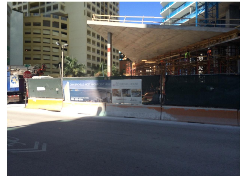
Photo 24: Brickell Bay Drive
