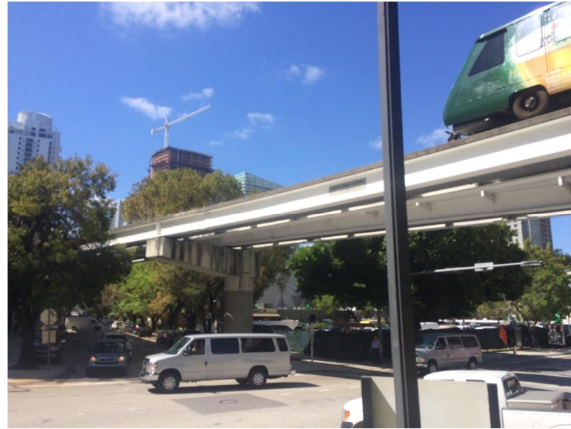
Photo 51: 8th Street Metromover Station
