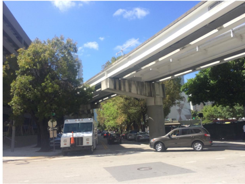
Photo 49: 8th Street Metromover Station
