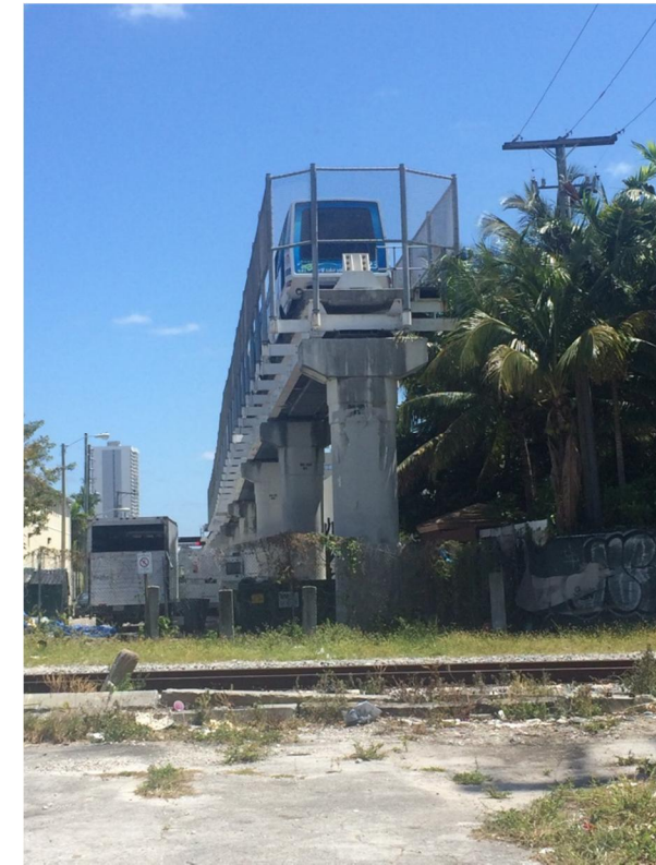
Photo 59: End of Line, School Board Metromover Station
