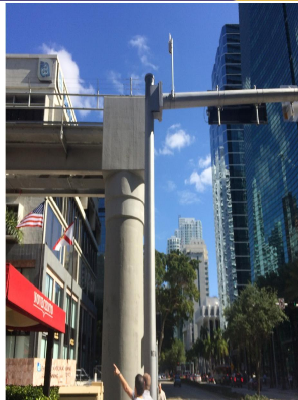
Photo 9: End of Line, Financial District Station
