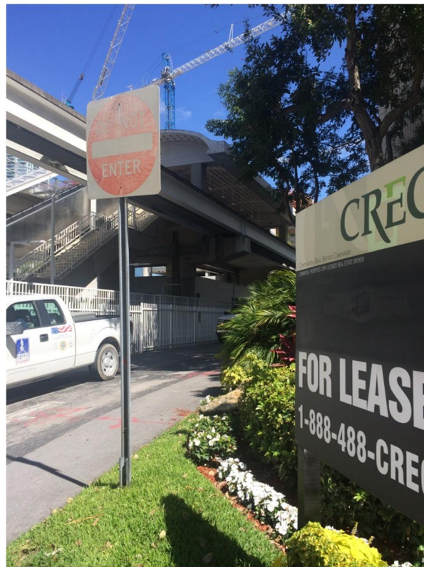
Photo 44: 8th Street Metromover Station
