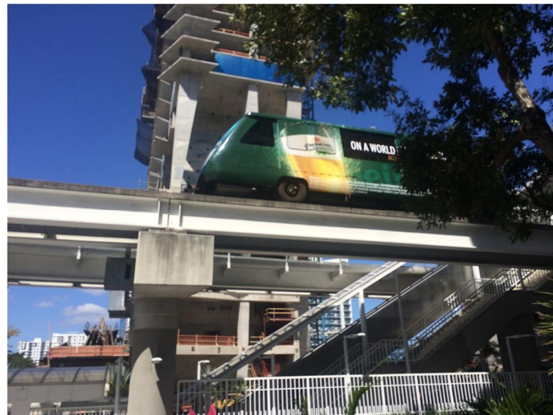
Photo 52: 8th Street Metromover Station
