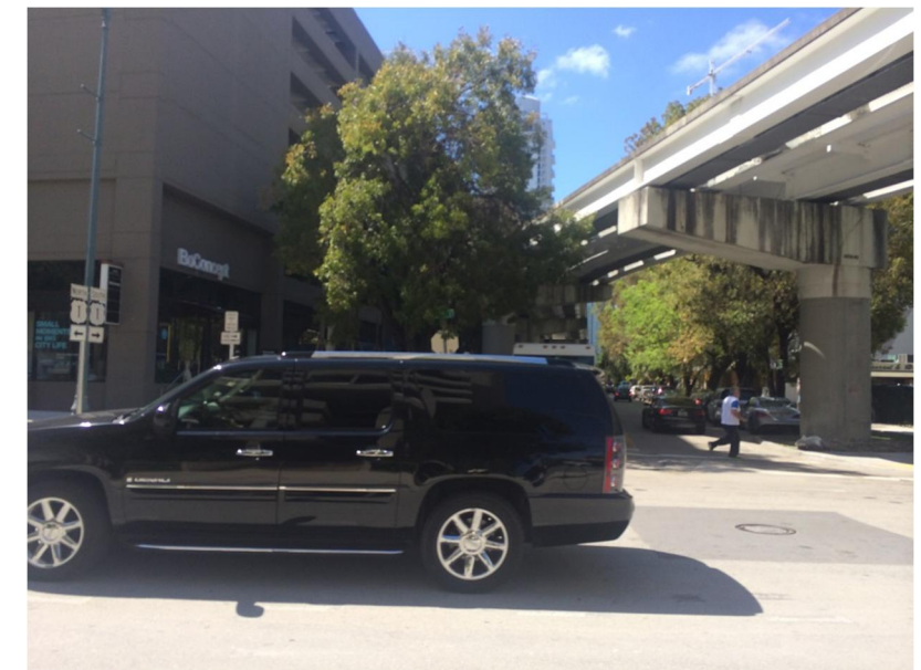
Photo 48: Guideway South of 8th Street Metromover Station
