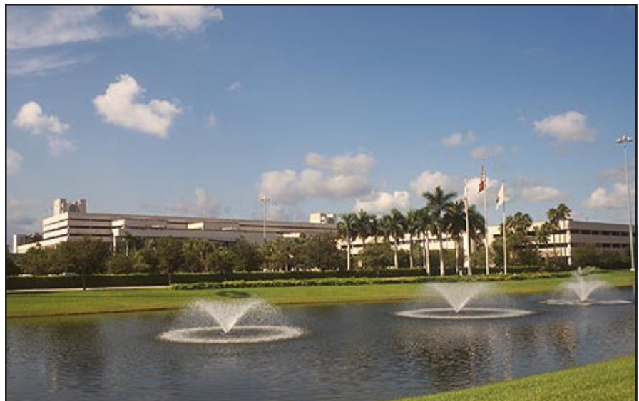
Source: Palm Beach International Airport
