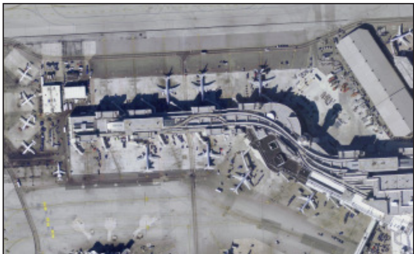
An aerial view of Miami International Airport
