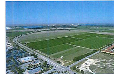
aerial view from southeast (se) corner
