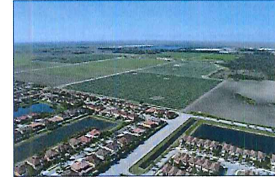
aerial view from northeast (ne) corner
