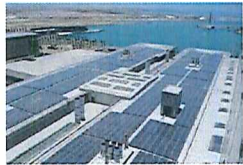
ROOF TOP SOLAR PANEL ARRAY
