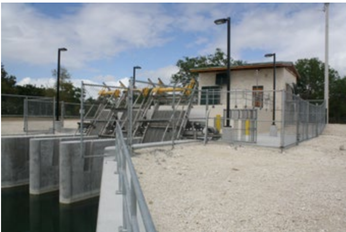
Structure S700 (Pump Station) of the Cutler Slough Rehydration Project April, 2012
