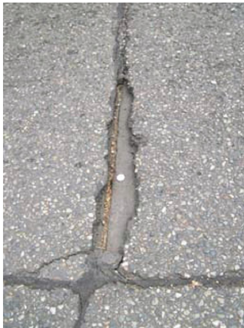
Seattle's Bicycle Spot Improvements fixes pavement problems
