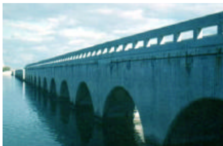
Long Key Bridge - Then and Now
