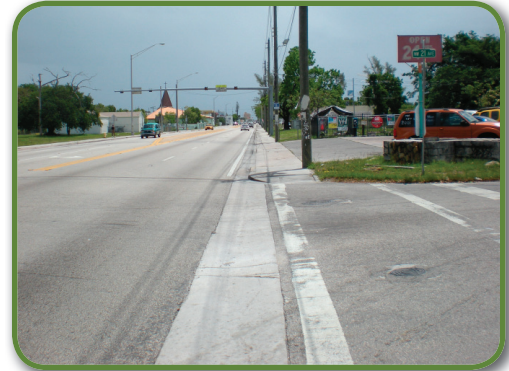
Crossing arterials such as NW 54th Street requires safety improvements
