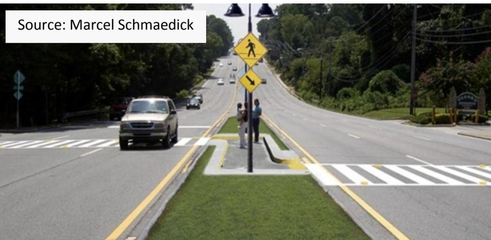
**Mid-Block Crossing with Staggered Median Crossing on 6-Lane Roadway**
