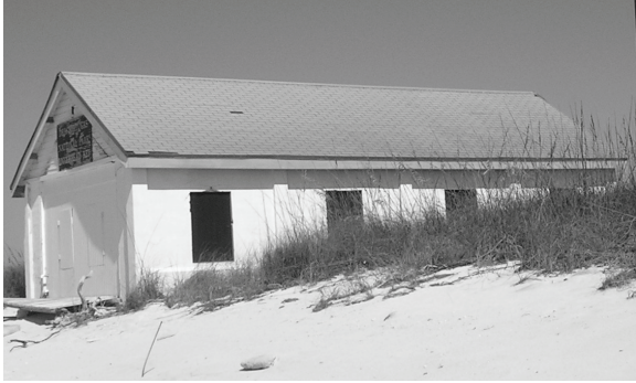
Figure 144. South elevation of Boat House.
