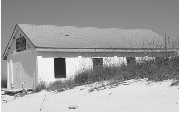
Figure 144. South elevation of Boat House.
