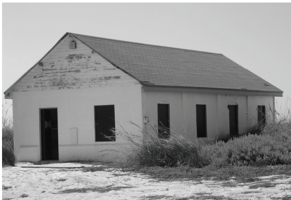
Figure 142. North elevation of Boat House.
