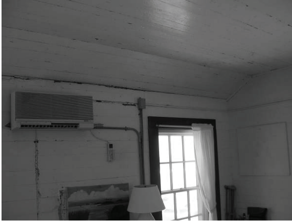
Figure 107. View of second floor facing south.
