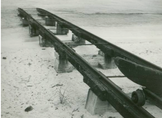
Figure 60. Ca. 1941 photo of marine railway extending into the Gulf of Mexico.
