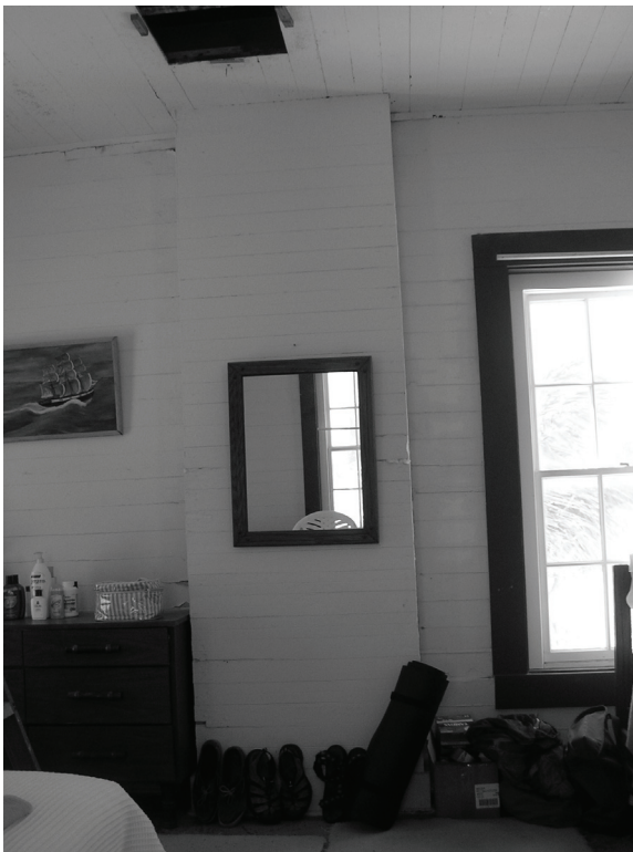
Figure 112. View of horizontal tongue and groove encasing chimney.
