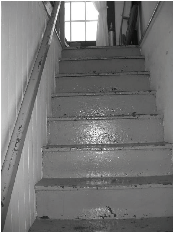
Figure 102. Wood stairs and railing in Kitchen Building.
