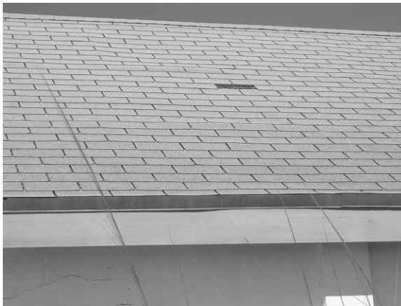
Figure 132. Metal flashing and eave fascia at north elevation.
