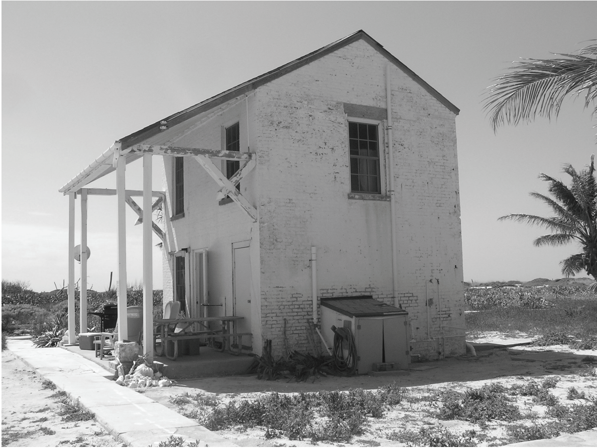
Figure 90. North elevation of Kitchen Building.
