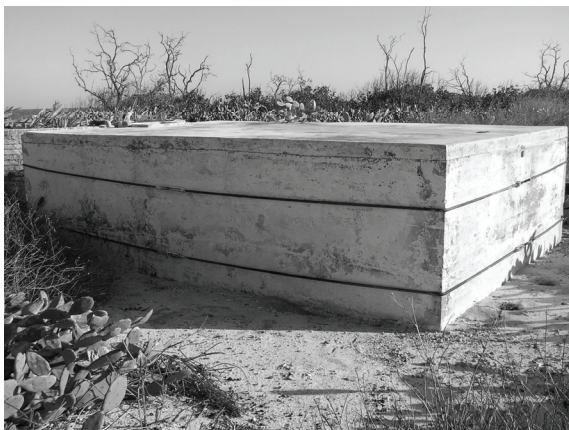
Figure 158. View of south concrete cistern.
