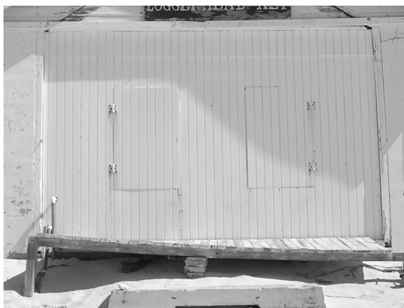
Figure 140. Wood deck at west elevation.
