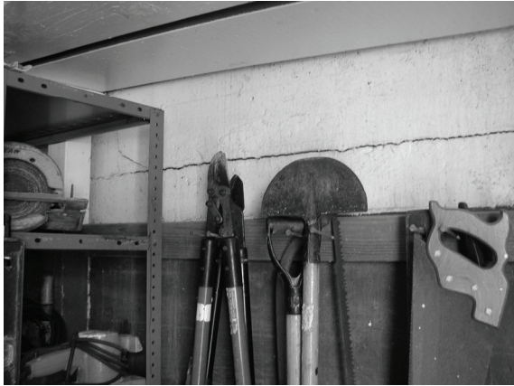
Figure 156. Interior view of the New Oil House walls and tool storage.
