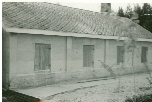
Figure 55. Ca. 1940s photo of side elevation of Boat House showing shuttered windows. openings.
