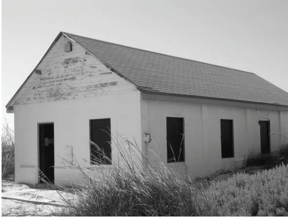
Figure 135. Concrete and framed walls of Boat House.
