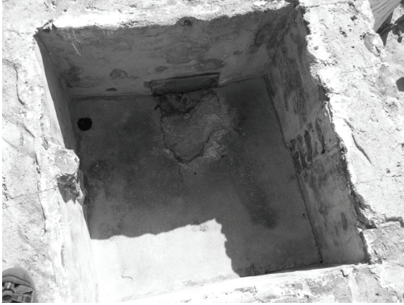
Figure 127. View of intake box at south brick cistern.
