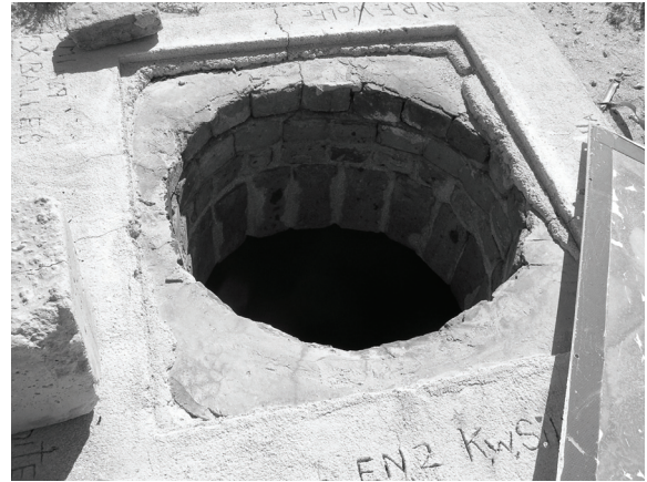
Figure 124. Opening in the brick extension of east brick.
