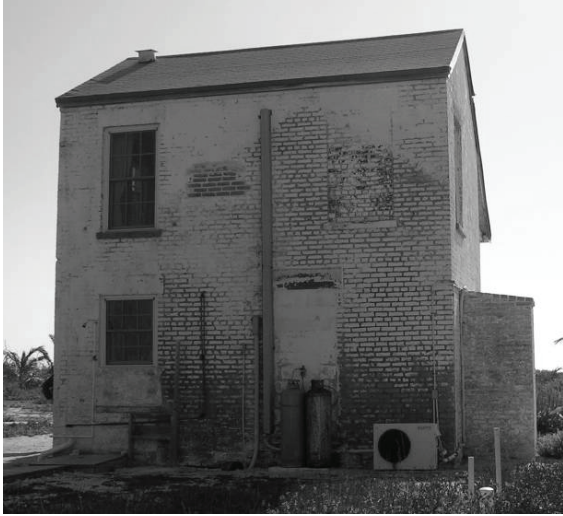
Figure 85. West (rear) elevation of Kitchen Building. Note the ghosting left by the Kitchen/Dining Room addition that was removed after the 1945 fire.
