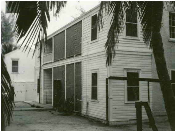
Figure 39. Ca. 1941 photo of enclosed rear porch at Keeper's Dwelling.
