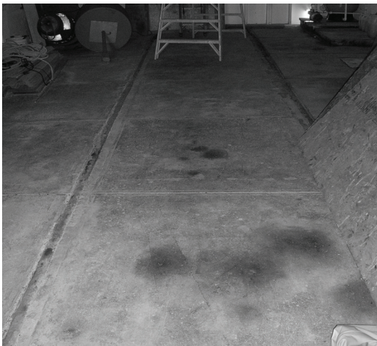
Figure 150. Concrete panel flooring inside Boat House.
