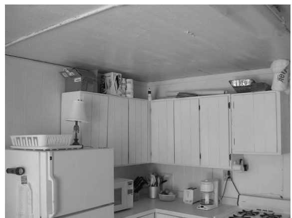
Figure 101. Interior view of first floor kitchen area facing west.
