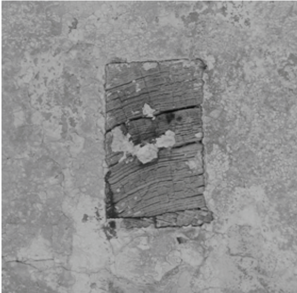
Figure 83. Blocking embedded in masonry walls, adjacent to various window openings.
