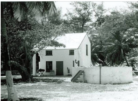
Figure 26. Undated view of brick cistern located adjacent to original Kitchen.
