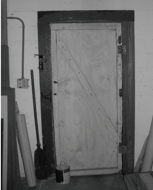
Figure 151. View of interior door face with flat wood casing.
