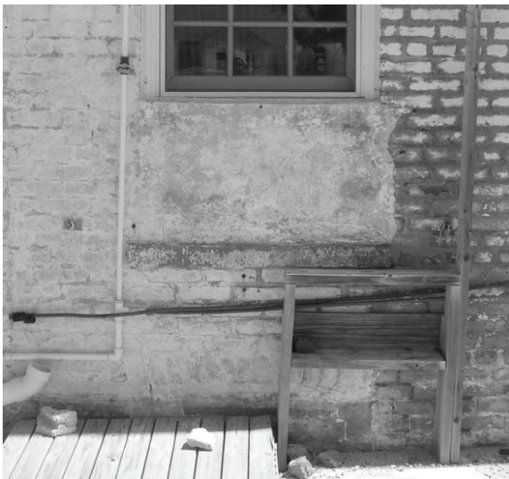
Figure 86. Outline of brick segmental arch at north side of west elevation.
