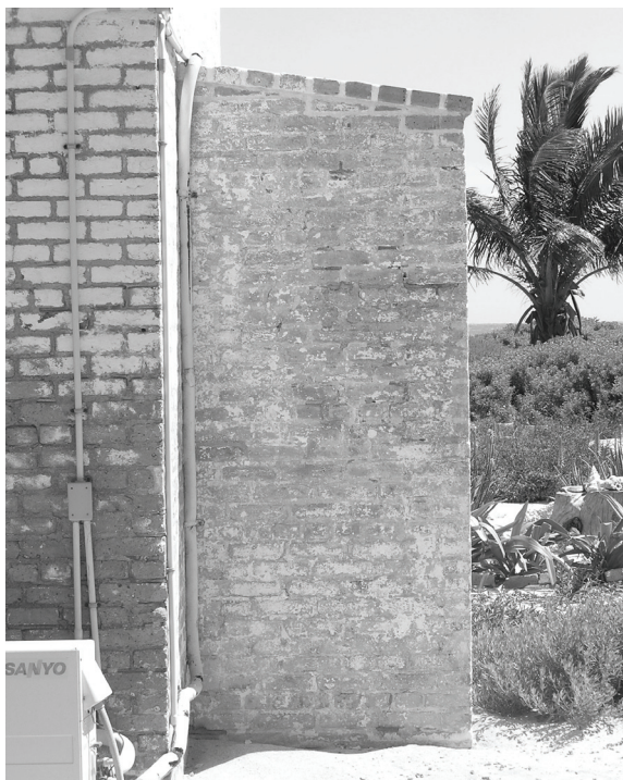
Figure 92. South elevation of Kitchen Building.
