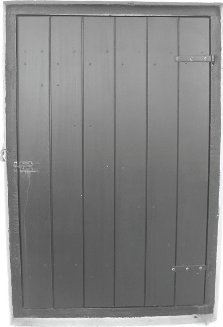
Figure 147. Example of typical wood shutters at window openings.
