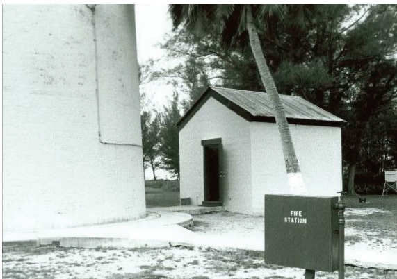
Figure 62. Undated oblique view of Oil Storage Building/Bosun's Workshop adjacent to Lighthouse.
