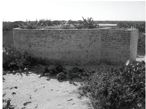
Figure 125. View of south brick cistern facing south.
