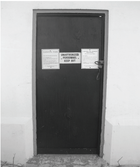
Figure 146. View of wood door at front entry.
