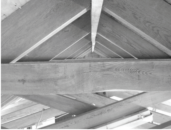
Figure 129. Roof framing at Boat House.
