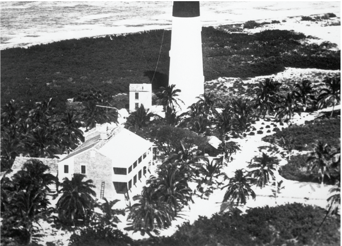
Figure 1. Undated early twentieth century view of the Dry Tortugas Light Station.
