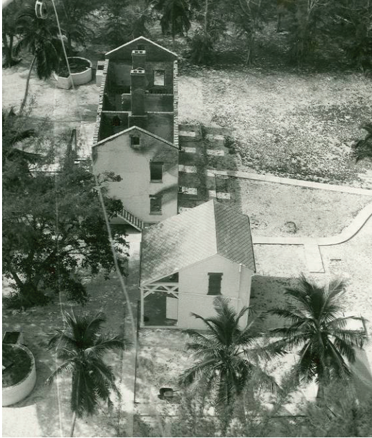
Figure 17. Image taken from the top of the tower showing the burned remains of the original keeper's dwelling.
