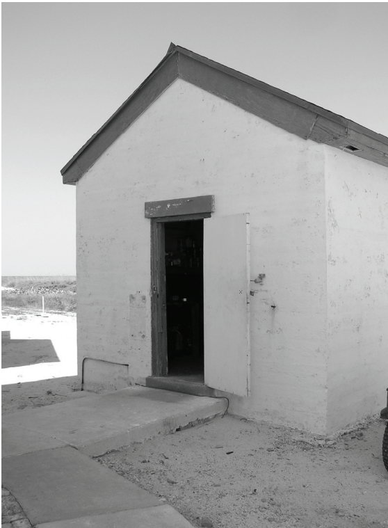
Figure 155. View of New Oil House façade and entry facing west.
