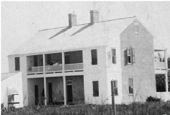
Figure 22. Close-up view of rear elevation of original Keeper's Dwelling.
