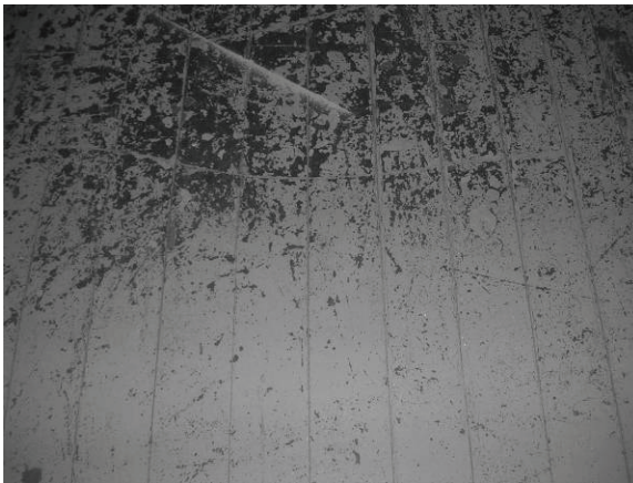
Figure 108. Close-up of tongue and groove flooring at second floor.
