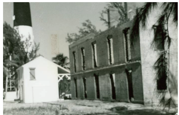
Figure 69. Undated oblique view of Keeper's Dwelling showing fire damage.
