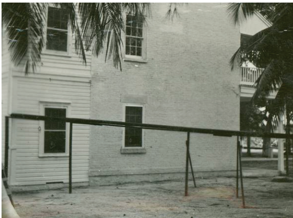
Figure 49. Ca. 1941 photo of gutters leading from Keeper's Dwelling downspouts to cisterns.
