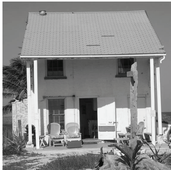
Figure 82. Two entrances & doors at east elevation.
