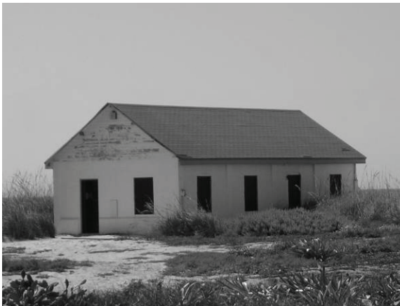
Figure 130. Gable roof of Boat House.
