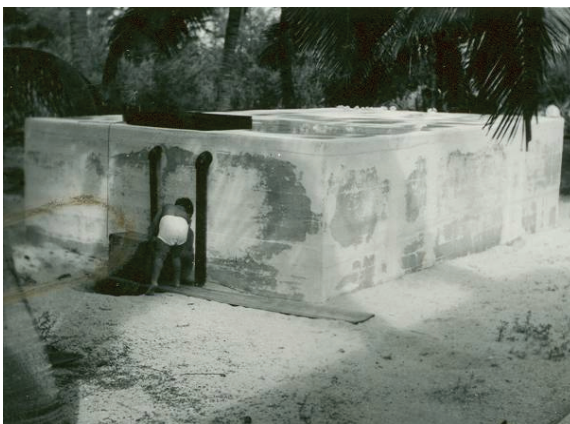
Figure 50. Ca. 1941 photo of concrete cistern adjacent to 1922 Keeper's Residence.
