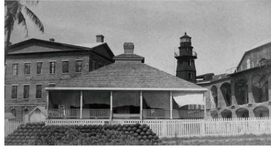
Figure 15. Undated view of the Garden Key Keeper's Residence with the iron lighthouse on bastion C in the distance.
