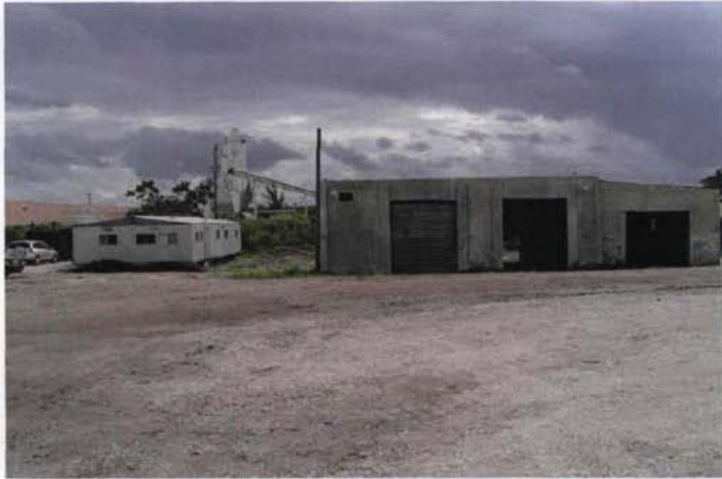
New temporary trailer/office and old garage on Payne parcel.
