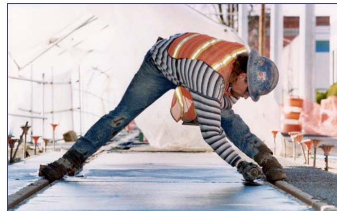
Portland Streetcar Rail Construction
