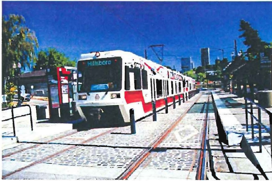
Portland at-grade guideway
