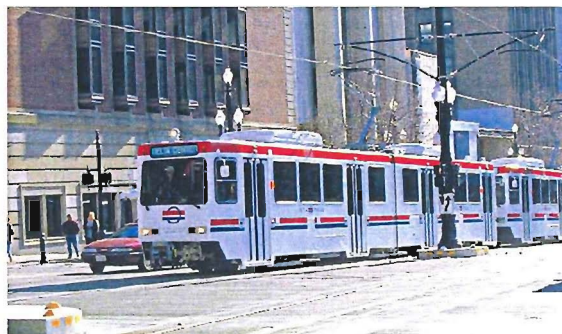
Overhead catenary system delivers electricity to power the Salt Lake City light rail transit line
