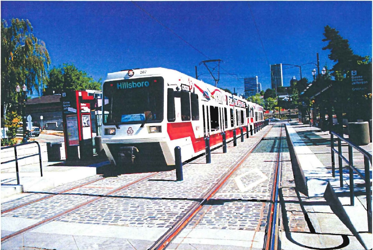
Light Rail Transit—Portland, Oregon
