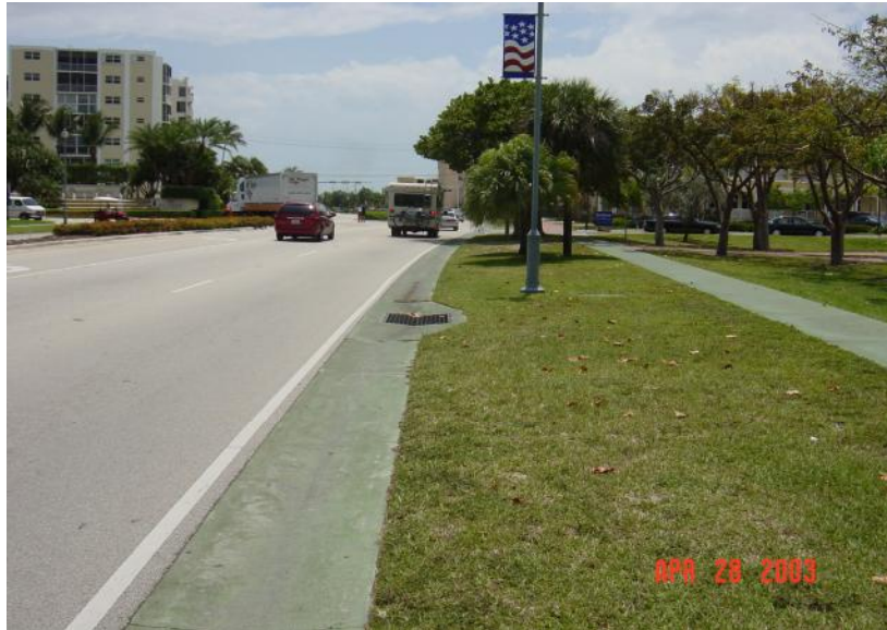
Existing Valley Gutter at Edge of Pavement
