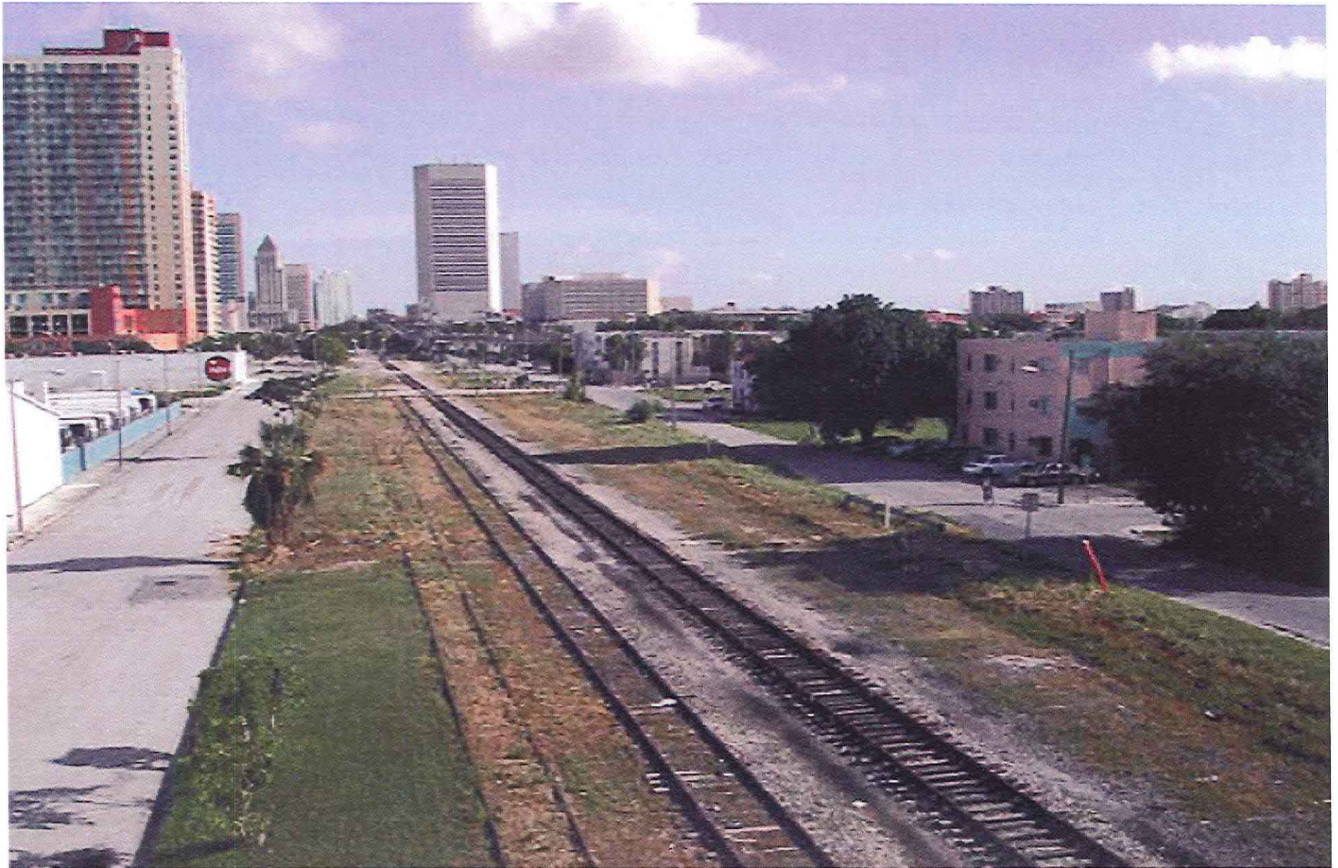
NW 1st Avenue, looking south: Existing conditions. The railroad tracks are especially divisive because few east-west streets cross them. The lack of shade, empty lots, and blank walls contribute to a hostile environment.
