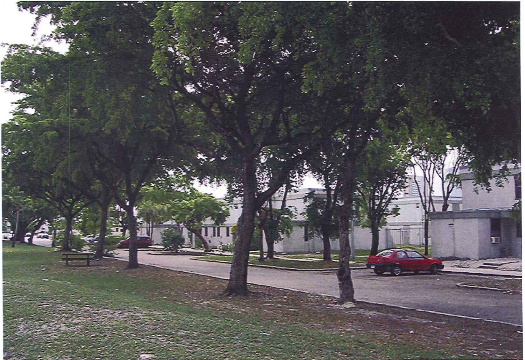
Reeves Park, existing conditions: Apartment buildings are set back far from the street. There are few windows and doors facing the park, depriving it of natural surveillance.
