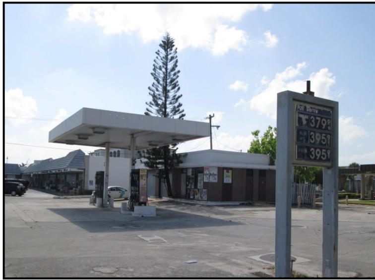
Out of Service Gas Station (2014)
