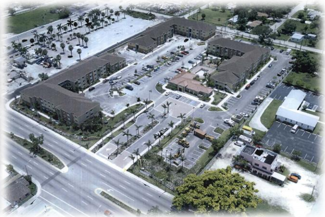
The Corinthian completed (June 8, 2007)
