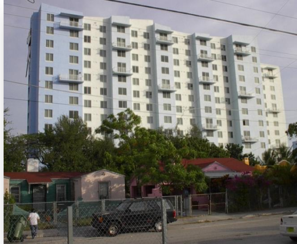
Completed Los Sueños Apartments
