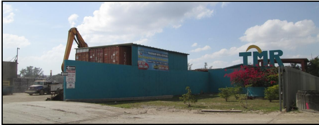
Trademark Metals Recycling Facility (2014)
