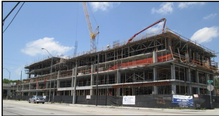
Site construction (May 2014)
