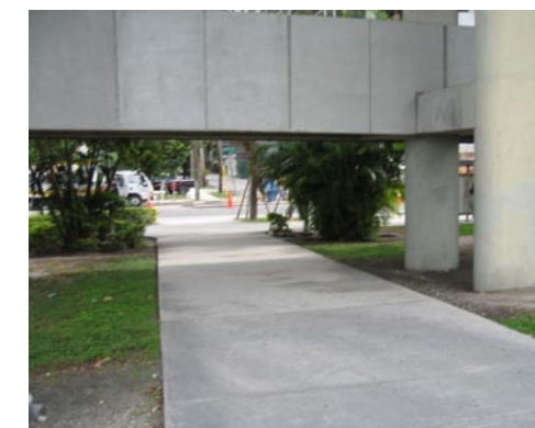
In areas where low clearance obstacles cannot be adjusted to meet the eight-foot height requirement, signage shall be used to warn trail users that they are approaching a low clearance area.
