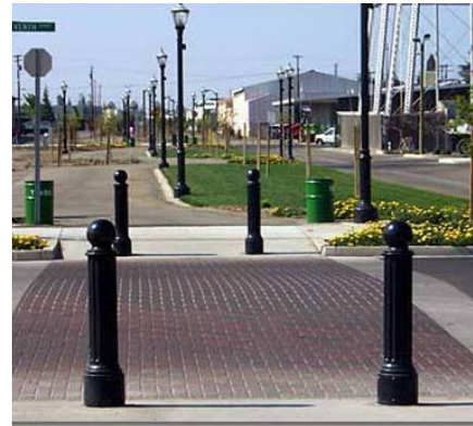
Removable bollards such as these may be used to prevent unauthorized access along the trail.
