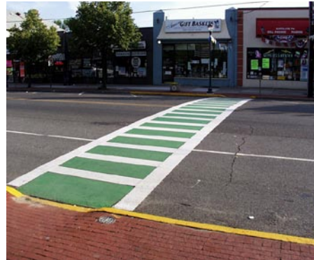
Additional pavement coloring, as shown in this picture, should be utilized to emphasize M-Path crossings.
