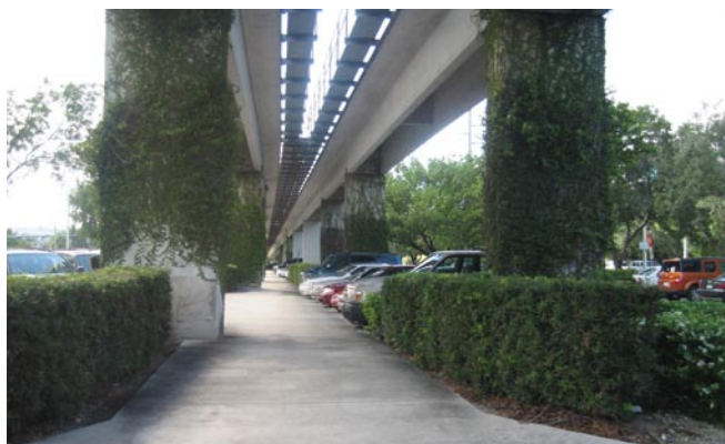
Installing wheel-stops in the spaces adjacent to this section of M-Path will minimize encroachment of the trail.
