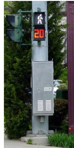
Pedestrian signal heads should feature countdown timers whenever possible.
