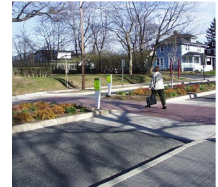
The mid-block crossing shown in this picture features a raised colored crosswalk along with a pedestrian refuge island.
