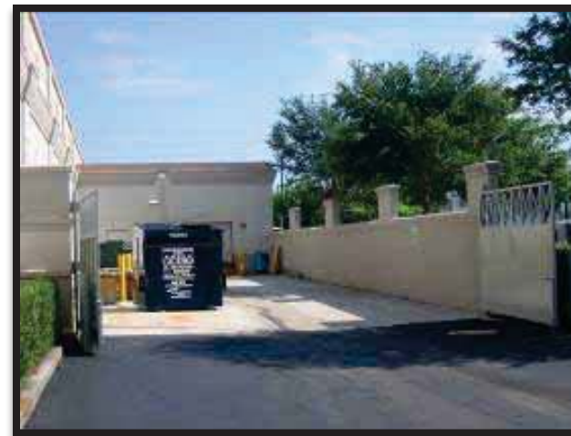
Walled in service entrance and hidden refuse containers
