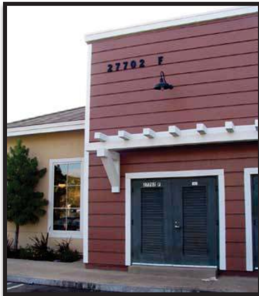
Screened service entrance
